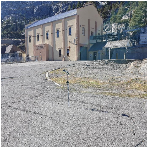
Northeast of Tailrace
