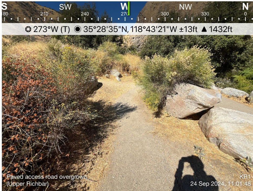
Photo B-36. Upper Richbar Day Use Site – Paved Access Path
