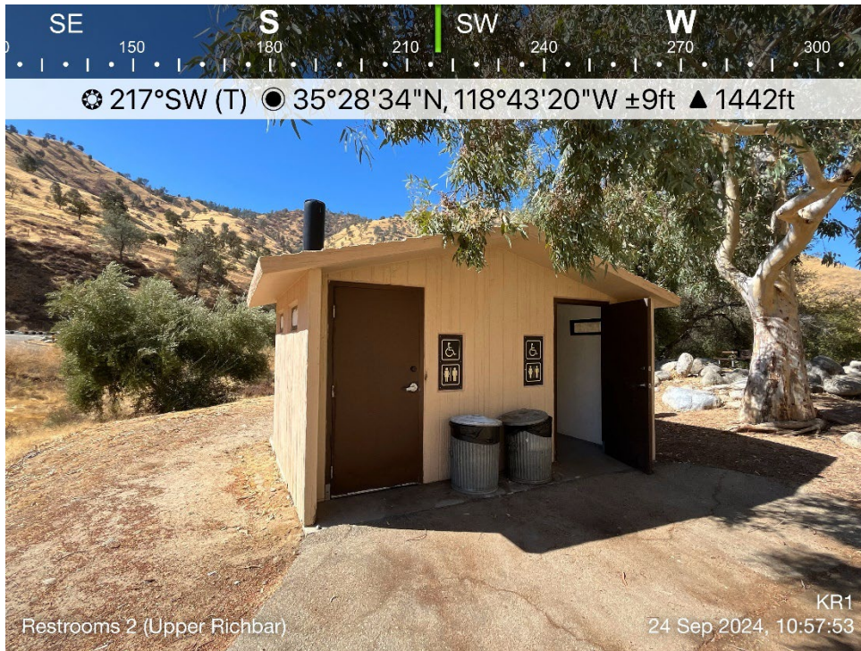
Photo B-32. Upper Richbar Day Use Site – Pit Toilets #2
