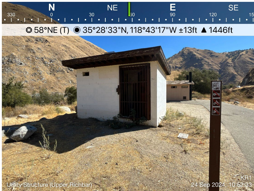
Photo B-29. Upper Richbar Day Use Site – Locked Utility Structure
