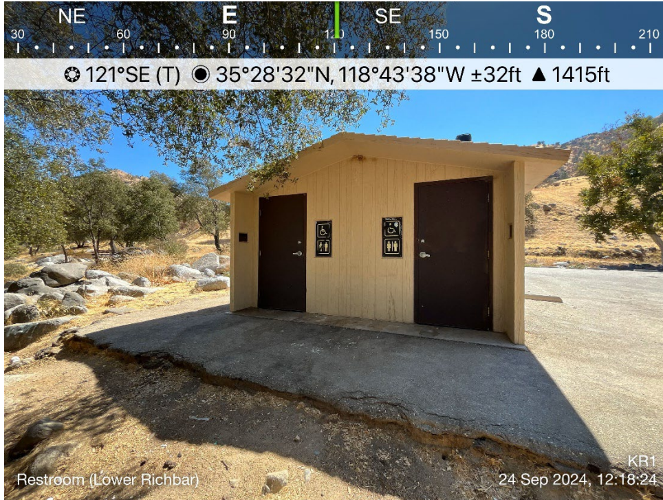
Photo B-59. Lower Richbar Day Use Site – Pit Toilets
