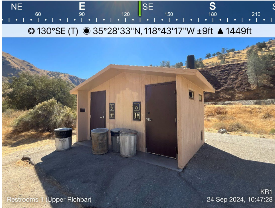
Photo B-30. Upper Richbar Day Use Site – Pit Toilets #1
