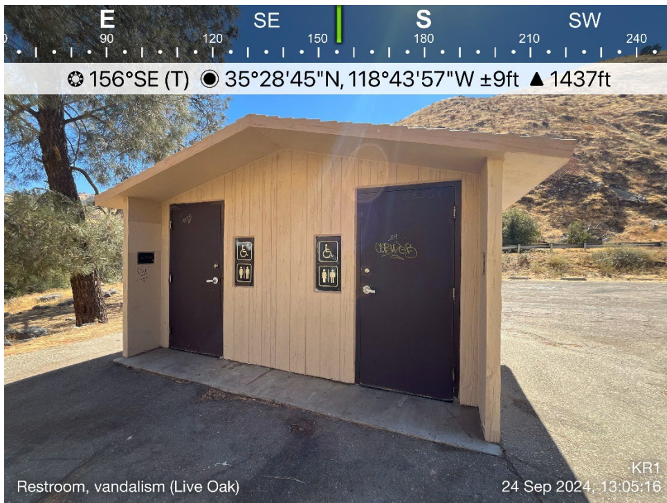
Photo B-70. Live Oak Day Use Site – Pit Toilets
