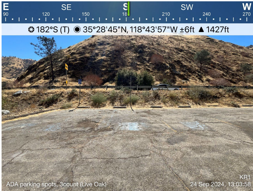
Photo B-68. Live Oak Day Use Site – ADA Parking Spots
