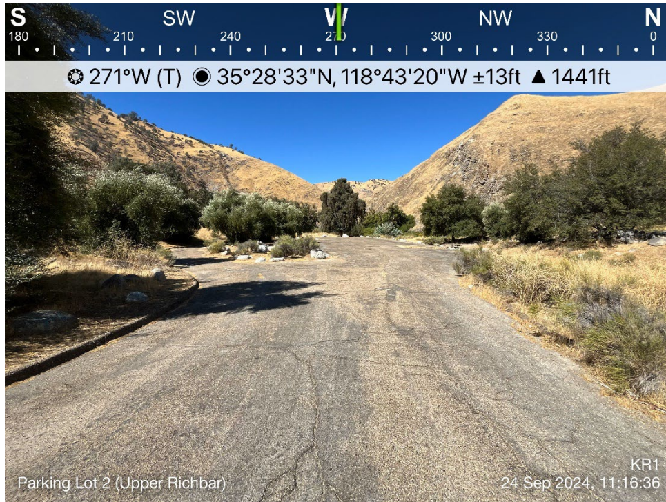
Photo B-26. Upper Richbar Day Use Site – West Parking Lot
