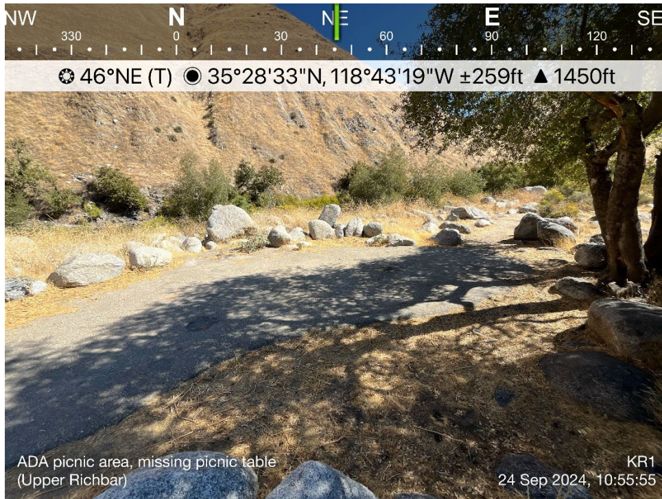
Photo B-34. Upper Richbar Day Use Site – Paved Access Path
