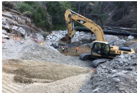
Installation and Compaction of Permeable Base Rock
