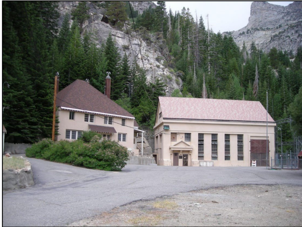
Figure 6.12-7. Poole Powerhouse (right) and Triplex Cottage (left).
