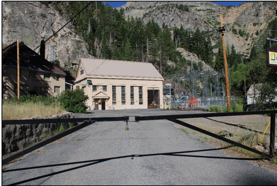
Figure 6.12-20. Key Observation Point 7—Poole Powerhouse Gate, View West.
