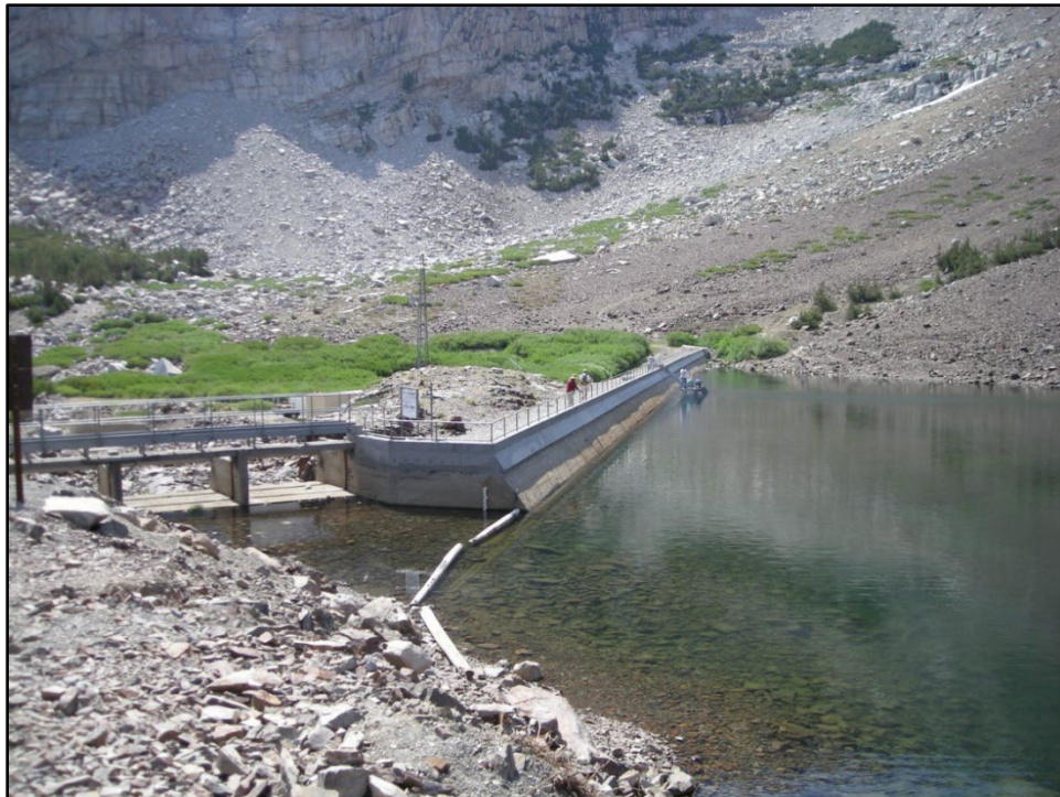
Figure 6.12-6. Rhinedollar Dam (Ellery Lake) and Spillway.
