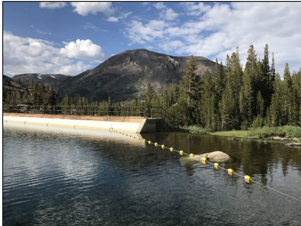
Figure 6.12-4. Tioga Dam and Spillway.
