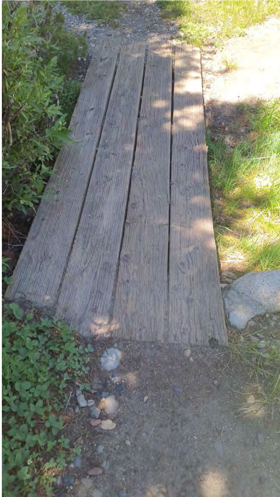
Photo 64. Junction Campground, Footbridge
