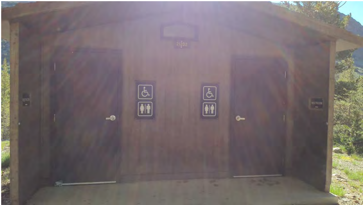
Photo 7. Saddlebag Lake Campground, Restroom
