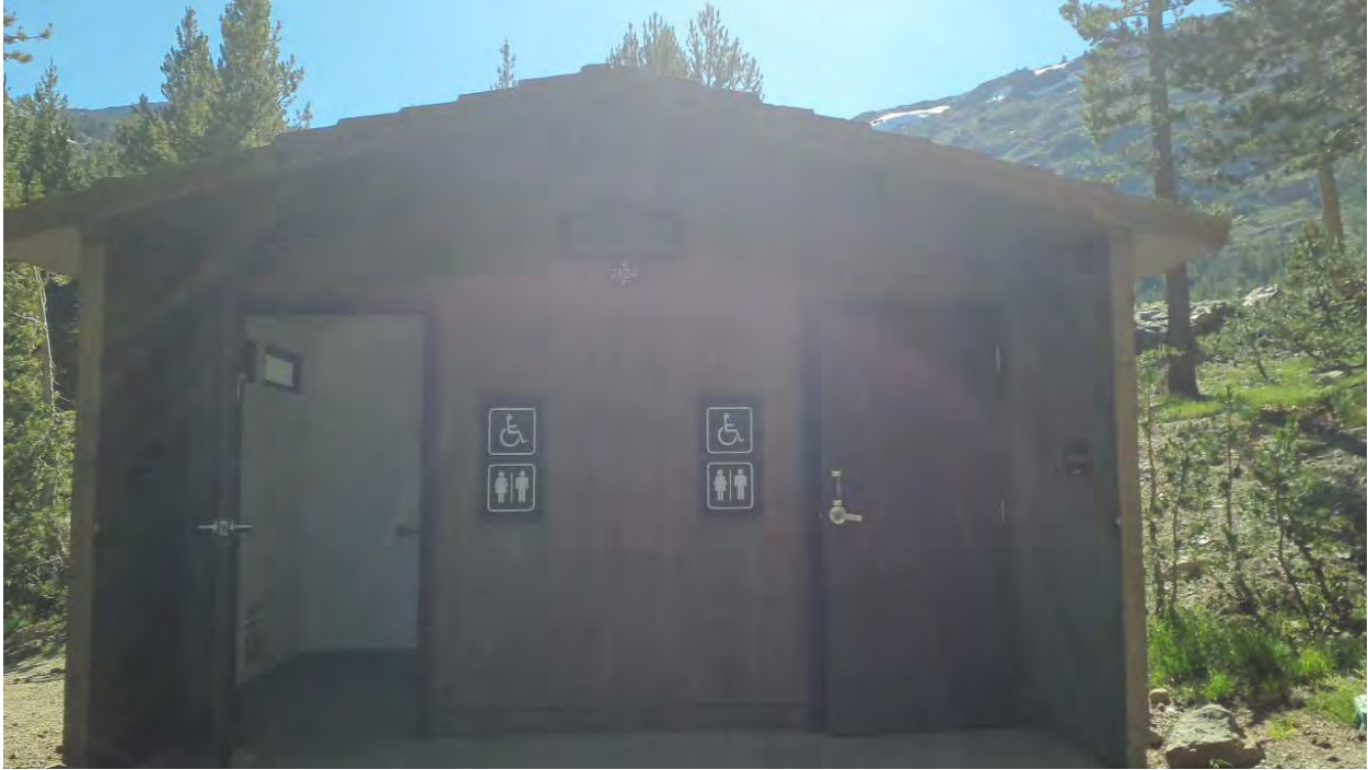
Photo 34. Tioga Lake Campground, Restroom
