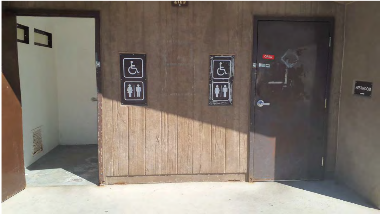
Photo 39. Tioga Lake Overlook, Restroom
