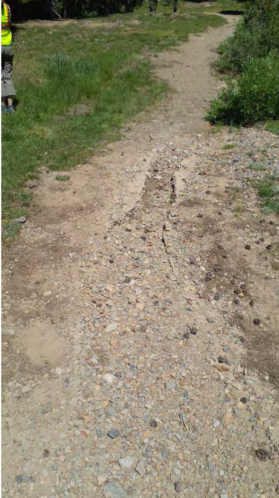
Photo 74. Sawmill Walk-In Campground, Erosion
