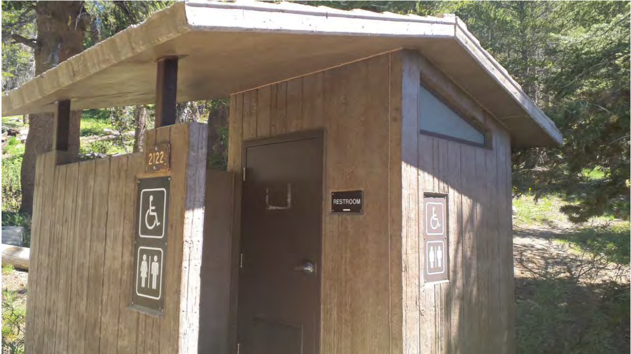
Photo 72. Sawmill Walk-In Campground, Restroom
