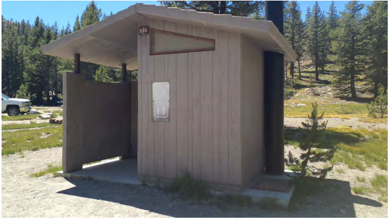
Photo 58. Junction Campground, Restroom
