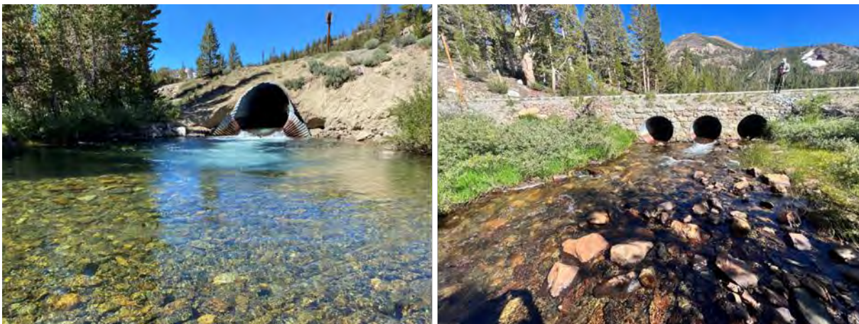
Figure 4.3-2. Potential Fish Passage Barriers Identified in Lee Vining Creek Between Ellery Lake and the Confluence of Slate Creek (left), and Glacier Creek Between the Confluence of Lee Vining Creek and Tioga Dam (right).
