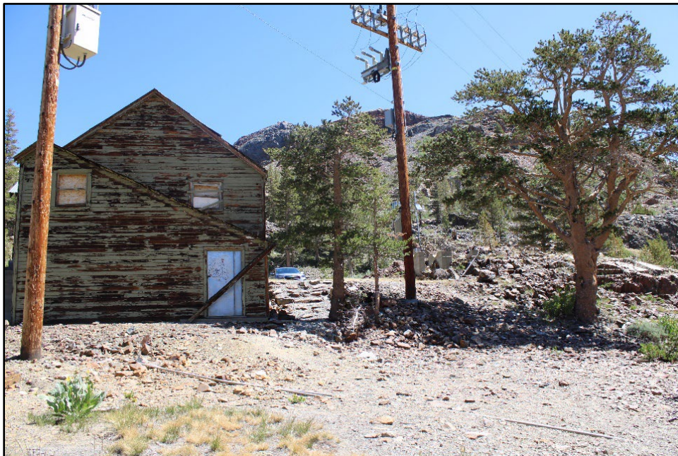
Figure 6.12-21. Key Observation Point 8—Pull-Off North of Ellery Lake, View Northeast with Operator’s Cabin.
