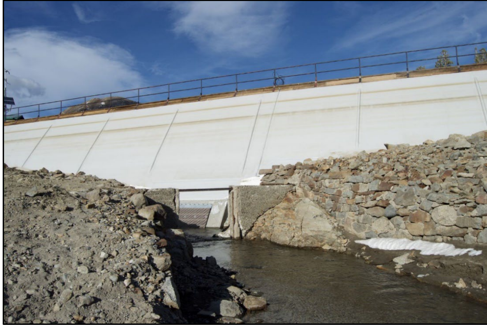
Figure 6.12-5. Tioga Dam Outlet.
