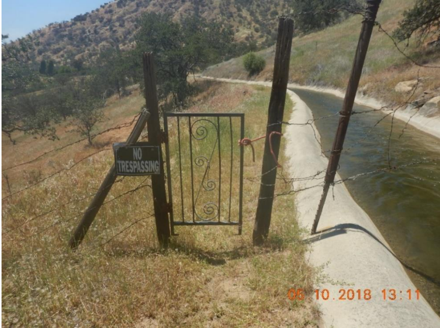
Photo C-1. Non-Project fencing with gate along the Kaweah No. Flowline. Photo taken May 10, 2018.
