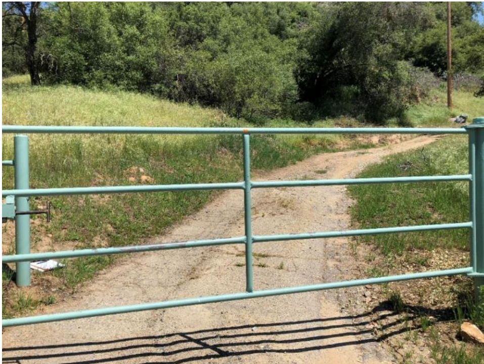
Photo D-12. Kaweah No. 2 Flowline West Access Road, gate, good condition, April 24, 2018
