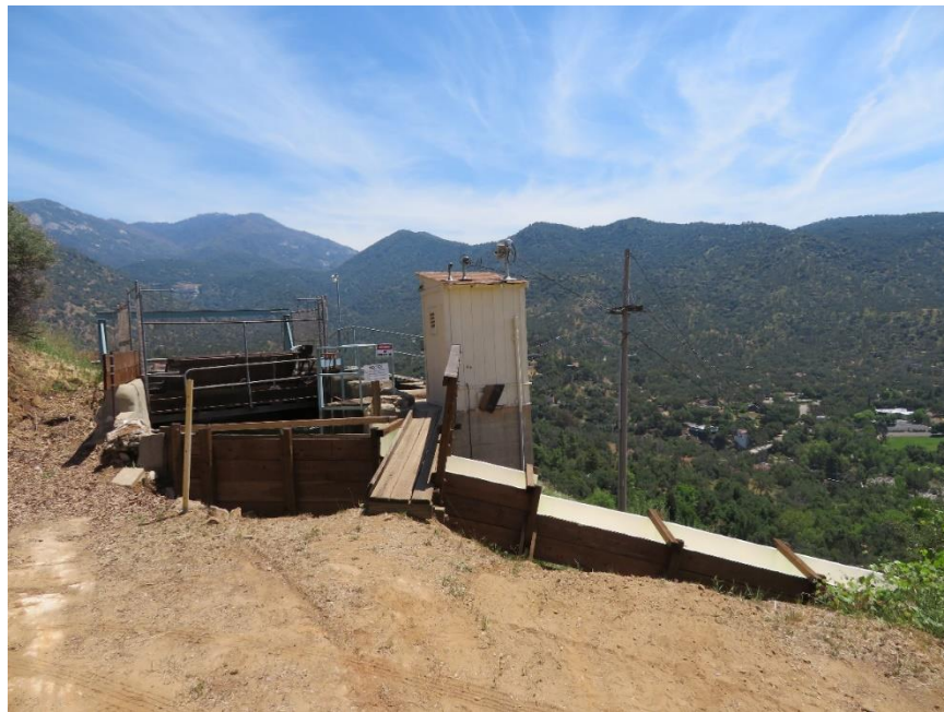
Photo B-12. Kaweah No. 2 Forebay Fence. Photo taken May 8, 2018.
