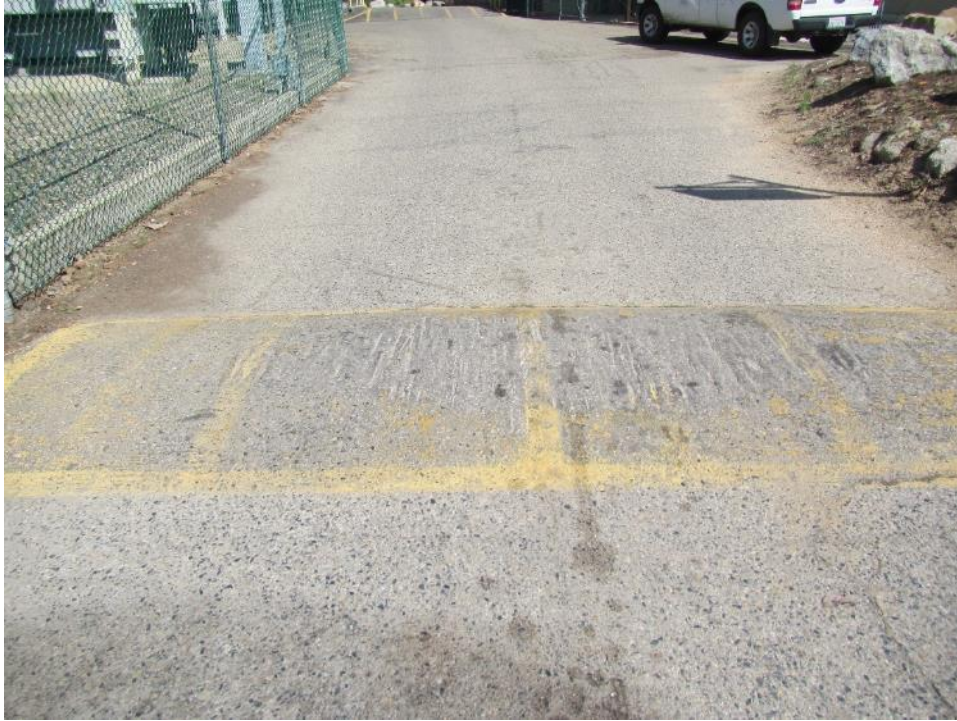
Photo D-11. Kaweah No. 2 Powerhouse Road, speed bump, good condition, April 24, 2018
