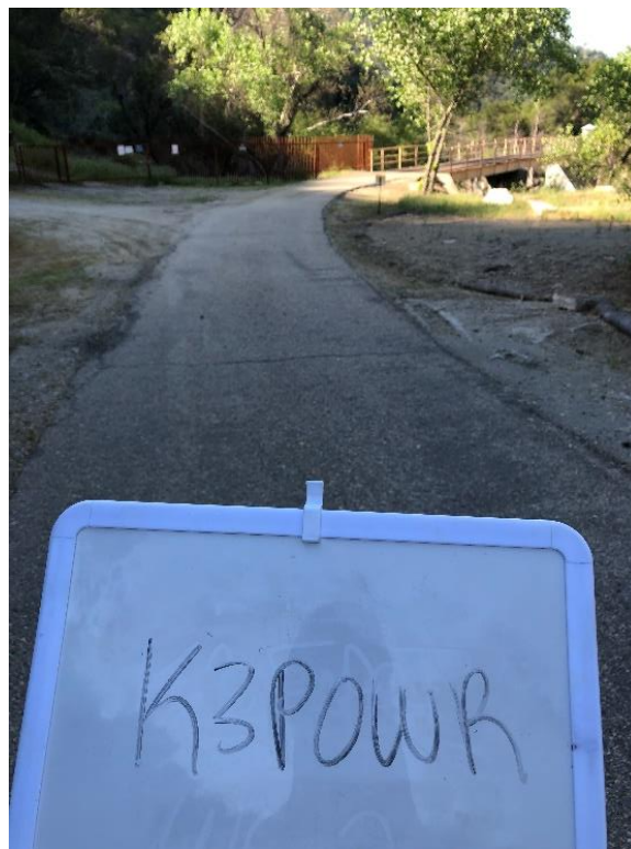
Photo D-2. Kaweah No. 3 Powerhouse Road, road end, good condition, April 24, 2018
