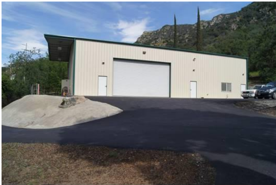
Photo B-2. New maintenance building constructed within the Kaweah No. 1 Powerhouse Campus boundaries in 2012. View is looking east from within the campus. Photo taken April 18, 2018.
