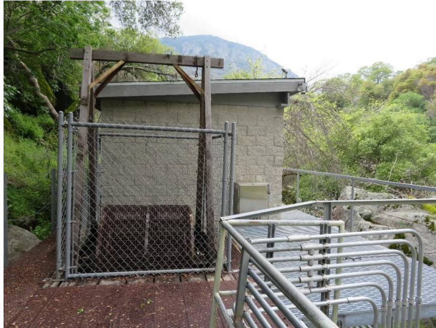
Photo B-7. Kaweah No. 1 Fish Wheel Fence. Photo taken April 17, 2018.
