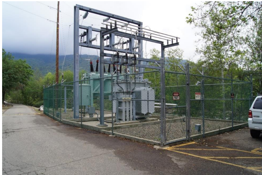
Photo B-14. Kaweah No. 2 Switchyard Perimeter Fence. Photo taken April 17, 2018.
