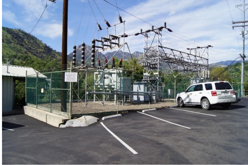
Photo B-9. Kaweah No. 1 Switchyard Perimeter Fence. Photo taken April 17, 2018.
