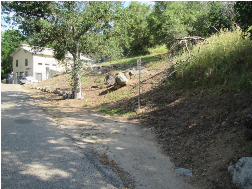
Photo D-10. Kaweah No. 2 Powerhouse Road, turnout, good condition, April 24, 2018
