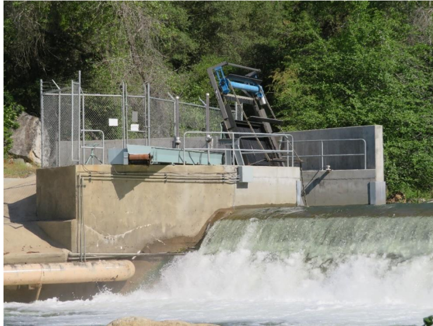
Photo B-11. Kaweah No. 2 Intake Fence. Photo taken April 17, 2018.
