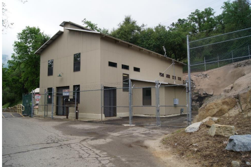
Photo B-13. Kaweah No. 2 Powerhouse Perimeter Fence. Photo taken April 17, 2018.
