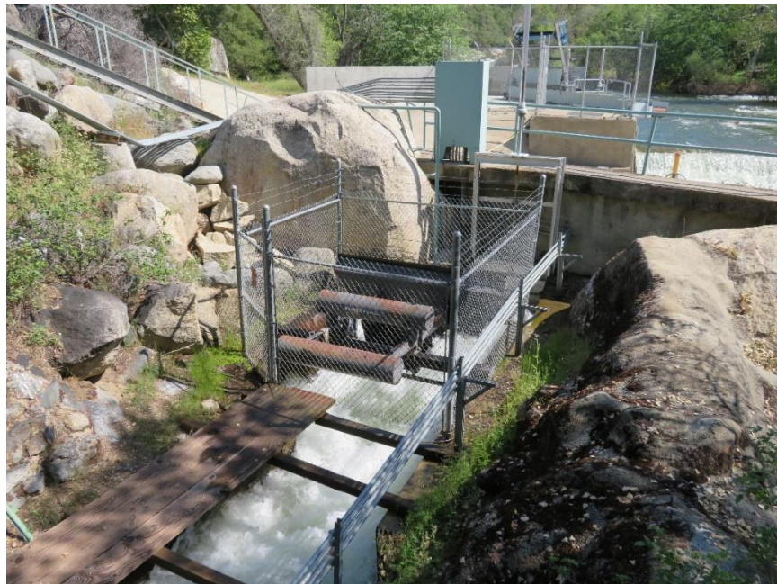
Photo B-16. Kaweah No. 2 Flowline Control Gate Fence. Photo taken April 17, 2018.
