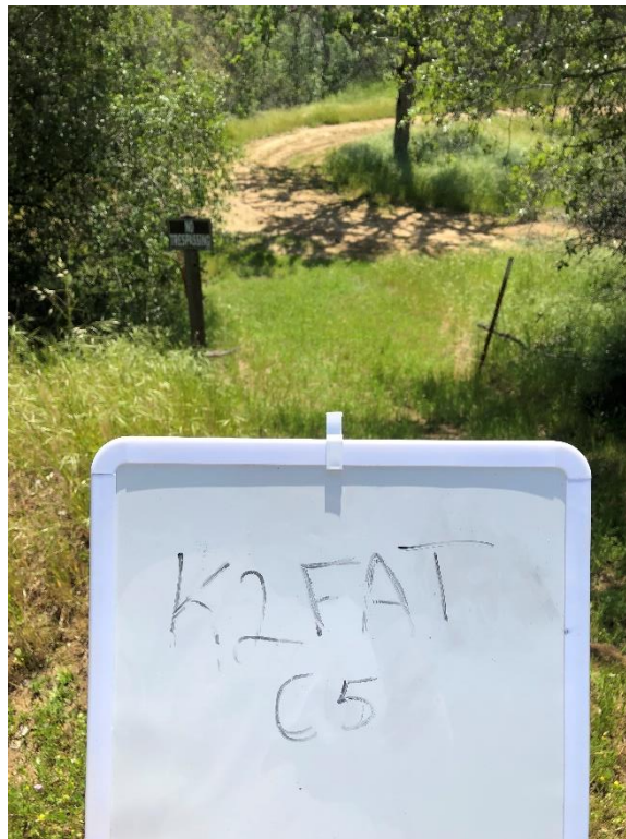
Photo D-4. Kaweah No. 2 Flowline Access Trail – Canal 5, trail end, good condition, April 25, 2018
