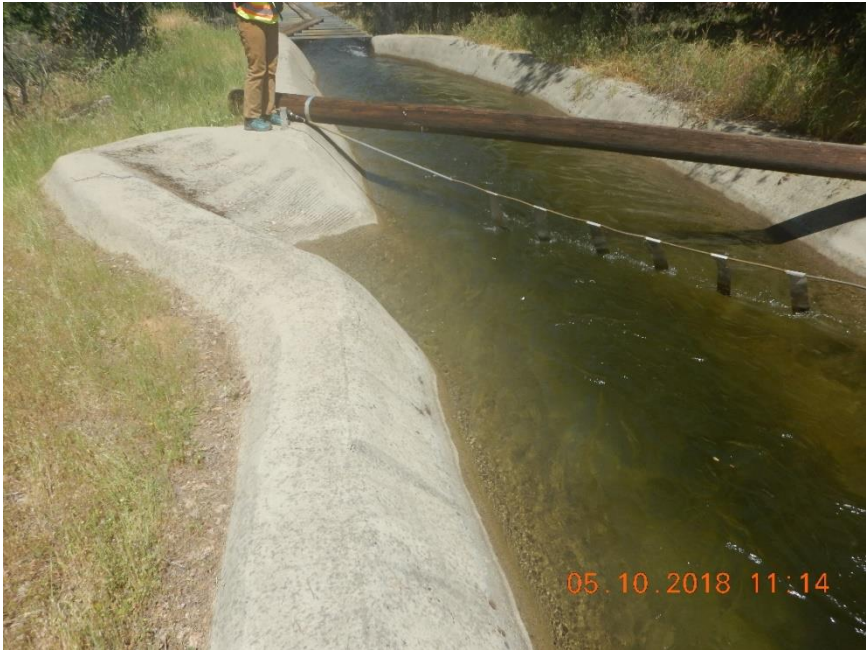
Photo B-2. Kaweah No. 2 Flowline, escape ramp, hazer, and flasher, all in good condition. Photo taken on May 10, 2018.
