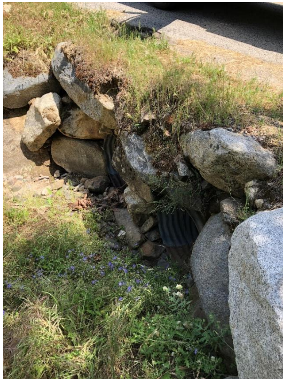
Photo D-6. Kaweah No. 2 Flowline East Access Road, culvert, good condition, April 25, 2018
