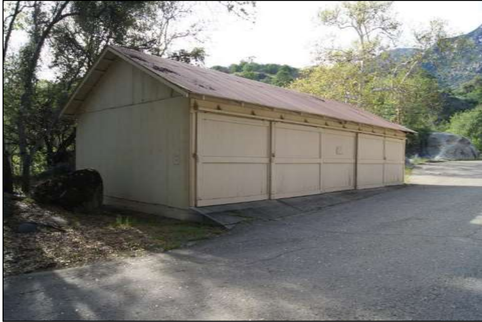
Photograph 9. Garage southwest of Kaweah No. 3 Powerhouse, camera facing northwest. April 18, 2018.
