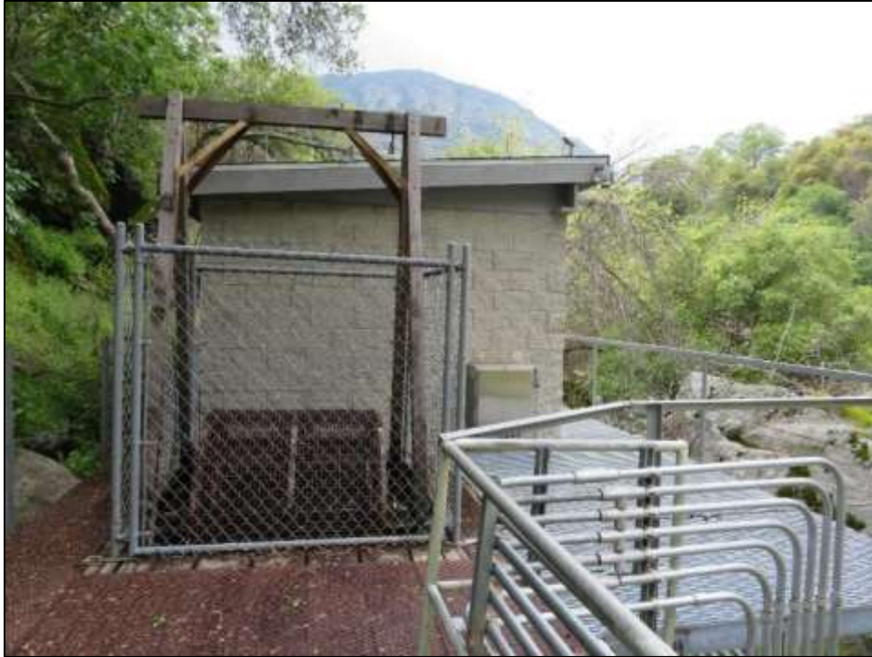
Photograph 8. Fish wheel and gauge house, camera facing southwest. April 18, 2018.
