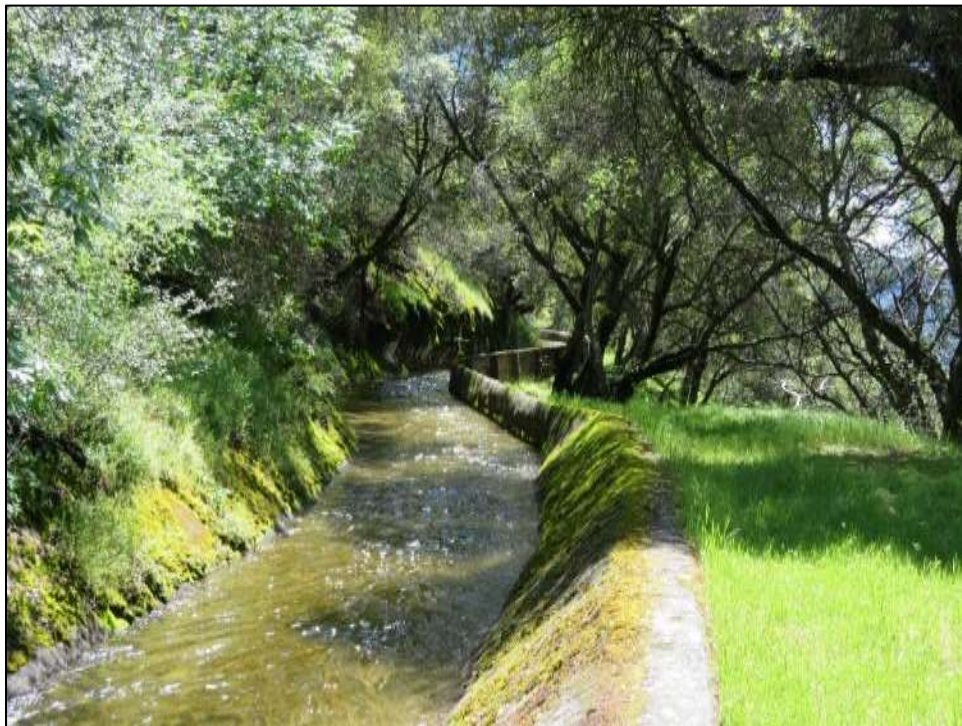
Photograph 3. Marble Fork Flowline showing ditch section transitioning to flume, camera facing south. April 17, 2018.
