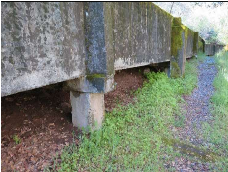
Photograph 5. Footing on Middle Fork Flowline flume, note replacement footing, camera facing west. April 17, 2018.
