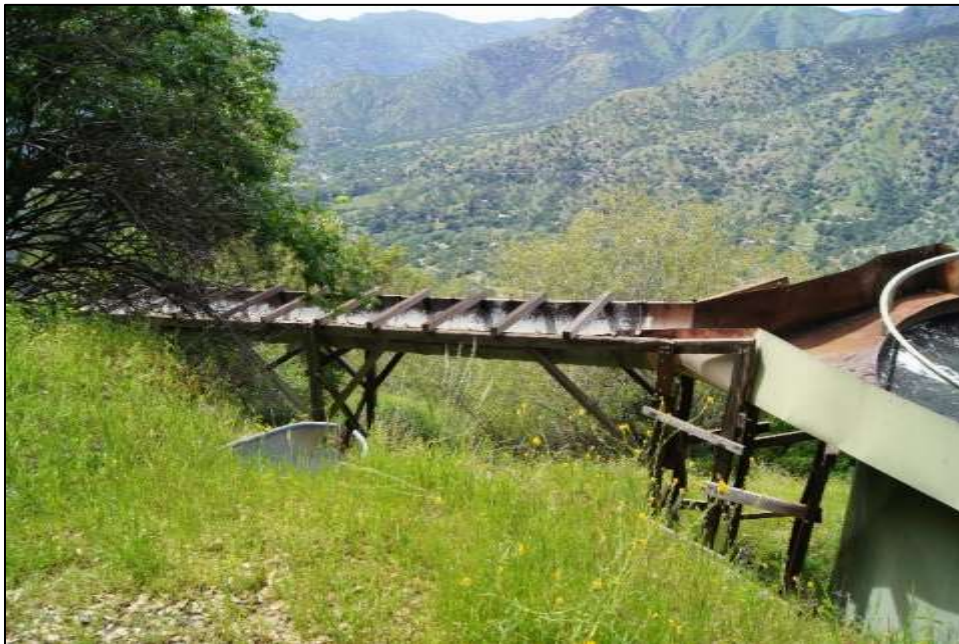
Photograph 4. Spillway chute, camera facing west. April 18, 2018.
