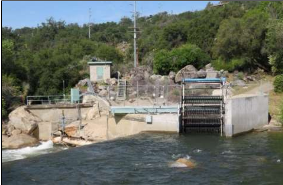
Photograph 2. Kaweah No. 2 Diversion intake structure, note metal trash rack, camera facing east. April 18, 2018.
