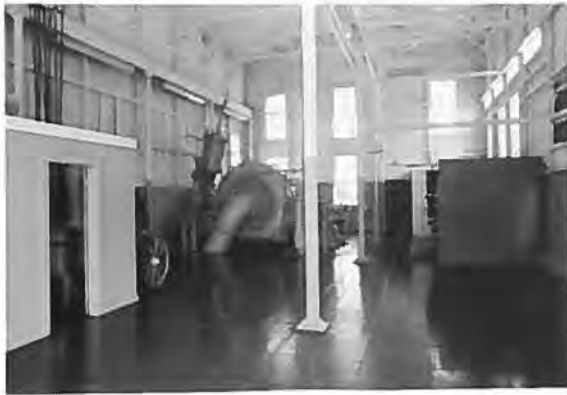
Bldg. 0101, Interior Kaweah Powerhouse No. 2 View to NE Roll 1, Frame 24, 6-27-89
