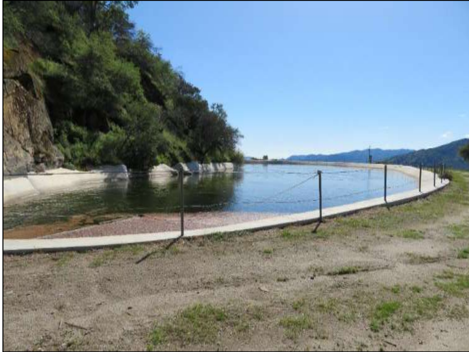
Photograph 2. Kaweah No. 3 Forebay, camera facing west. April 17, 2018.
