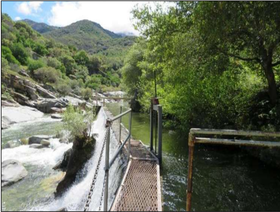
Photograph 4. Sandbox, note ungated spillway and two slide gates, camera facing east. April 17, 2018.
