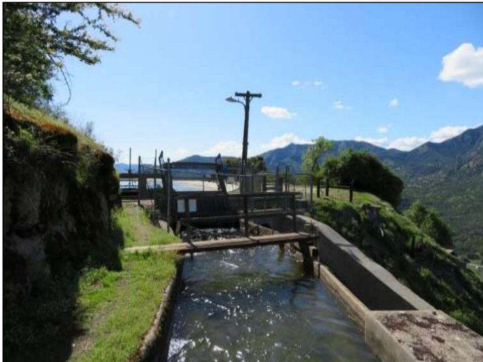
Photograph 3. Connection of Middle Fork Conduit with Kaweah No. 3 Forebay, camera facing west. April 17, 2018.
