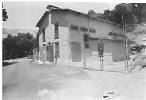
Bldg. 0101 Kaweah Powerhouse No. 2 View to N Roll 1, Frame 30, 6-27-89
