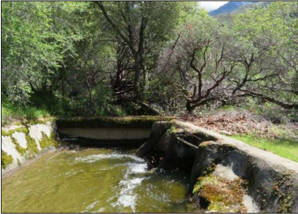
Photograph 6. End of Marble Fork Conduit and headgate for Marble Fork Siphon, camera facing east. April 17, 2018.
