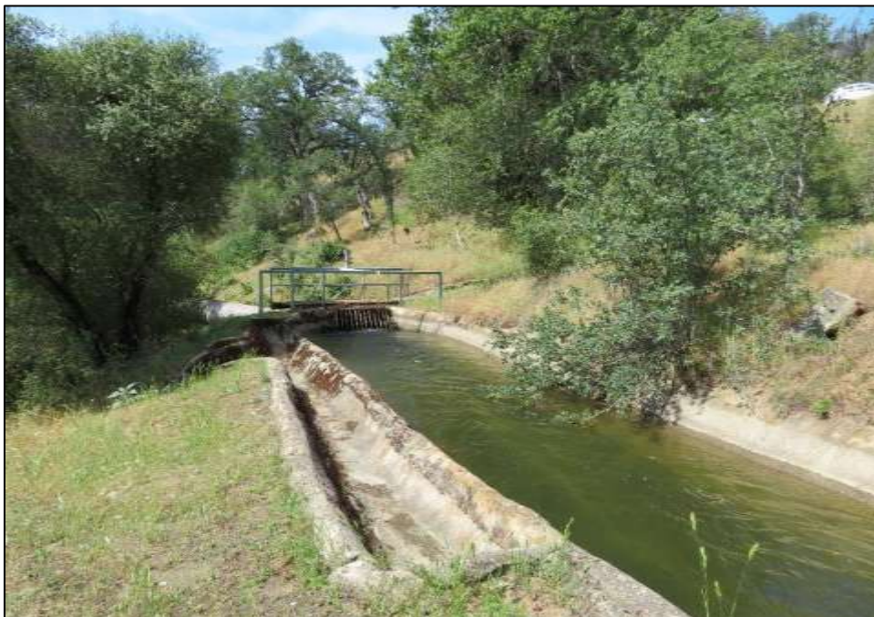
Photograph 9. Spillway and entry trashrack at transition to siphon pipe, camera facing southwest. May 8, 2018.
