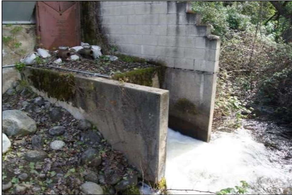
Photograph 10. Concrete tailrace channel, April 18, 2018.
