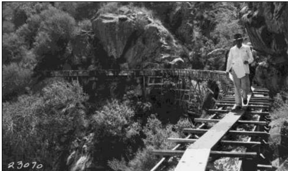
Figure 2. Men walking on Kaweah No. 1 Flowline, note redwood box flume, 1940 (Huntington Library, Call Number 02 - 23070).
