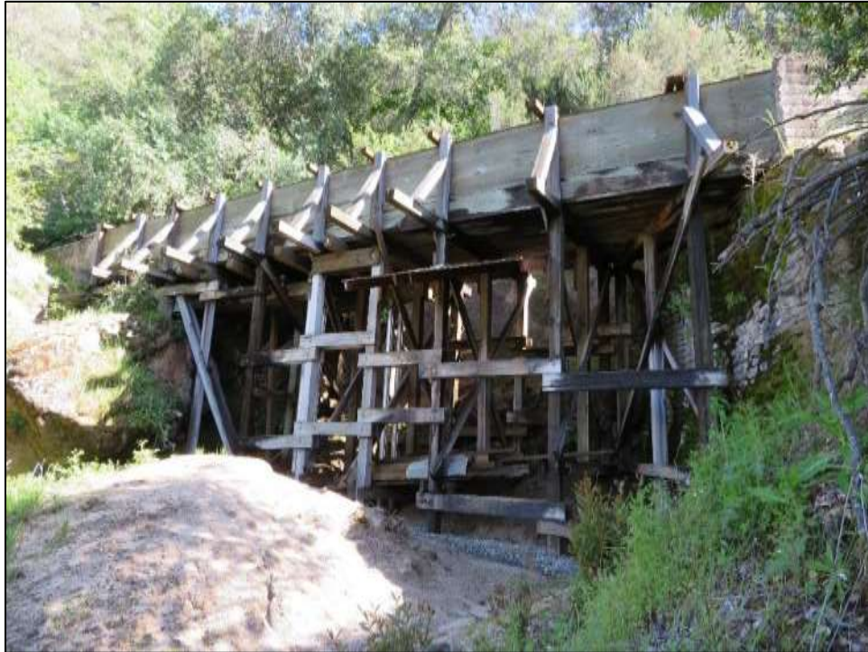
Photograph 6. Modern wood flume section, camera facing south. April 17, 2018.
