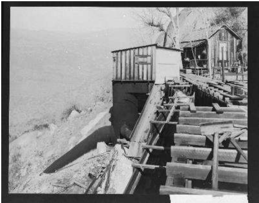
Figure 7: Kaweah No. 1 Flume at Powerhouse No. 1 Penstock, circa 1908 (Huntington Digital Library, SCE Photograph Collection, Call Number 04 - 00724)
