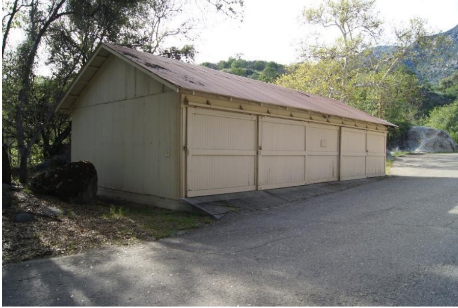
Figure CUL 5-49 Kaweah No. 3 Powerhouse Garage, camera facing northwest
