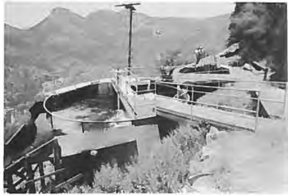
Penstock Intake Kaweah Powerhouse No. 1 View to N Roll 2, Frame 27, 6-28-89
