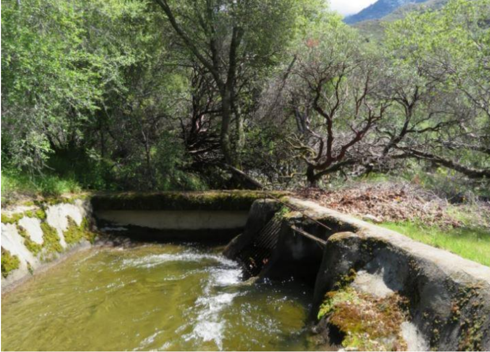
Figure CUL 5-55 Marble Fork Siphon Headbox, camera facing southeast
