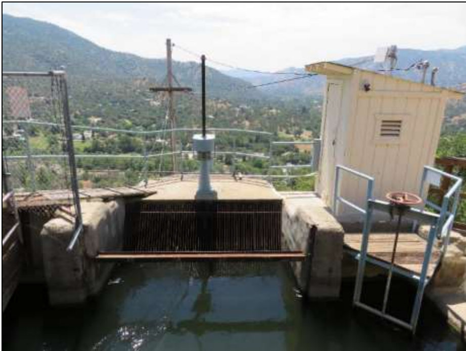
Photograph 3. Trash rack at entry into Kaweah No. 2 Penstock, camera facing southwest. May 8, 2018.
