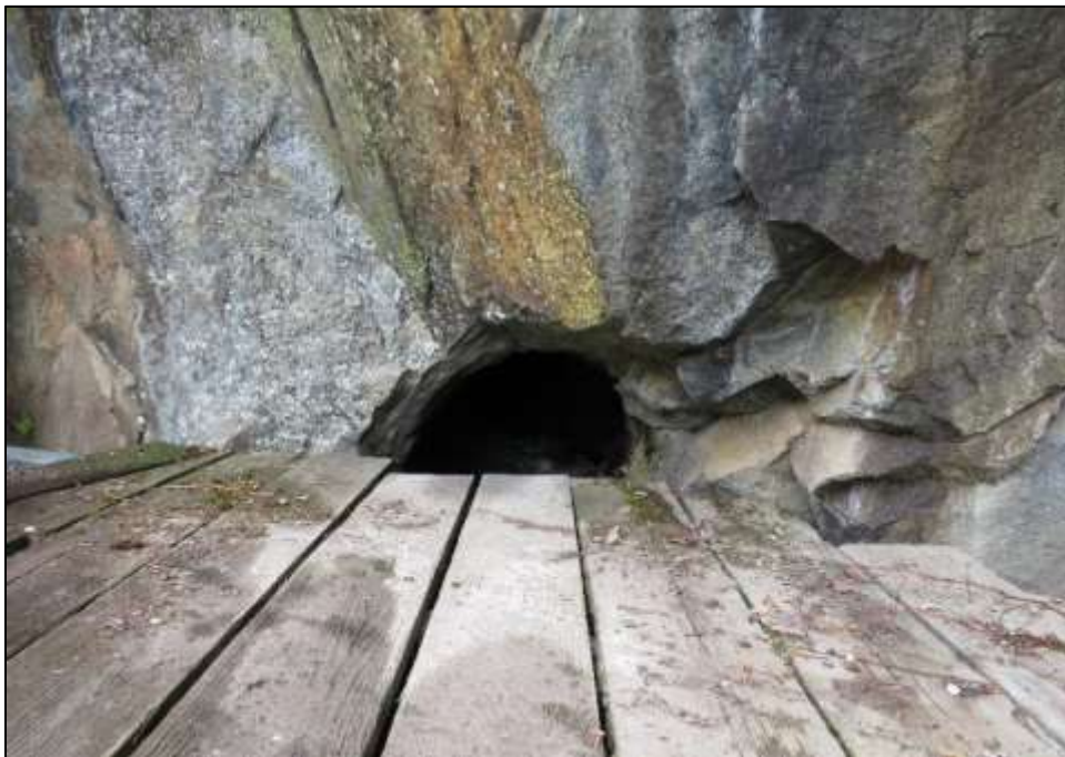
Photograph 3. Kaweah No. 1 Diversion Tunnel, camera facing northeast. April 18, 2018.
