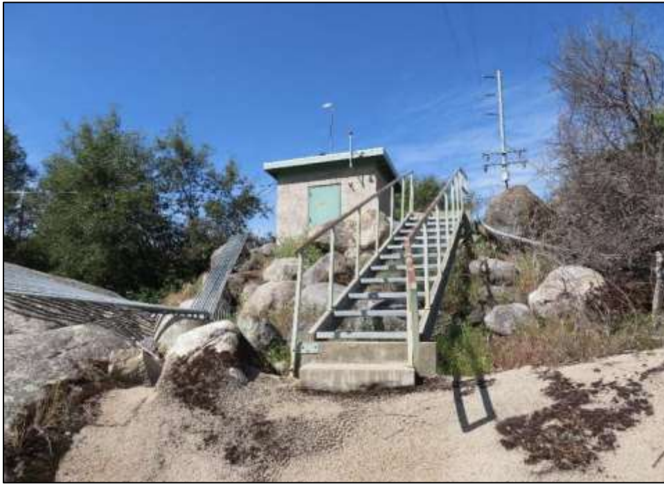
Photograph 4. Control Building. Camera facing north. April 18, 2018.
