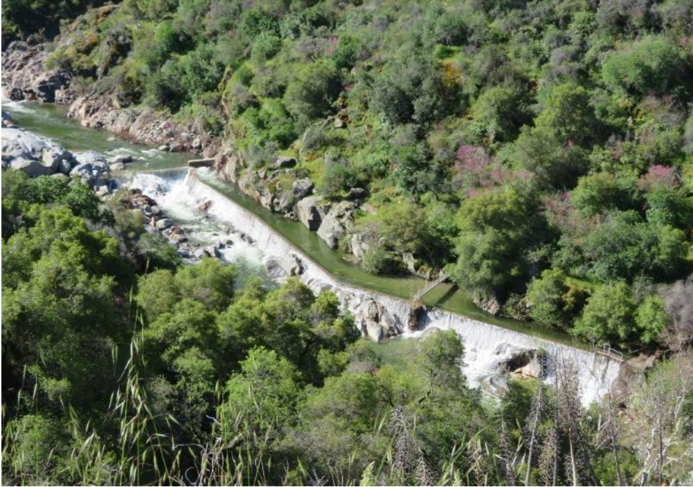
Figure CUL 5-58 Middle Fork Diversion Dam, camera facing east
