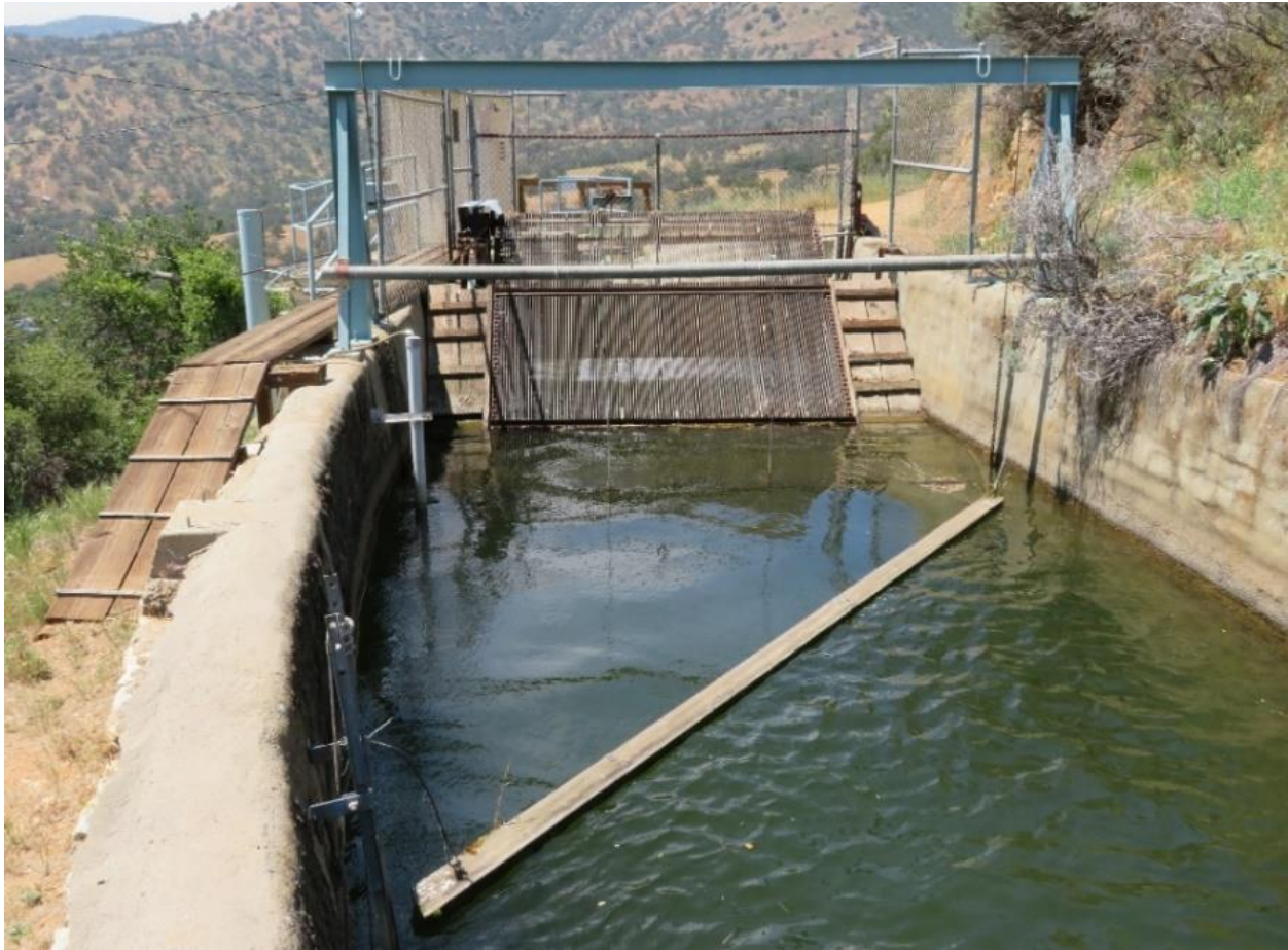
Figure CUL 5-46 Kaweah No. 2 Forebay and Trash Rack, camera facing west
