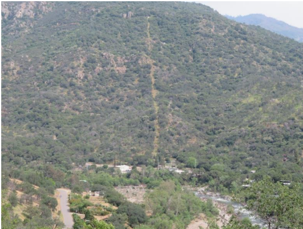
Figure CUL 5-30 Kaweah No. 1 Penstock alignment, camera facing south
