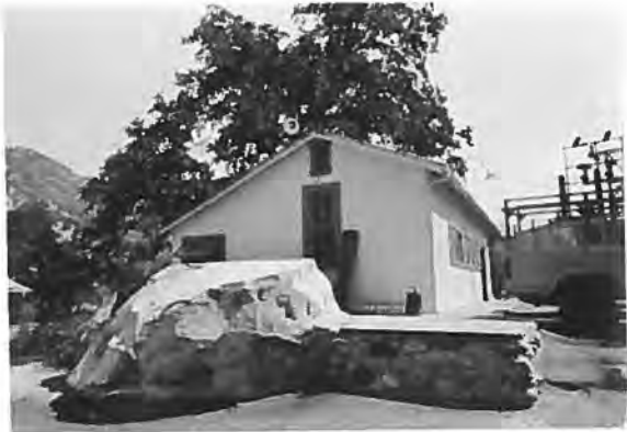
Bldg. 0107, Shop Kaweah Powerhouse No. 1 View to N Roll 1, Frame 15, 6-27-89
