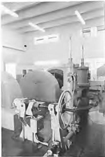
Bldg. 0101, Generator Floor Kaweah Powerhouse No. 3 View to N Roll 2, Frame 4, 6-27-89
