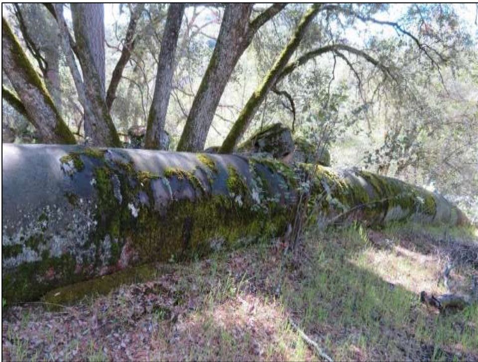
Photograph 7. Marble Fork Siphon, camera facing southeast. April 17, 2018.
