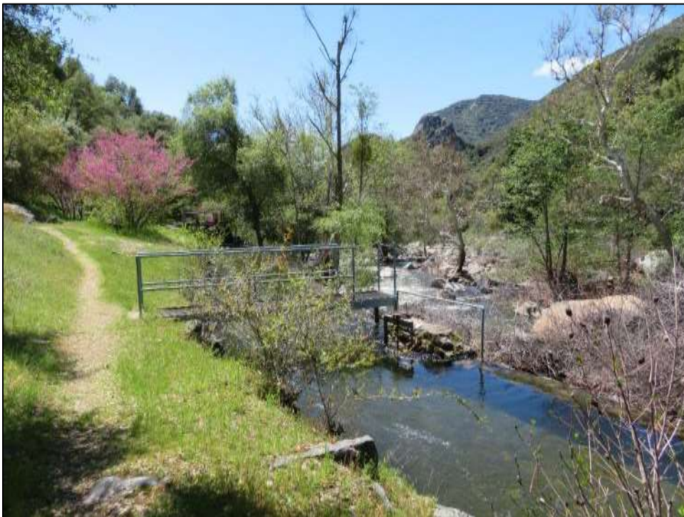
Photograph 5. Marble Fork Diversion Sandbox showing grated platform and sluice gate, camera facing south. April 17, 2018.
