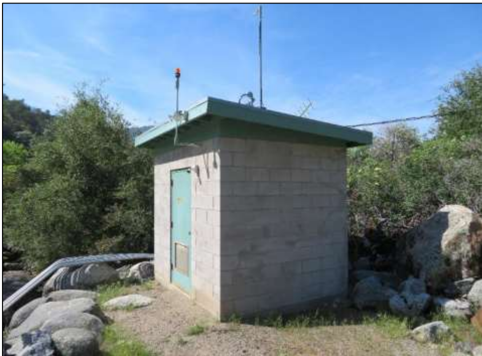
Photograph 5. Control Building. Camera facing west. April 18, 2018.
