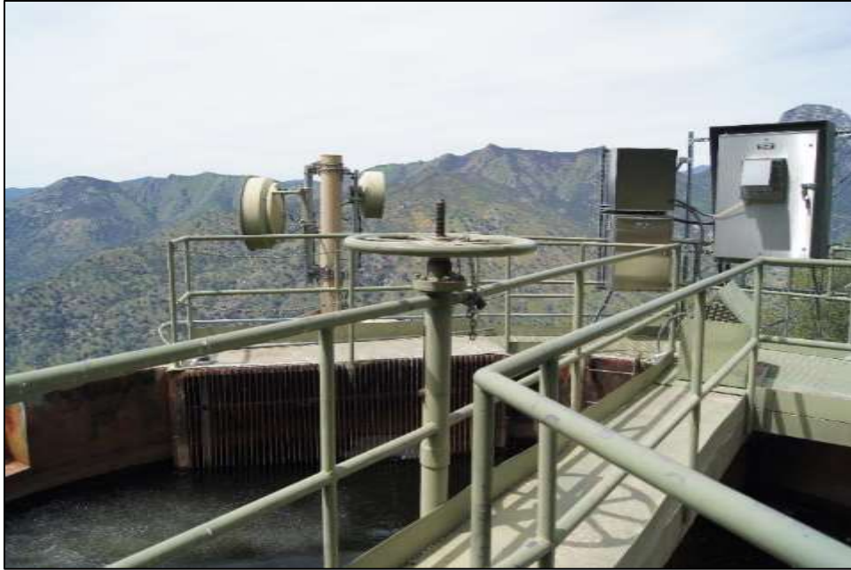
Photograph 3. Metal trash rack at penstock connection, camera facing northwest. April 18, 2018.
