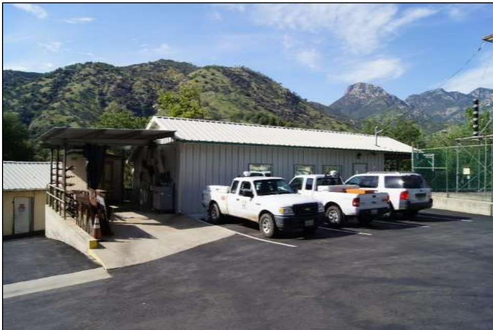
Photograph 5. Operator's Office, showing south and west sides, camera facing northeast. April 18, 2018.
