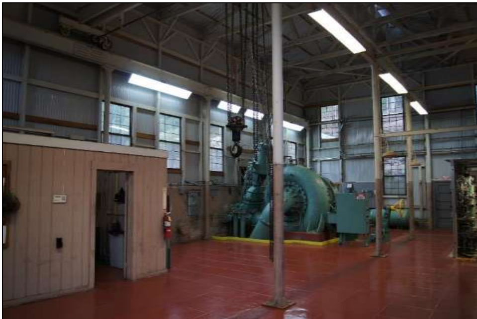
Photograph 7. Interior of Kaweah Powerhouse No. 2, camera facing northwest. April 19, 2018.
