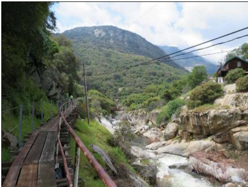
Photograph 2. Distribution line along Kaweah No. 1 Flowline, camera facing west, April 18, 2018.
