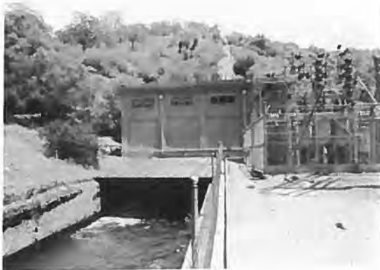
Bldg. 0101, Tailrace and Substation Kaweah Powerhouse No. 3 View to SW Roll 2, Frame 9, 6-27-89
