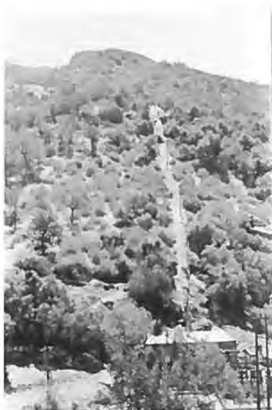
Penstock Kaweah Powerhouse No. 3 View to SE Roll 2, Frame 25, 6-28-89
