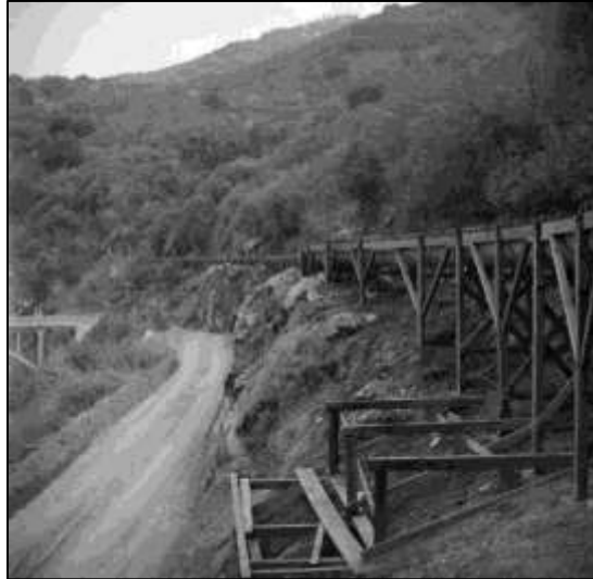
Figure 3. Kaweah No. 1 Flowline at Kaweah River Bridge following reconstruction, note metal flume, 1948 (Huntington Library, Call Number 02 - 26553).
