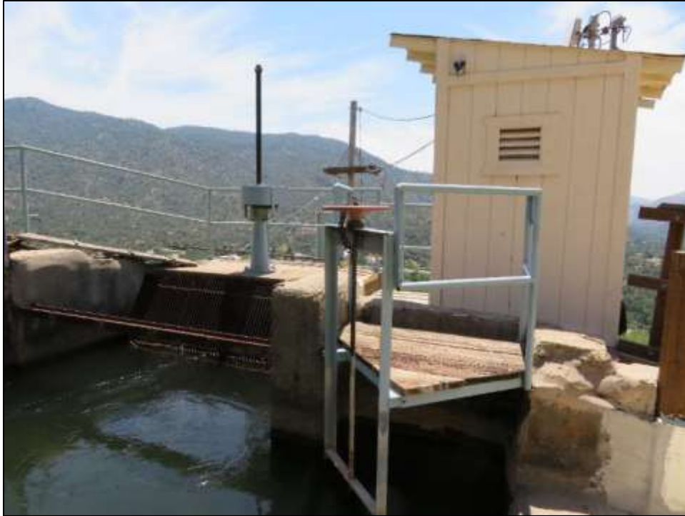
Photograph 6. Control building and slide gates, camera facing south. May 8, 2018.
