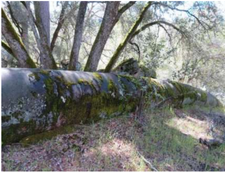
Photograph 4. Marble Fork Siphon, camera facing east. April 17, 2018.
