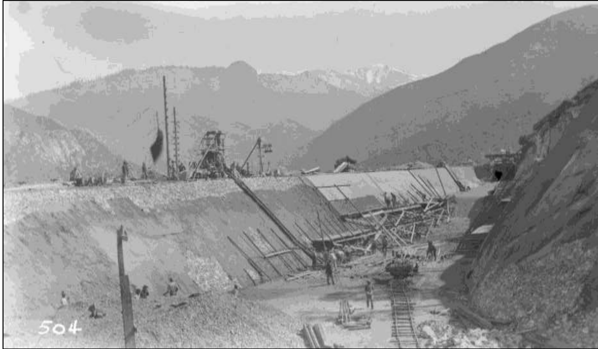
Figure 1. Kaweah No. 3 Forebay near completion, ca. 1912 (Huntington Library, Call Number 04 - 00504).
