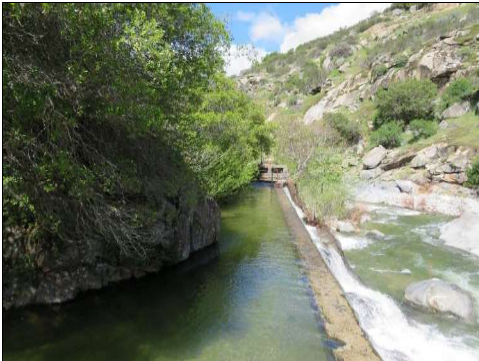
Photograph 3. Concrete sandbox, camera facing west. April 17, 2018.
