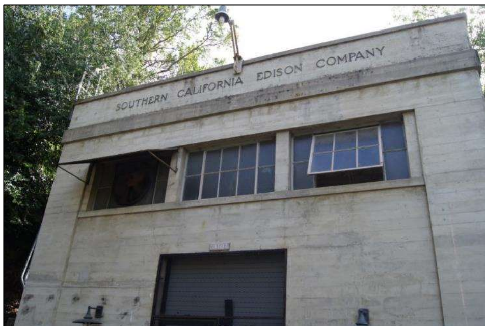
Photograph 8. West side of Kaweah No. 1 Powerhouse, camera facing west, April 18, 2018.
