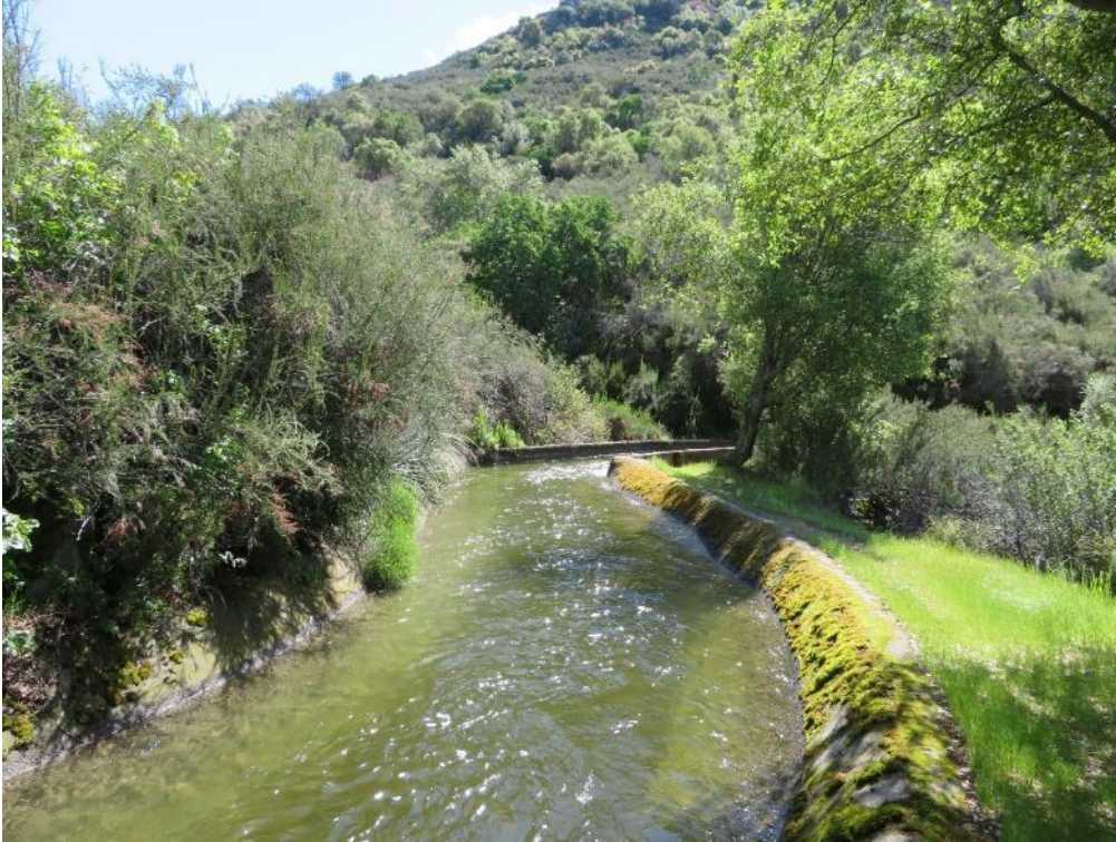
Figure CUL 5-61 Middle Fork Flowline concrete ditch section, camera facing south
