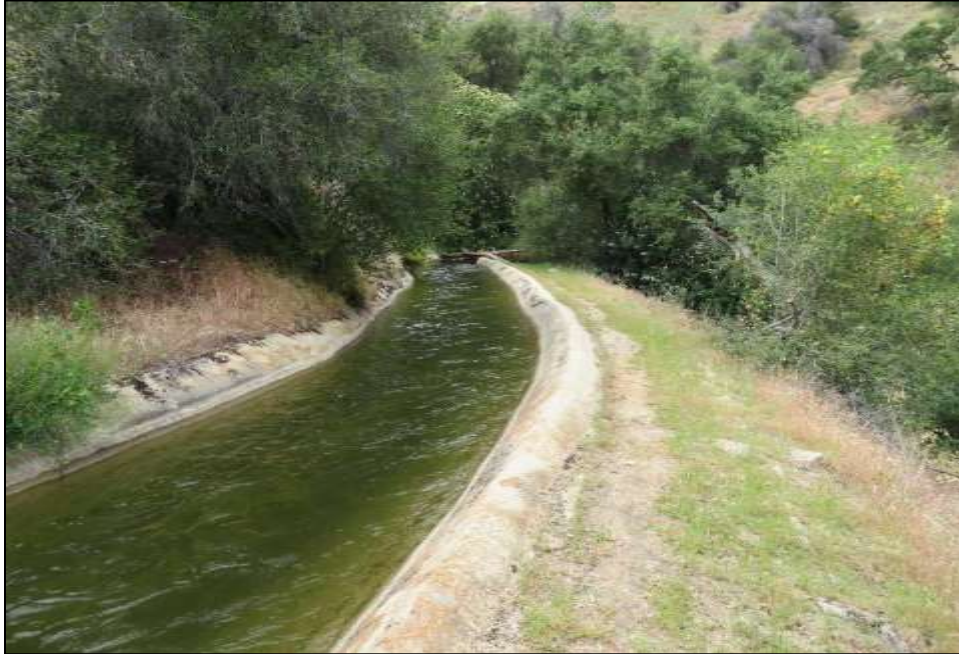
Photograph 2. Concrete lined ditch segment of Kaweah No. 2 Flowline, camera facing northeast. May 8, 2018.
