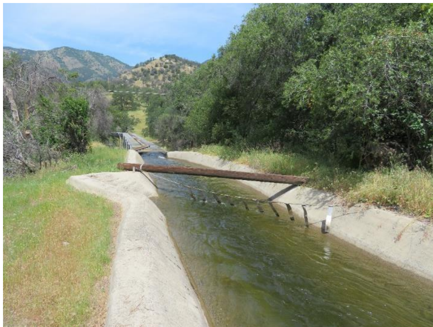
Figure CUL 5-44 Kaweah No. 2 Flowline, camera facing west
