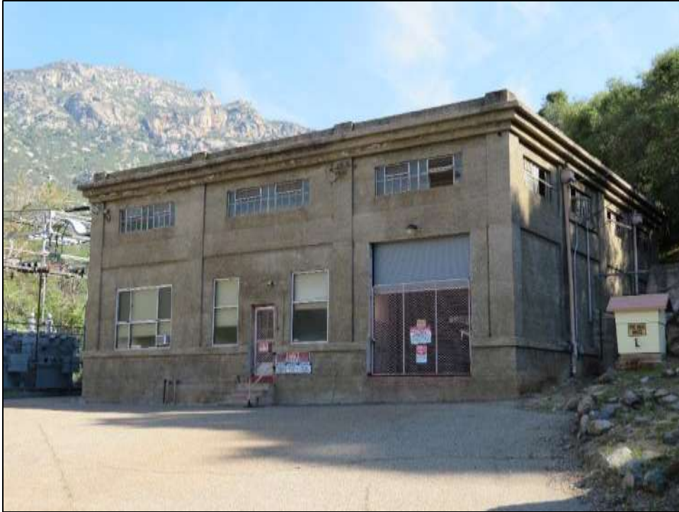
Photograph 2. Kaweah No. 3 Powerhouse, note pilasters, fenestration, and roll-up door, camera facing northwest. April 18, 2018.
