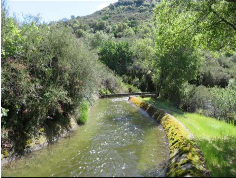
Photograph 8. Concrete-lined ditch segment along Middle Fork Flowline, camera facing south. April 17, 2018.
