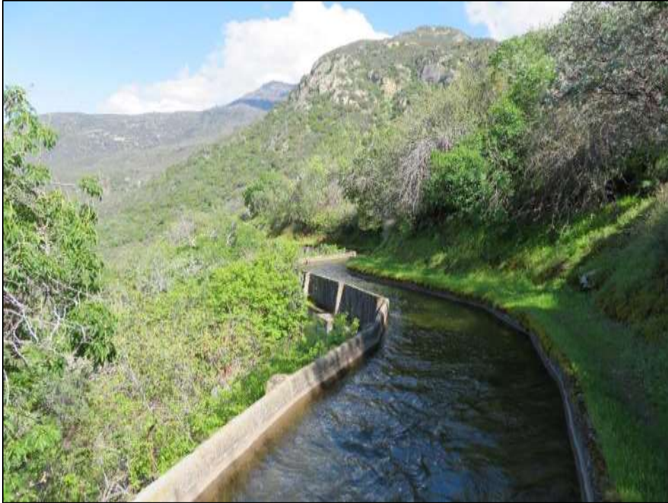
Photograph 2. Middle Fork Flowline, camera facing northeast. April 17, 2018.
