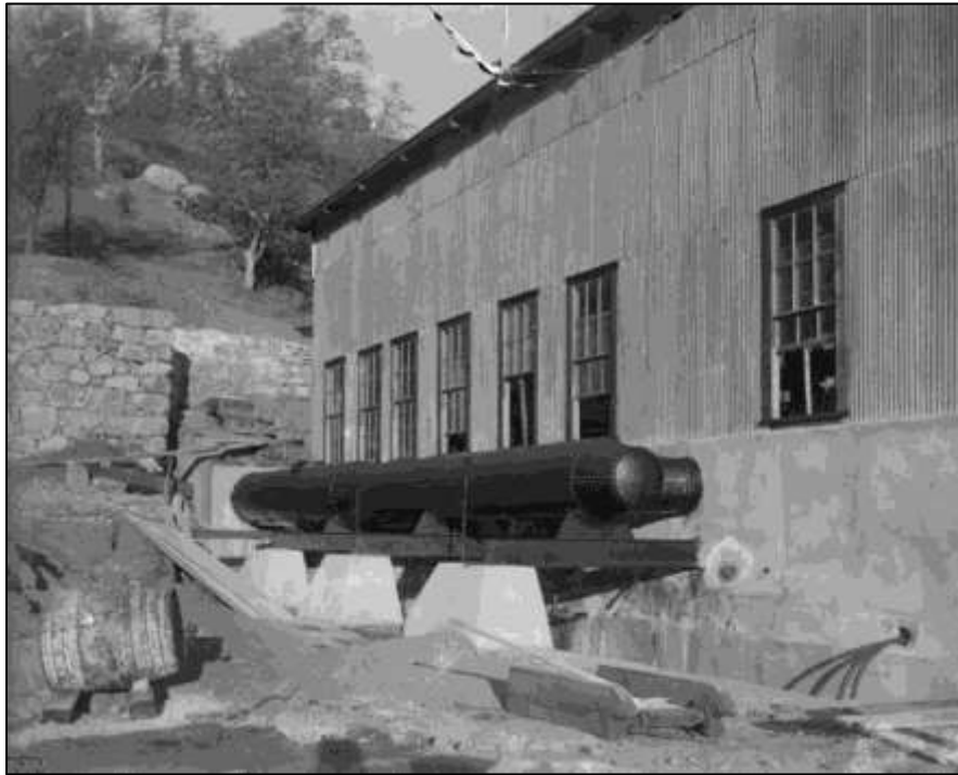
Figure 3. Kaweah No. 2 Powerhouse Penstock entering the powerhouse, 1904 (Huntington Library, Call Number 04 - 00055).
