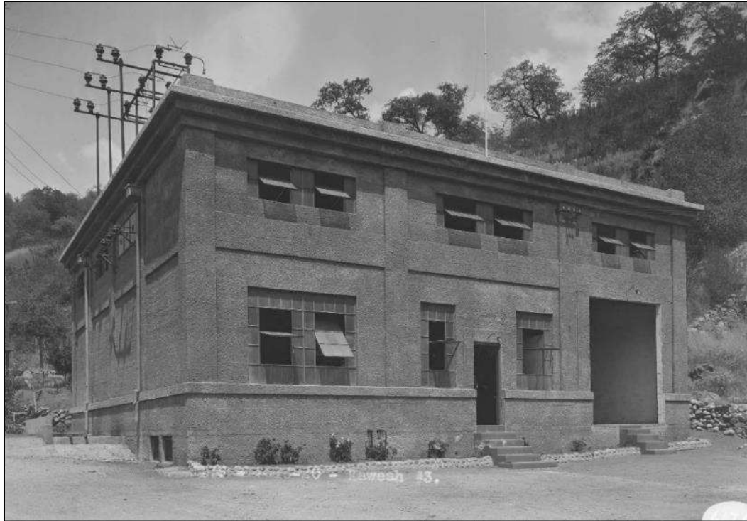
Figure 1. Kaweah No. 3 Powerhouse, 1920 (Huntington Library, Call Number 02 - 06179).
