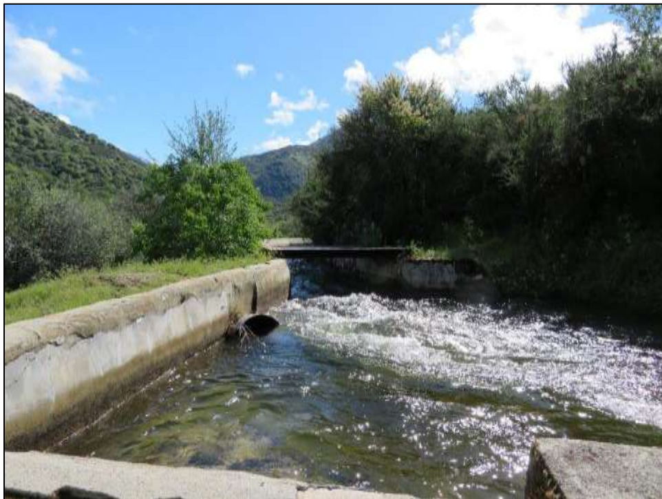
Photograph 7. Junction of Marble Fork Siphon and the Middle Fork Flowline, camera facing east. April 17, 2018.
