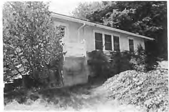
Bldg. 0121, Cottage Kaweah Powerhouse No. 1 View to SE Roll 1, Frame 23, 6-27-89
