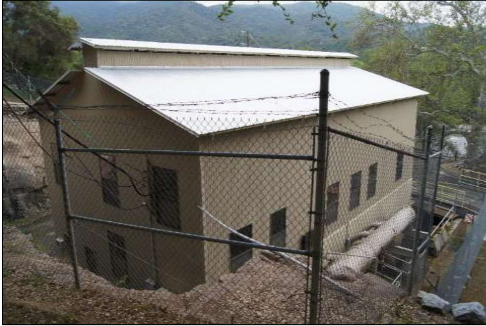
Photograph 4. Kaweah Powerhouse No. 2, camera facing west. April 19, 2018.
