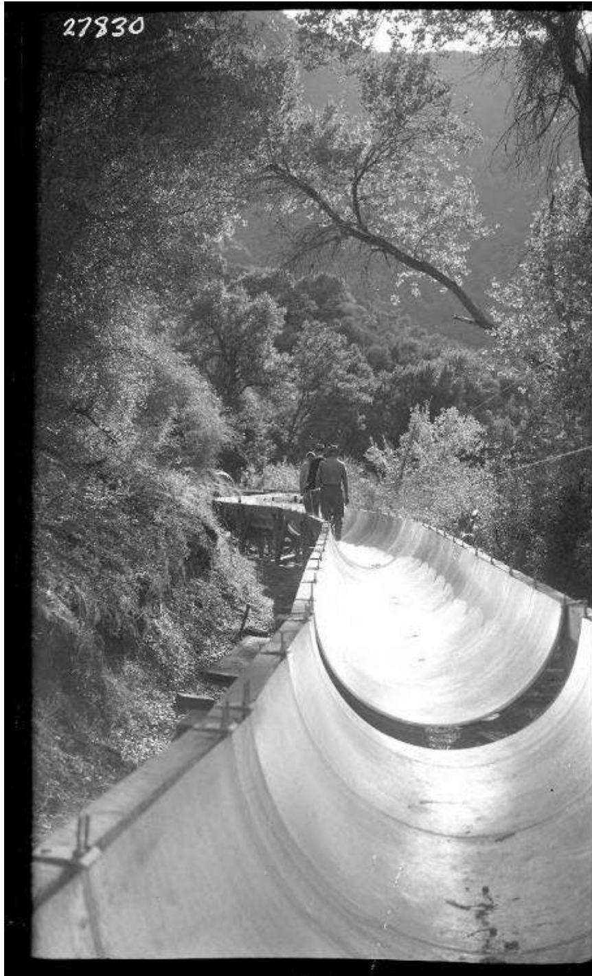
Figure 25: Rebuilt Kaweah No. 1 Flume, 1948 (Huntington Digital Library, SCE Photograph Collection, Call Number 02-27830)
