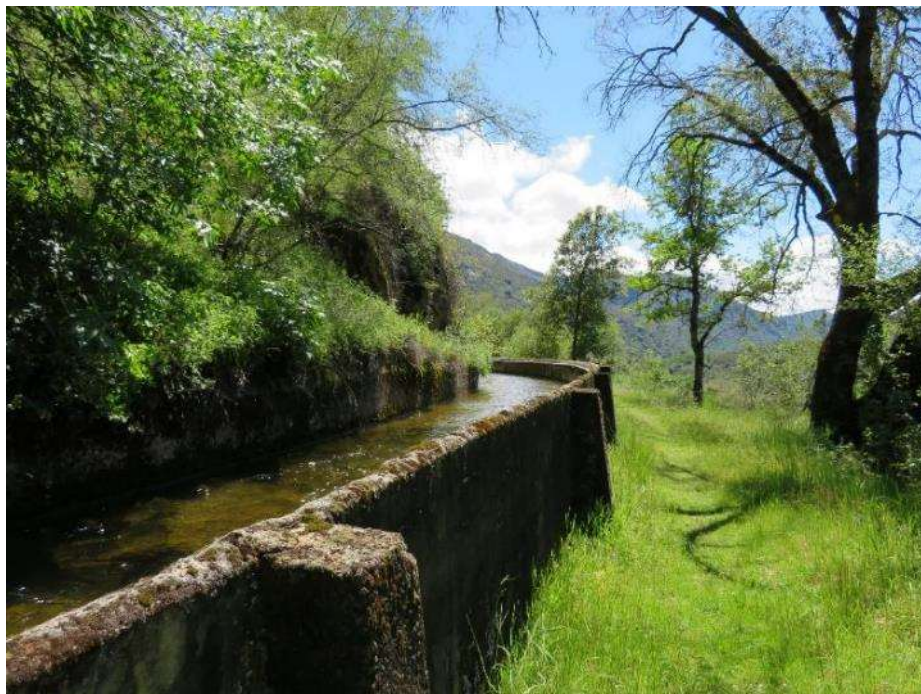
Photograph 3. Marble Fork Flowline, camera facing southwest. April 17, 201.
