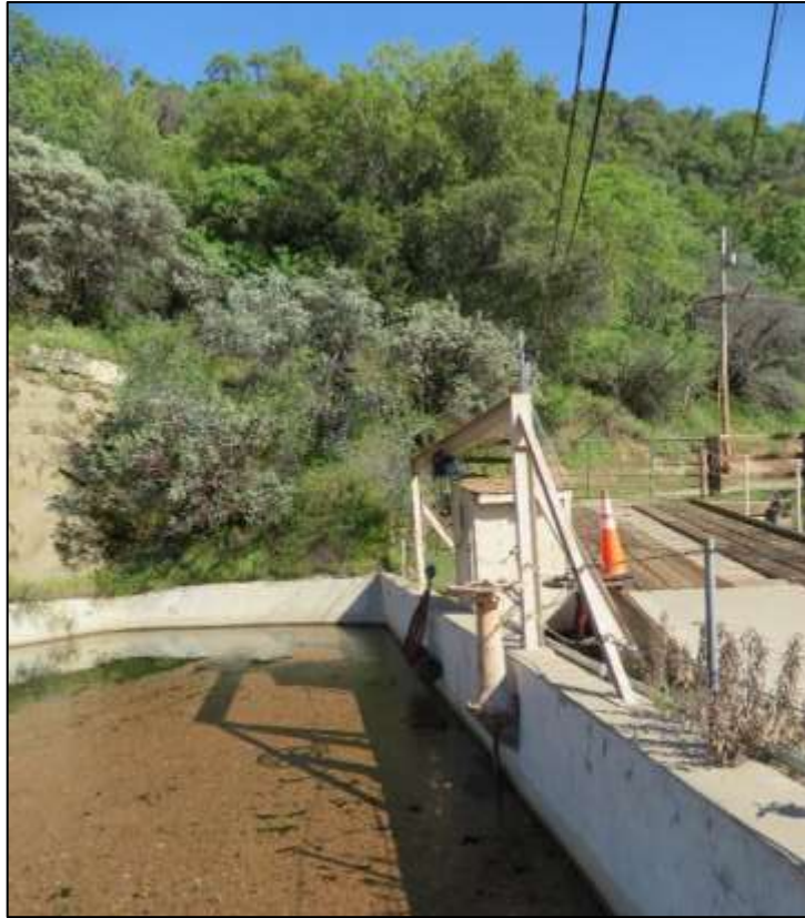
Photograph 4. Kaweah No. 3 Forebay outlet slide gate, camera facing south. April 17, 2018.
