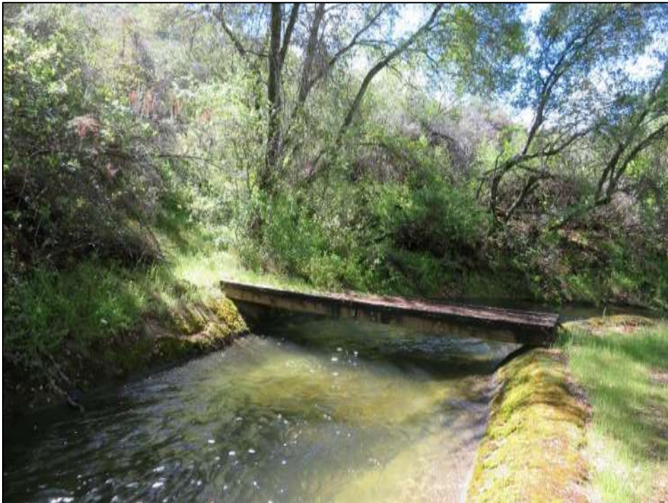
Photograph 9. Wildlife crossing along Middle Fork Flowline, camera facing south. April 17, 2018
