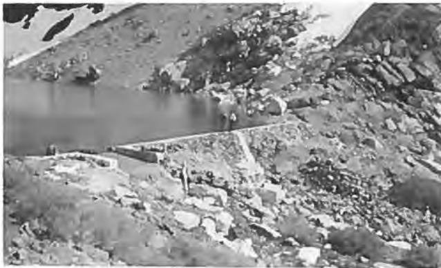
Crystal Lake Dam SCE Historical Photo Album View to SW 7-22-33
