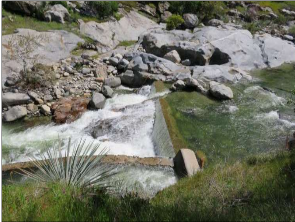
Photograph 2. Middle Fork Diversion Dam, camera facing northeast. April 17, 2018.
