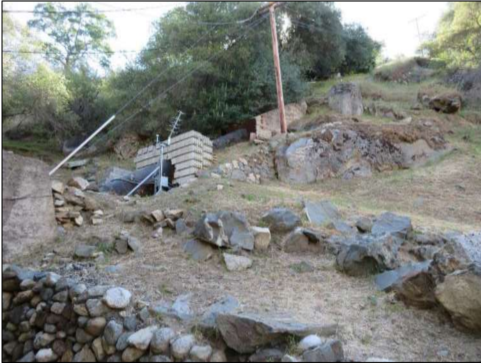
Photograph 5. Kaweah No. 3 Penstock, note support structures, camera facing northeast. April 18, 2018.
