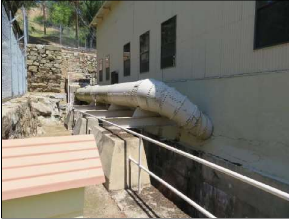
Photograph 6. North side of Kaweah Powerhouse No. 2 showing penstock, camera facing northeast. April 19, 2018.
