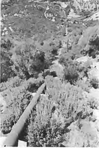
Penstock Kaweah Powerhouse No. 1 View to WNW Roll 2, Frame 31, 6-28-89
