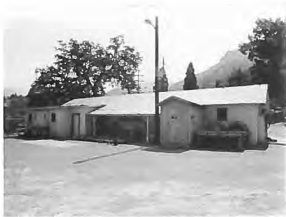
Bldg. 0110, Carpenter Shop/Garage Kaweah Powerhouse No. 1 View to NNE Roll 1, Frame 13, 6-27-89
