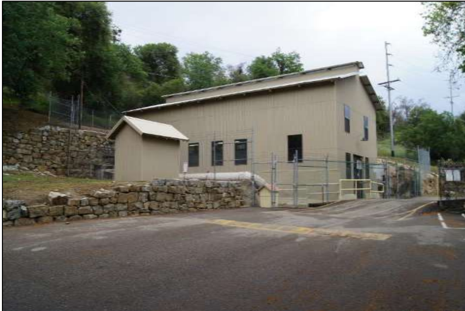
Photograph 2. Kaweah Powerhouse No. 2, camera facing west. April 19, 2018.
