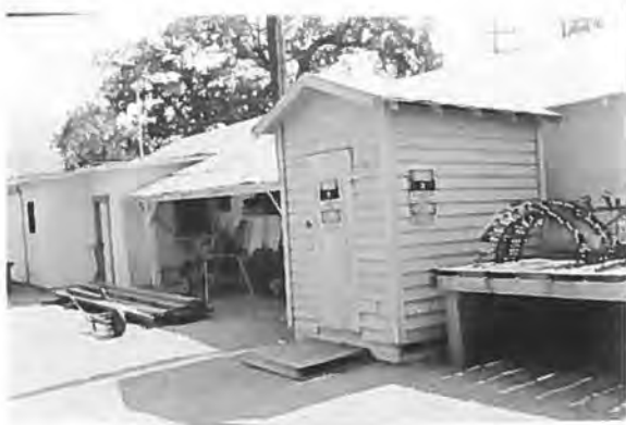
Bldg. 0128, Storage Shed Kaweah Powerhouse No. 1 View to NE Roll 1, Frame 11, 6-27-89
