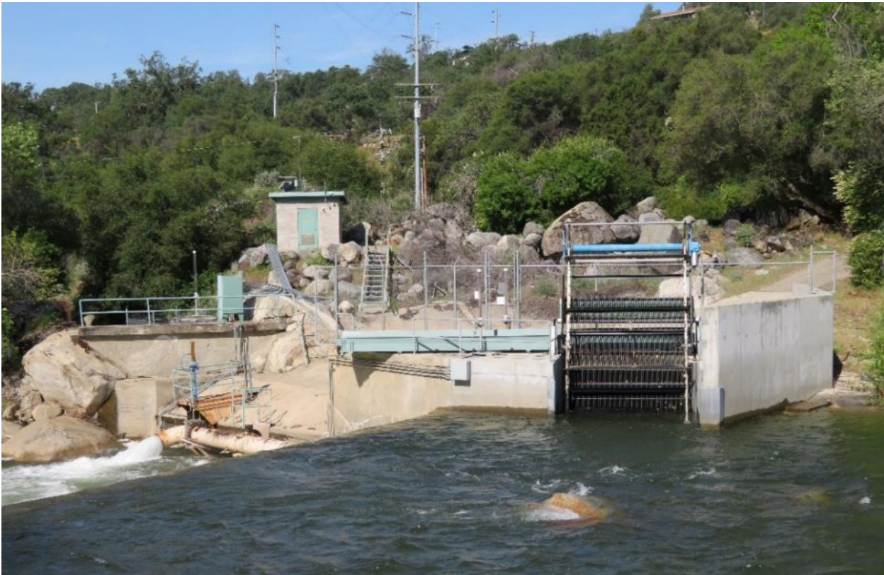
Figure CUL 5-43 Kaweah No. 2 Diversion Dam, camera facing west
