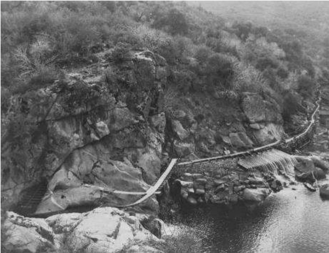
Figure 5: Overview of Kaweah No. 1 Diversion Dam with Catwalk leading to Flume (l-r), 1908 (Huntington Digital Library, SCE Photograph Collection, Call Number 04 - 00720)
