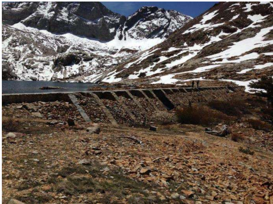
Photograph 3. Upper Monarch Lake Dam. SCE, 2018.
