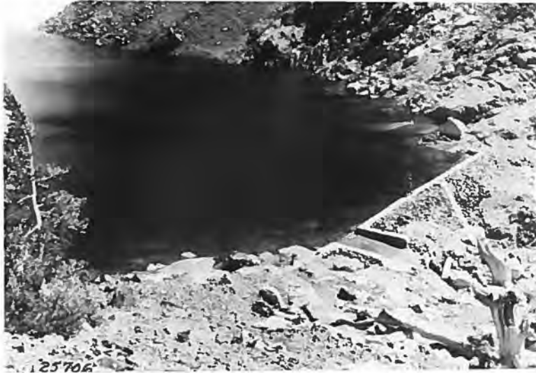
Crystal Lake Dam SCE Historical Photo Album View to SW 8-4-43
