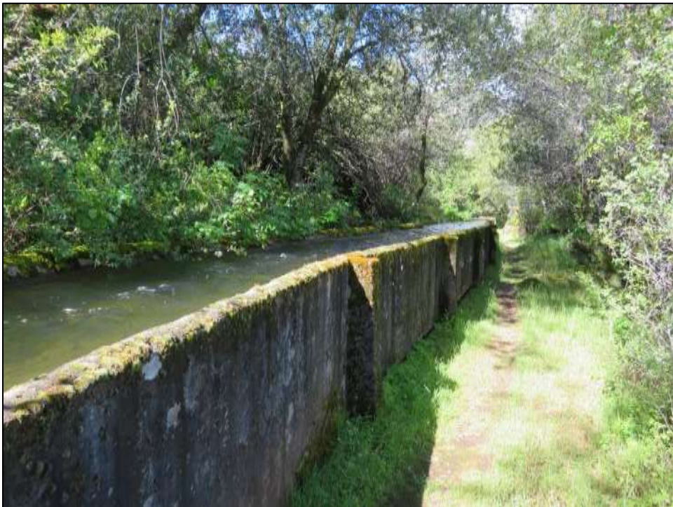
Photograph 3. Middle Fork Flowline, camera facing southwest. April 17, 2018.
