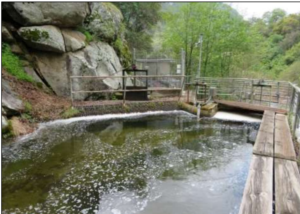
Photograph 7. West end of sandbox showing trash rack and slide gate, camera facing southwest. April 18, 2018.
