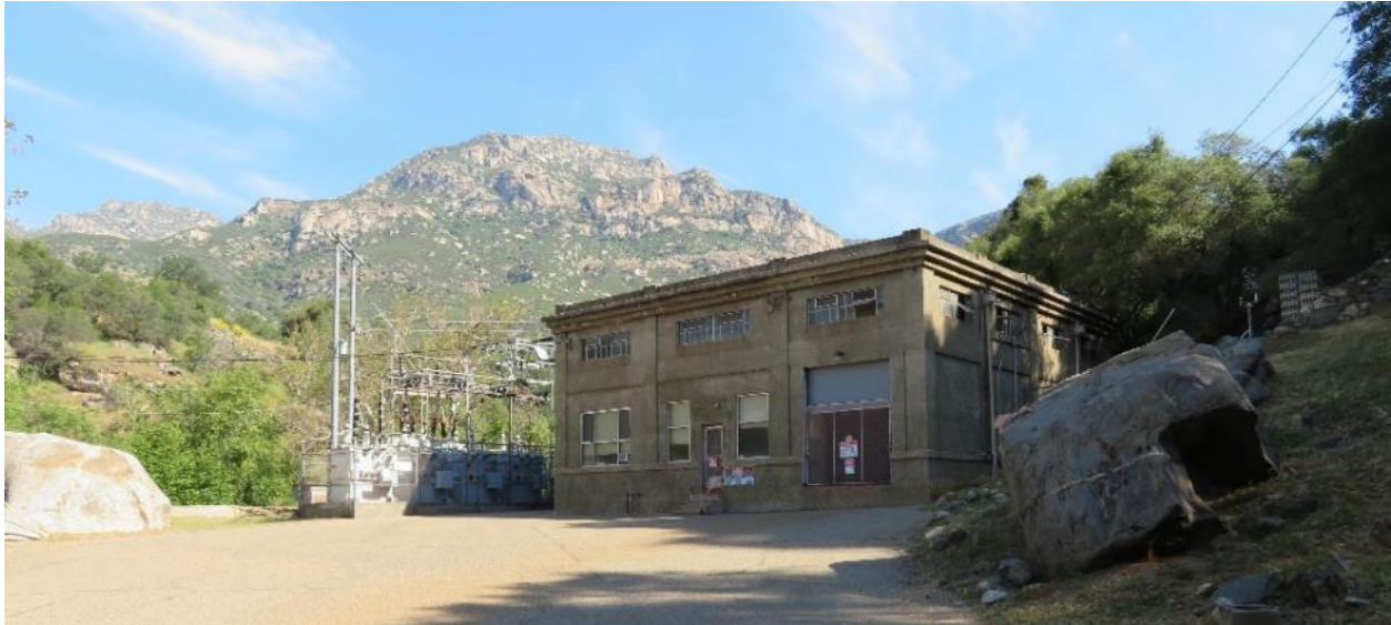
Figure CUL 5-47 Kaweah No. 3 Powerhouse, camera facing north
