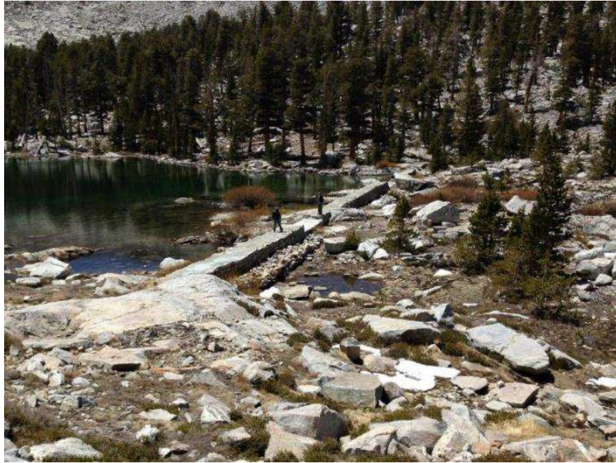
Photograph 2. Eagle Lake Dam. SCE, 2018.
