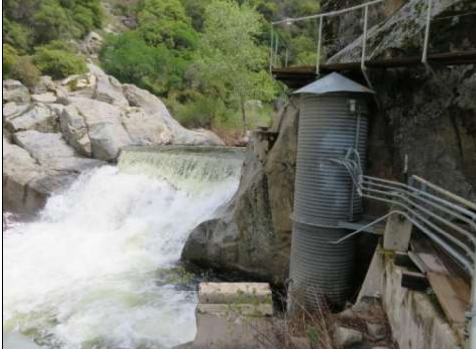
Photograph 2. Kaweah No. 1 Diversion Dam, camera facing northeast. April 18, 2018.
