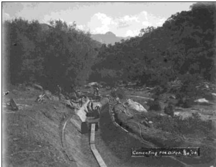
Figure 1. Construction crew cementing Kaweah No. 2 Flowline canal, 1904 (Huntington Library, Call Number 04 - 00038).
