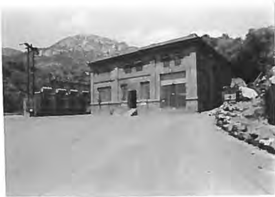
Bldg. 0101, Exterior Kaweah Powerhouse No. 3 View to SE Roll 2, Frame 2, 6-27-89
