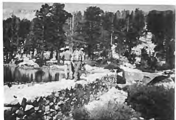
Eagle Lake Dam Kaweah Powerhouse No. 1 View to SW Courtesy, Dan Morgan, ca. 1985
