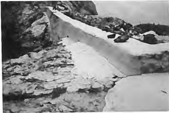
Crystal Lake Dam Kaweah Powerhouse No. 1 View to S Courtesy, Dan Morgan, ca. 1985
