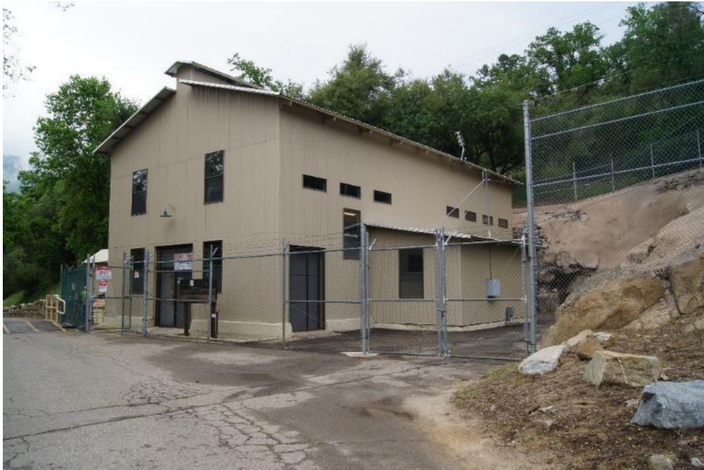
Figure CUL 5-40 Kaweah No. 2 Powerhouse, camera facing west
