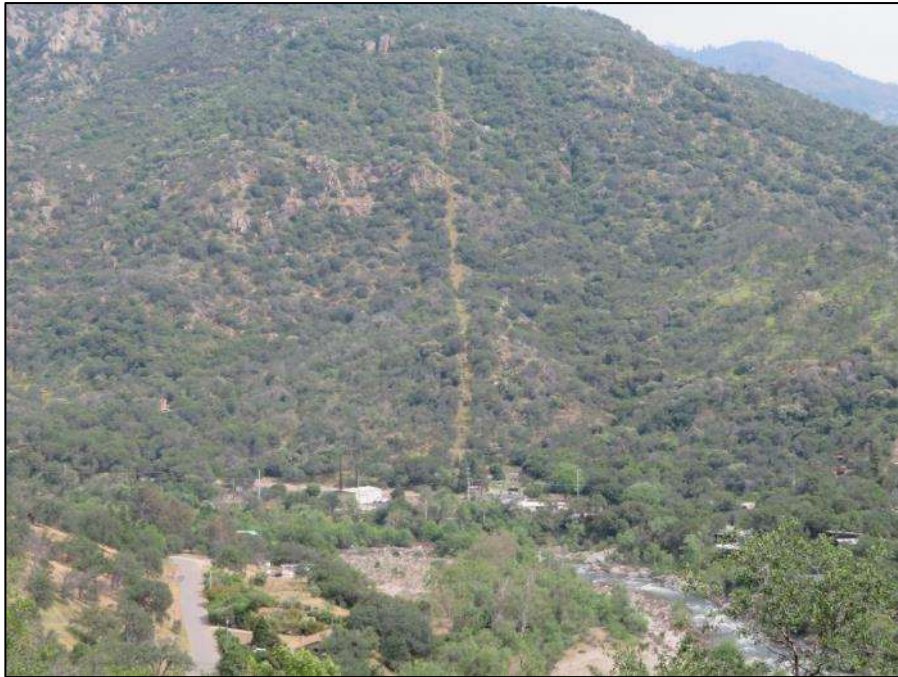
Photograph 4. Kaweah No. 1 Penstock alignment, camera facing southeast, May 8, 2018.
