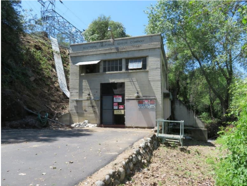
Figure CUL 5-29 Kaweah No. 1 Powerhouse, camera facing west
