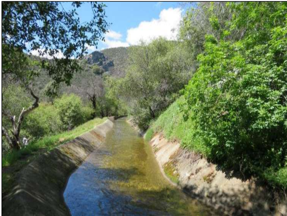
Photograph 4. Marble Fork Flowline showing concrete ditch section, camera facing north. April 17, 2018.
