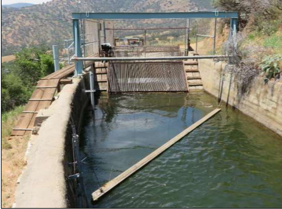
Photograph 2. Trash rack structure at Kaweah No. 2 Forebay, camera facing west. May 8, 2018.
