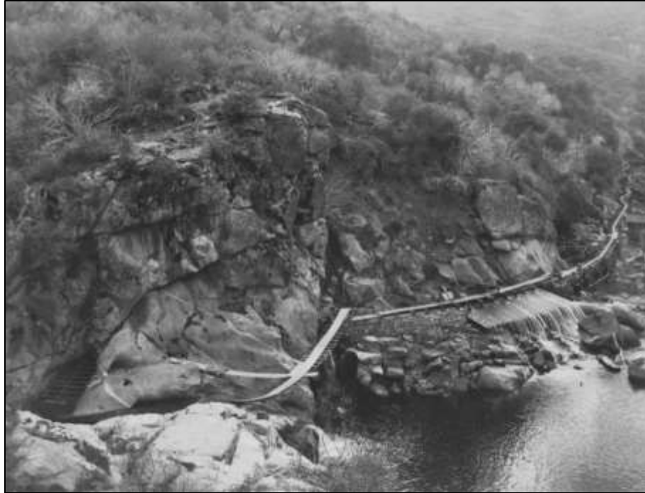
Figure 2. Kaweah No. 1 Diversion Intake, note lack of sandbox, 1904 (Huntington Library, Call Number 04 - 00720).
