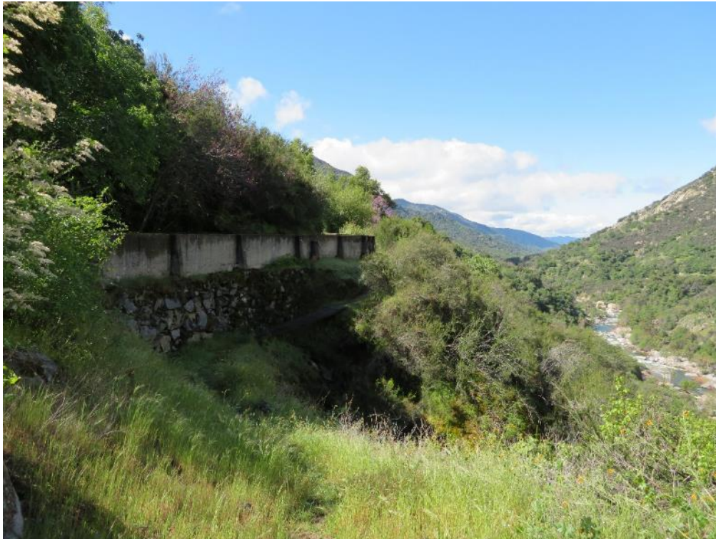
Figure CUL 5-60 Middle Fork Flowline concrete box flume section, camera facing southwest
