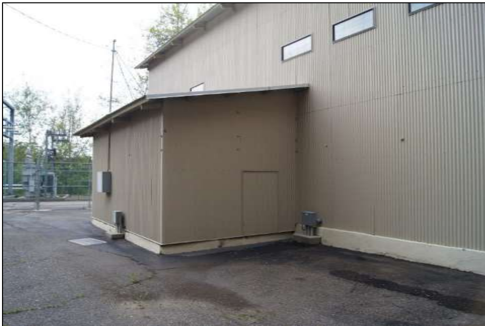
Photograph 5. West side of Kaweah Powerhouse No. 2, camera facing northeast. April 19, 2018.
