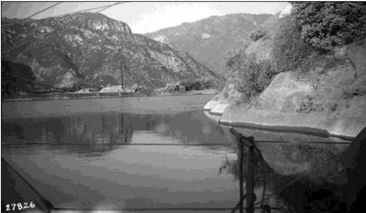
Figure 2. Kaweah No. 3 Forebay newly lined with gunite, 1947 (Huntington Library, Call Number 02 - 27826).
