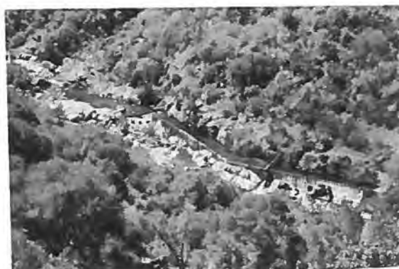
Middle Fork Diversion Kaweah Powerhouse No. 3 View to SSE Roll 2, Frame 23, 6-28-89
