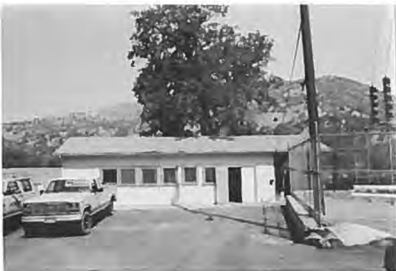
Bldg. 0107, Shop Kaweah Powerhouse No. 1 View to NW Roll 1, Frame 17, 6-27-89
