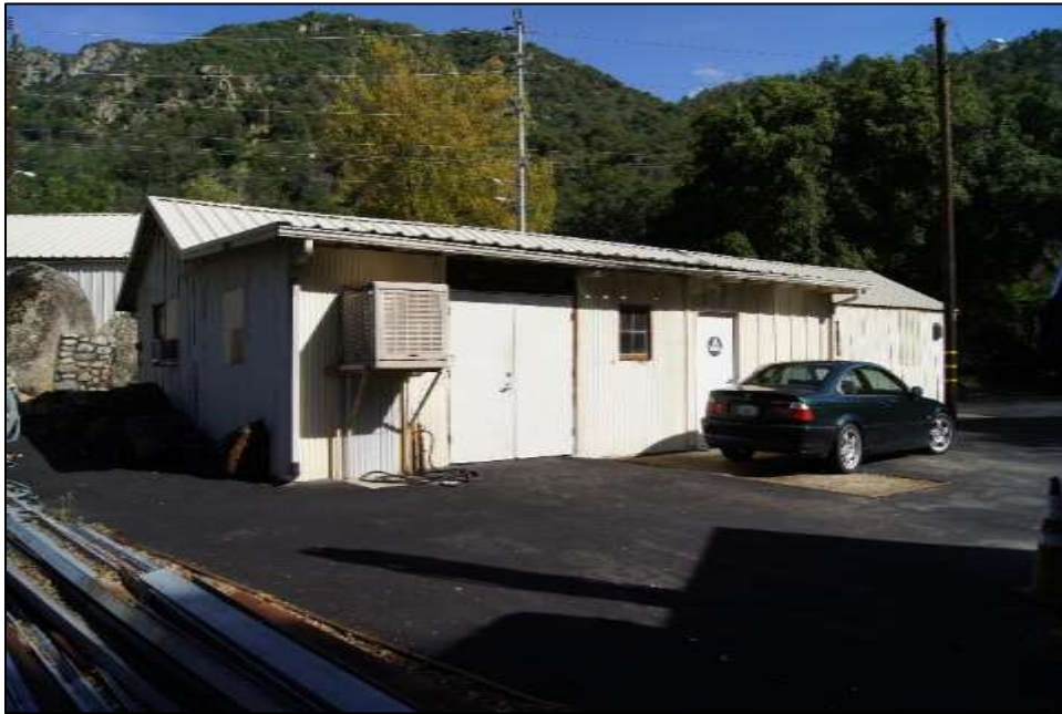
Photograph 8. Work Shop, camera facing southeast. April 18, 2018.
