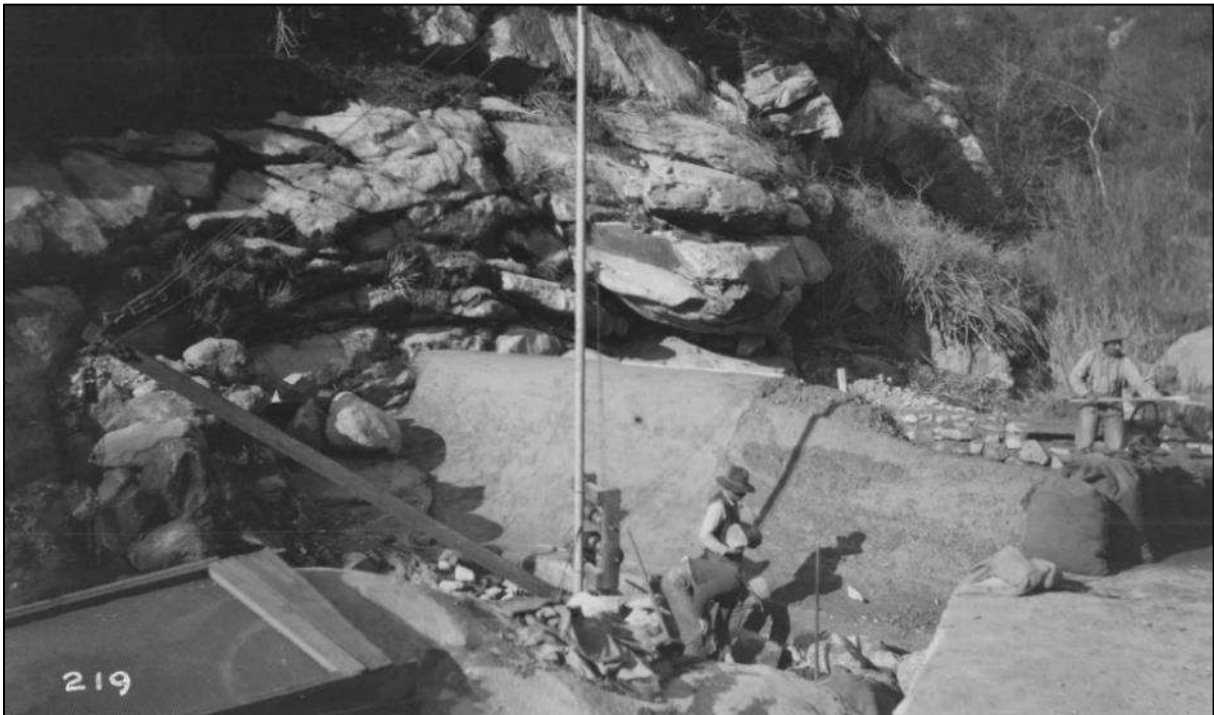
Figure 1. Construction crew at Marble Fork Diversion Dam, ca. 1912 (Huntington Library, Call Number 04 - 00219).
