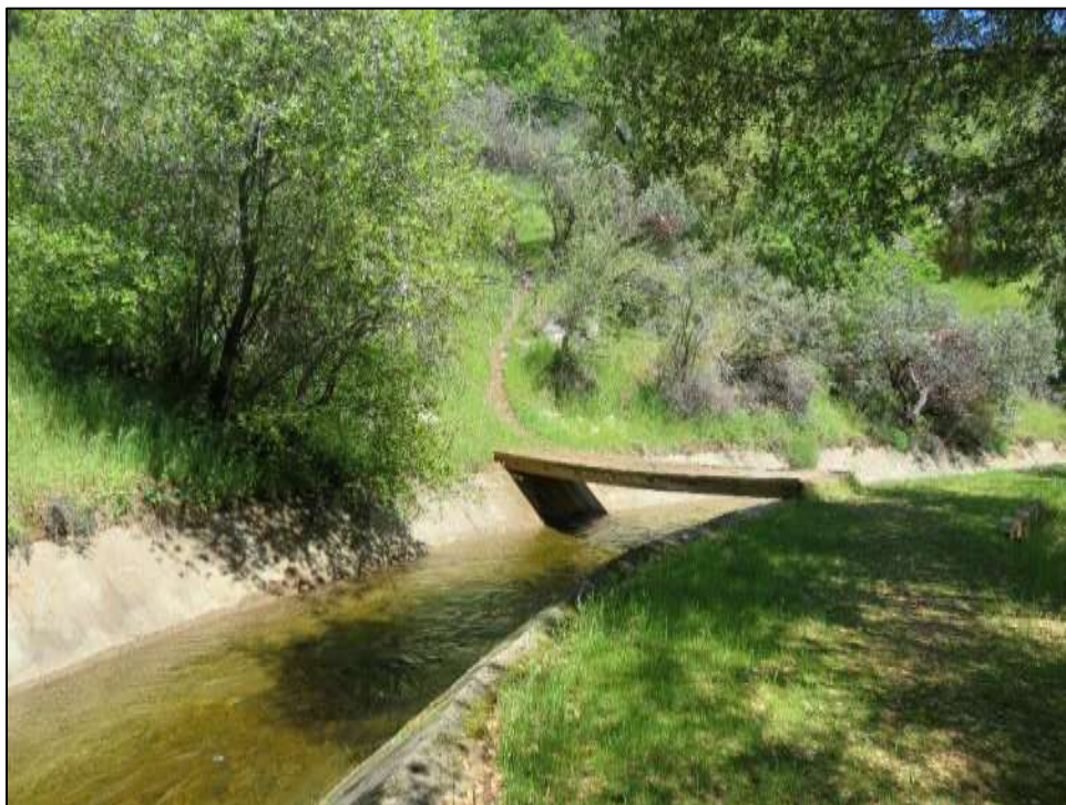
Photograph 5. Wildlife crossing on Marble Fork Flowline, camera facing southeast. April 17, 2018.
