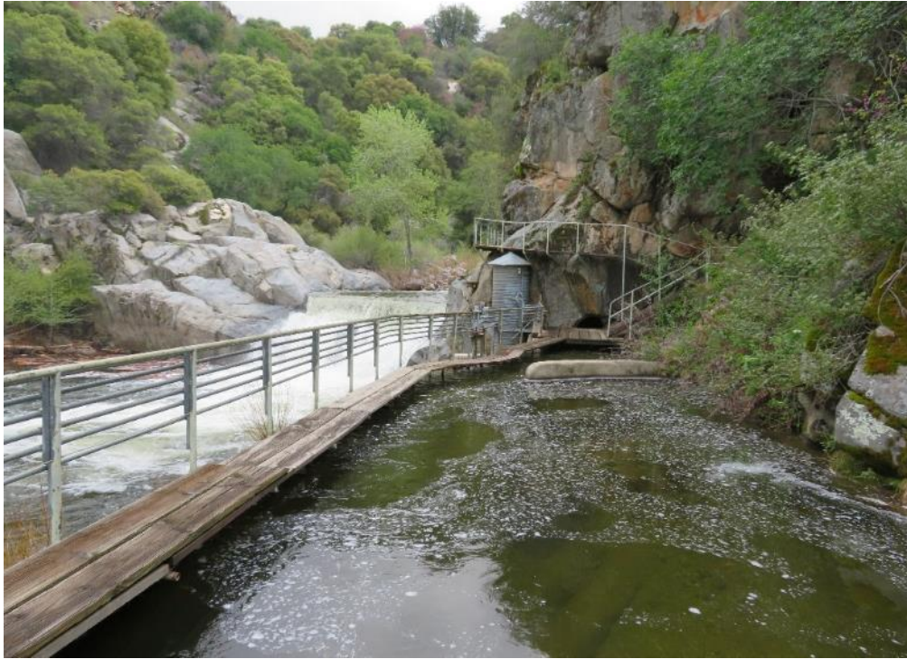
Figure CUL 5-32 Kaweah No. 1 Diversion Dam and Sandbox, camera facing east
