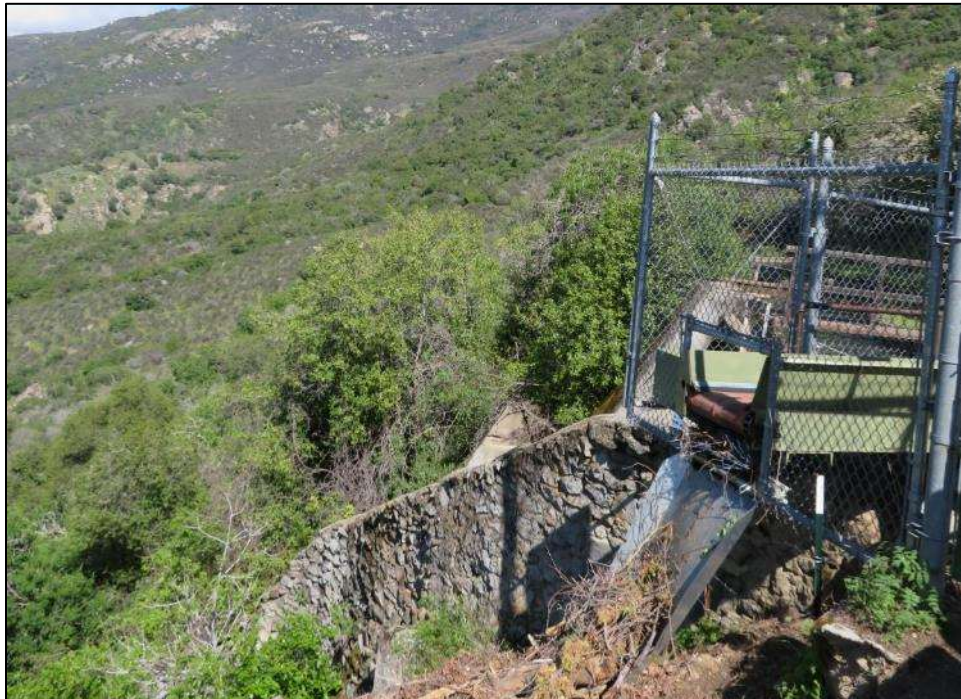
Photograph 5. Kaweah No. 3 Forebay spillway, camera facing east. April 17, 2018.
