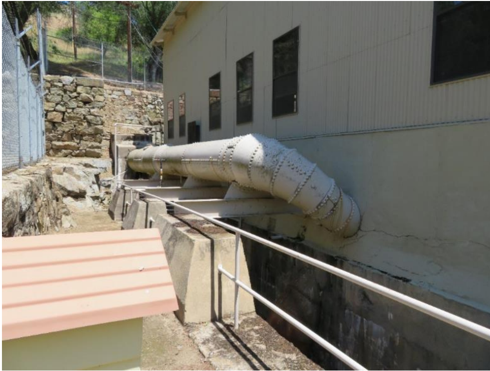
Figure CUL 5-41 Kaweah No. 2 Penstock, camera facing north
