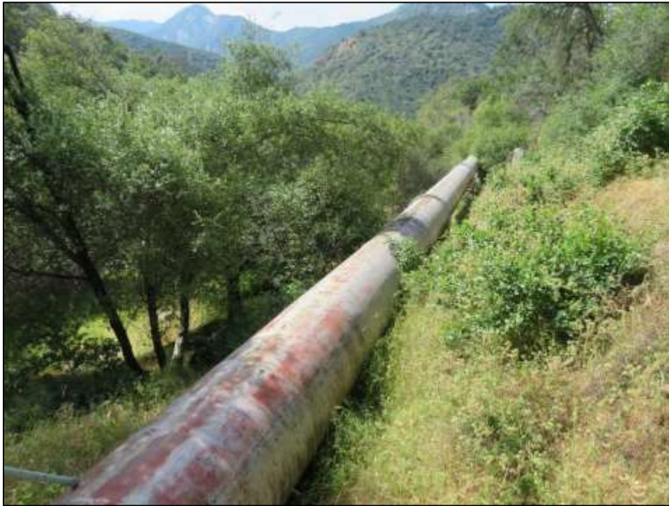
Photograph 10. Siphon pipe, camera facing southwest. May 8, 2018.
