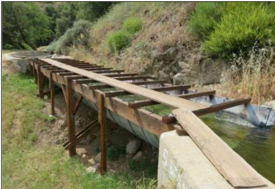
Photograph 5. Flume span along Kaweah No. 2 Flowline showing wood support structure, camera facing northwest. May 8, 2018.
