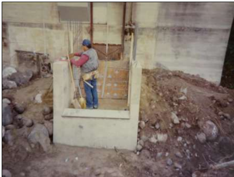
Photograph 6. Concrete tailrace channel under construction, 1991 (SCE).
