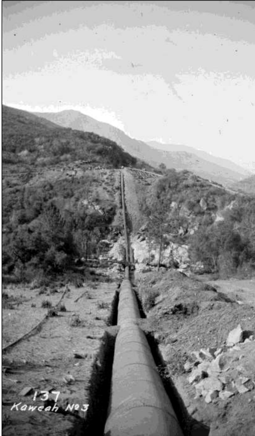
Figure 3. Marble Fork Siphon under construction, ca. 1913 (Huntington Library, Call Number 04 - 00137).
