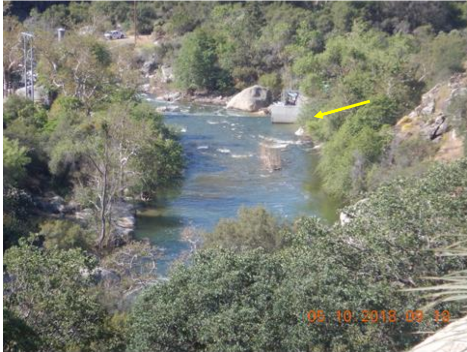
Photo A-8. Kaweah No. 2 Diversion Dam and intake structure on the Kaweah River as seen from the Indian Head Trailhead Parking Area. Camera facing southwest. May 10, 2018.
