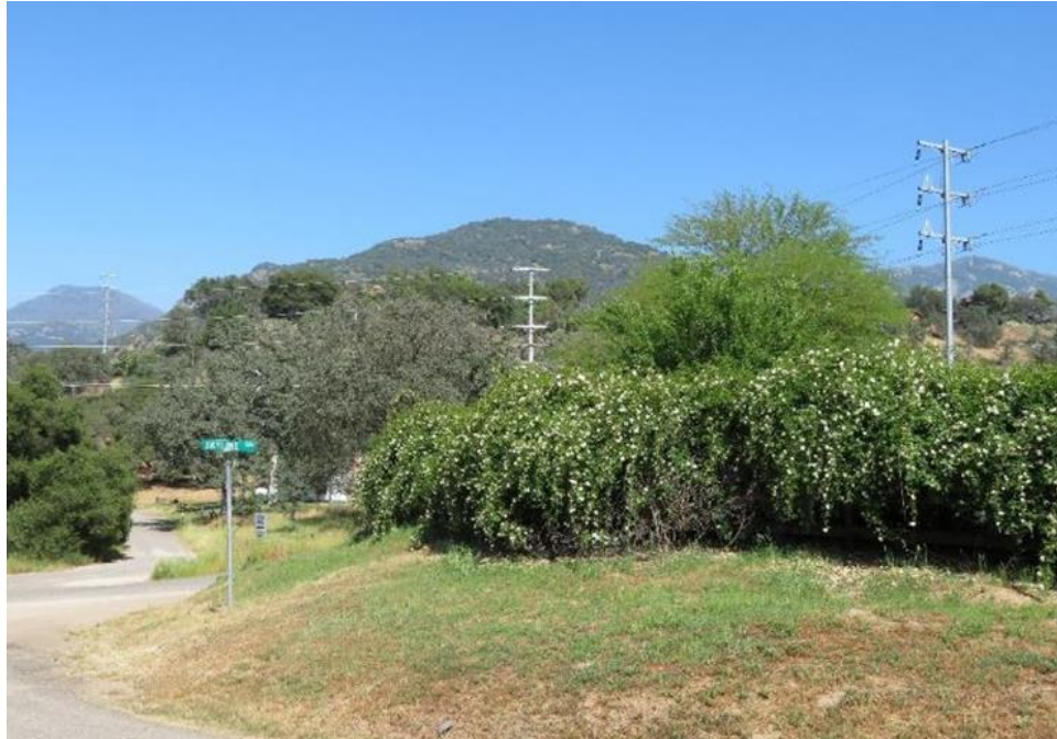
Photo A-16. Kaweah No. 3 Powerhouse to Three Rivers Substation 66 kV Transmission Line as seen from the intersection of Alta Acres and Skyline Drive. Camera facing north east. April 19, 2018.
