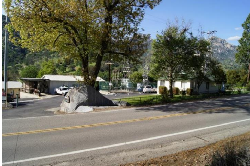
Photo A-6. Kaweah No. 1 Powerhouse Campus as seen travelling east on Highway 198. Camera facing northeast. April 18, 2018.
