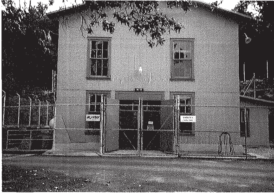
3C - Kaweah No. 2 Powerhouse
