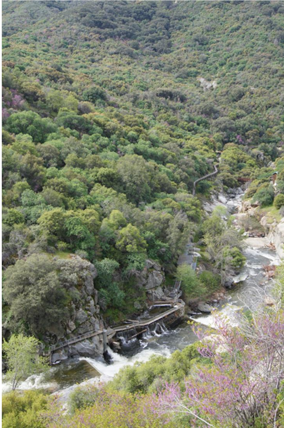
Photo A-3. Kaweah No. 1 Diversion Dam, sandbox, and flowline on the East Fork Kaweah River as viewed from below Mineral King Road. Camera facing southwest. April 17, 2018.
