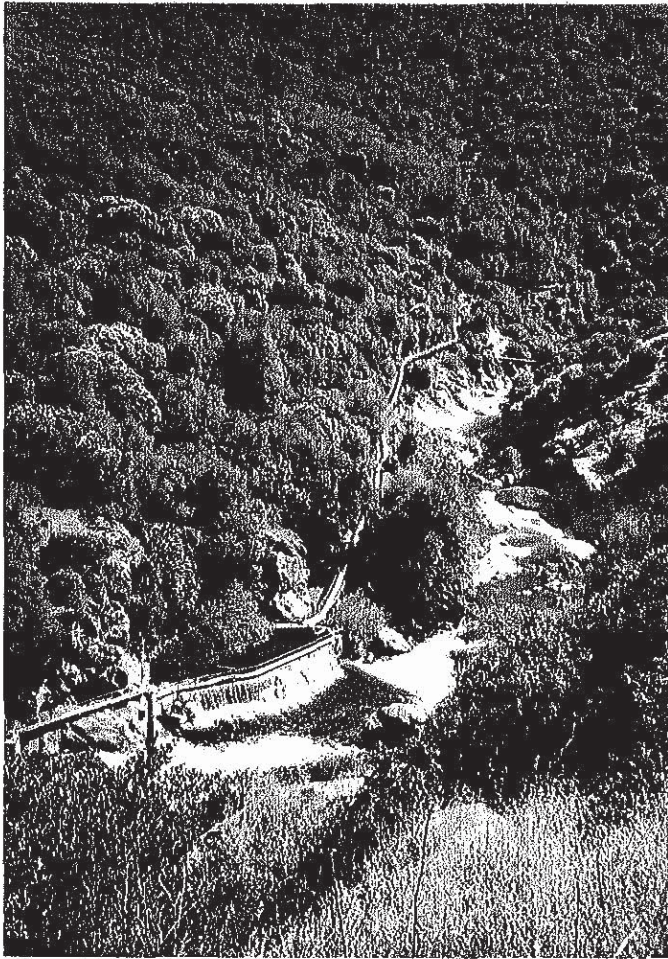
2A - East Fork Intake and Flume
