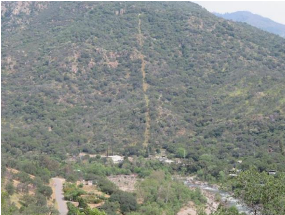
Photo A-5. Kaweah No. 1 forebay, penstock alignment and powerhouse as viewed from Dinely Road. The Kaweah River is in the foreground. Camera facing southeast. May 8, 2018.
