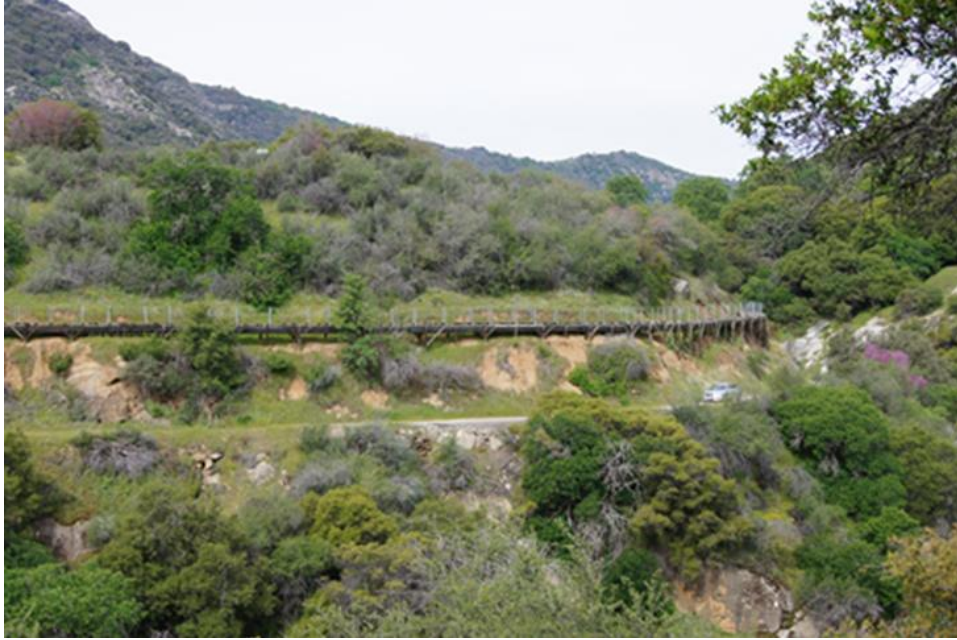
Photo A-4. Kaweah No. 1 Flowline, typical elevated steel flume section along the East Fork Kaweah River as seen from Mineral King Road. Camera facing southeast. April 17, 2018.
