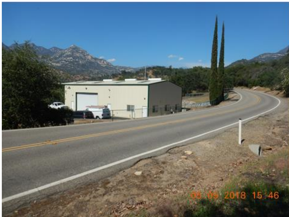
Photo A-7. New maintenance building at the Kaweah No. 1 Powerhouse Campus as seen from Highway 198. Camera facing northeast. May 9, 2018.
