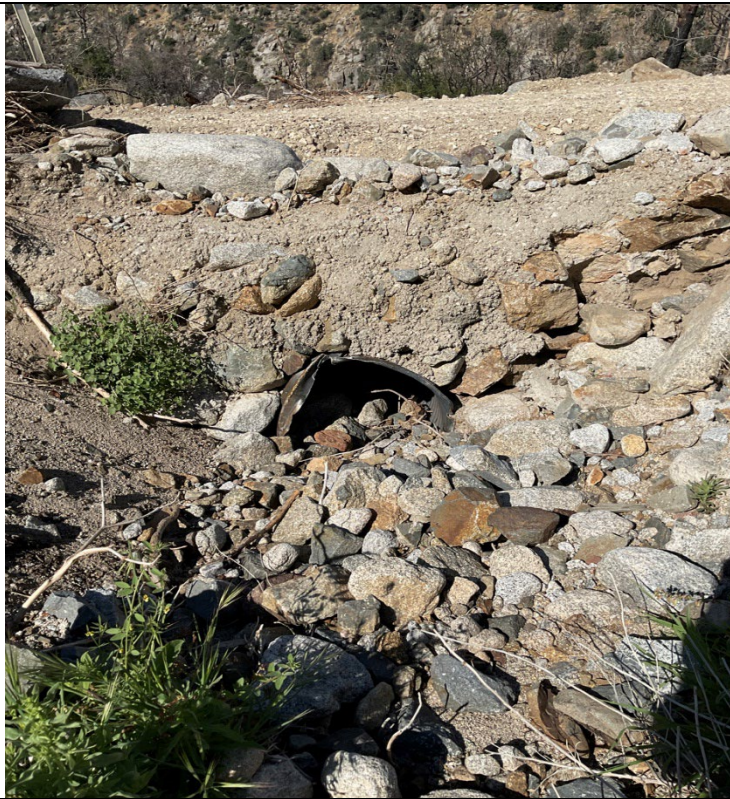
Photograph: 7 Example of culvert categorized as “Potential Concern”, due to blockage inlet side, facing north.
