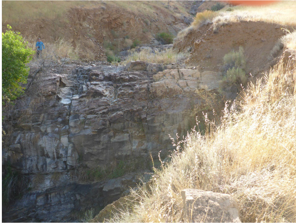
Figure A-59. Second knickpoint in KR3 Powerhouse Forebay Spillway channel.
