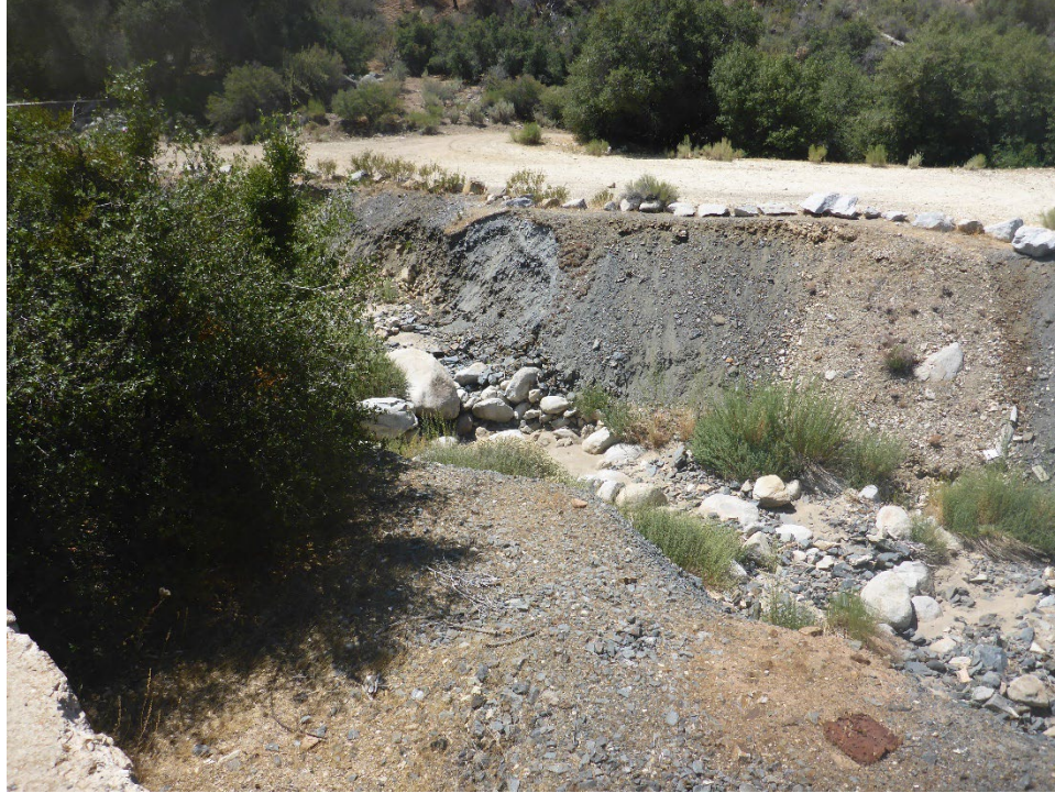
Figure A-49. Additional view of moderate erosion along left bank (south side) of Corral South Tunnel 18 Spoil Site (view immediately adjacent to left of Figure A-48 image).
