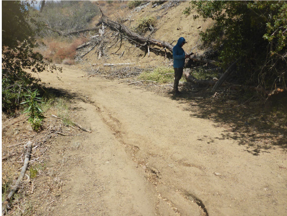
Figure A-29. Minor rilling cut into road surface at Tunnel 10 Spoil Site.
