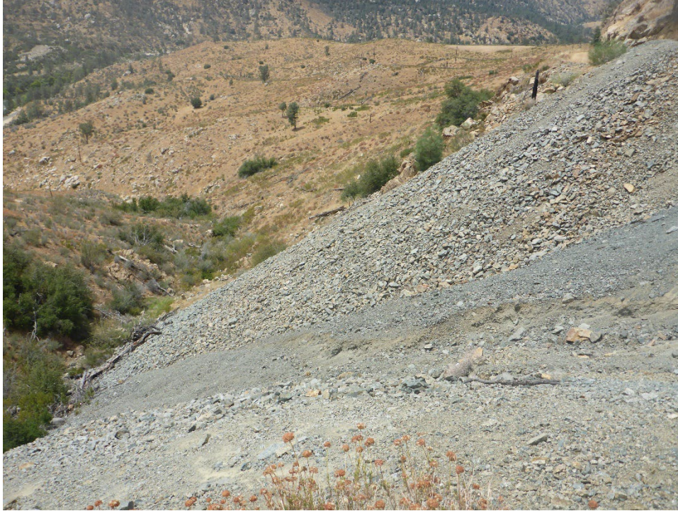
Figure A-37. Close-up view of erosion into Tunnel 14 spoil material.
