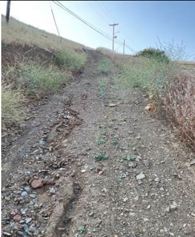
Photograph: 5 Example of road in “Fair Condition. Note the rills and some overgrown vegetation. North Penstocks Access Road, facing east.
