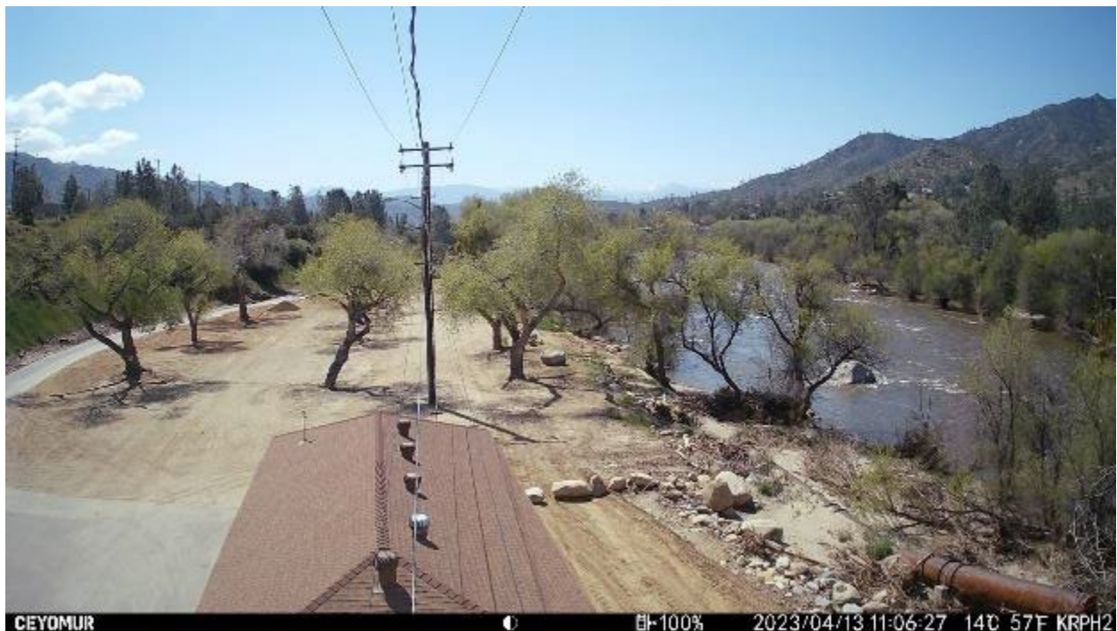
KRP12 facing downstream towards WHITEWATER parking area
