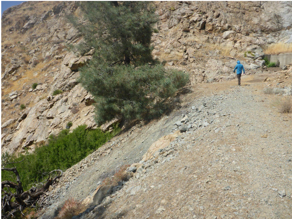
Figure A-38. Tunnel 15 Spoil Site (view looking upslope from access road).
