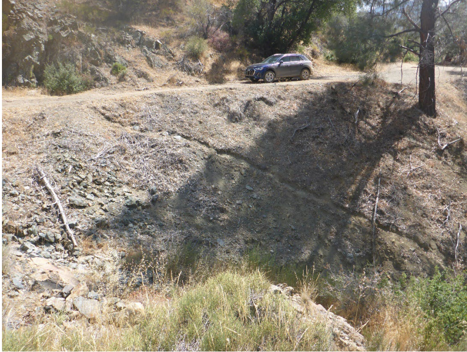
Figure A-41. Spoil material and access road at Tunnel 16/17 Spoil Site (view from immediately adjacent to right side of Figure A-40).
