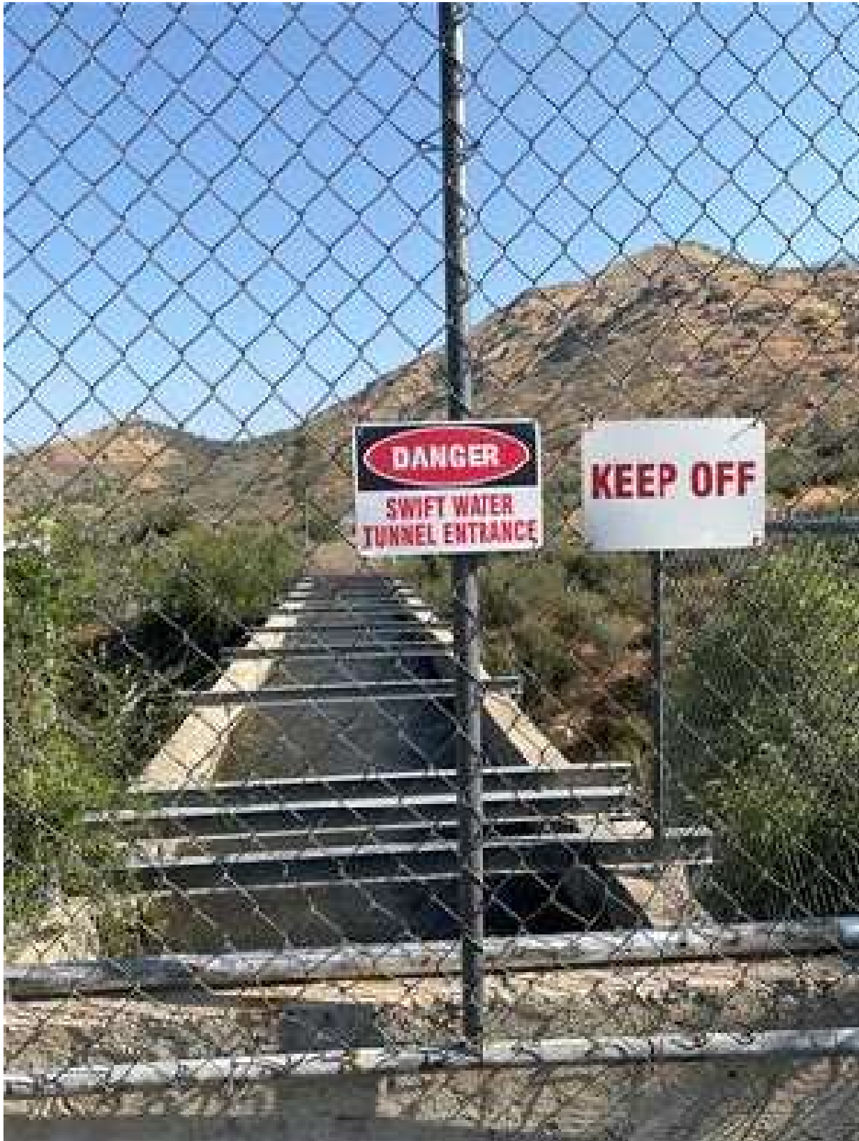
Tunnel at 18 Corral Creek Access (002).jpg
