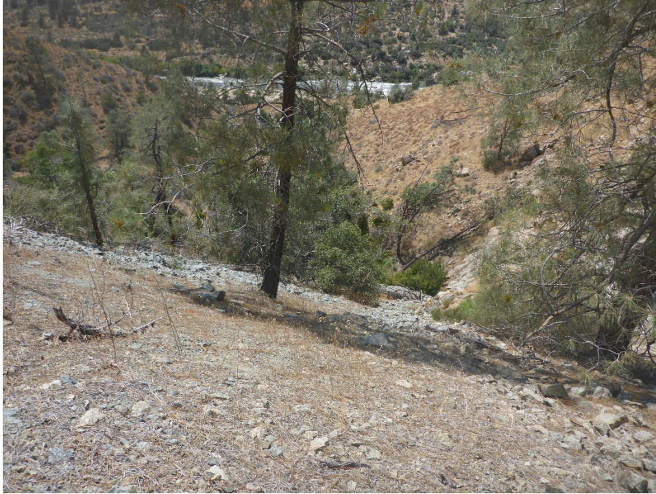
Figure A-39. Stable outboard edge of Tunnel 15 spoil pile with little-to-no active erosion; Kern River visible in background (view looking downslope).
