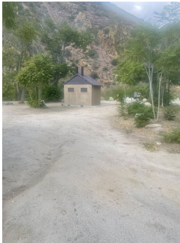
Photo C-5. Road's End Entrance and Restroom Access
