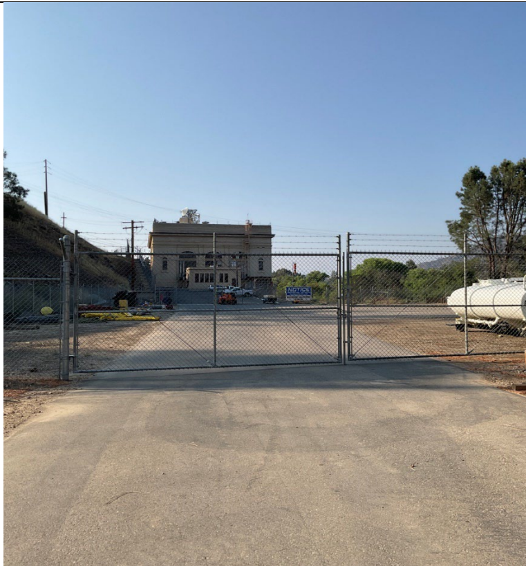
Photograph: 15 Example of gated SCE Project Road, restricting public access. All SCE gates were locked and in good working condition.
