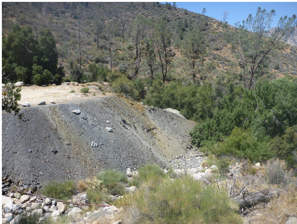
Figure A-48. Moderate erosion of left bank (south side) of Corral South Tunnel 18 Spoil Site; sediment delivered directly to the watercourse.
