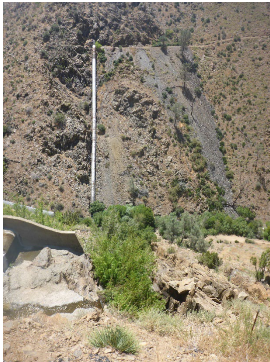
Figure A-54. Cannel Creek Siphon Spillway (view looking downslope).
