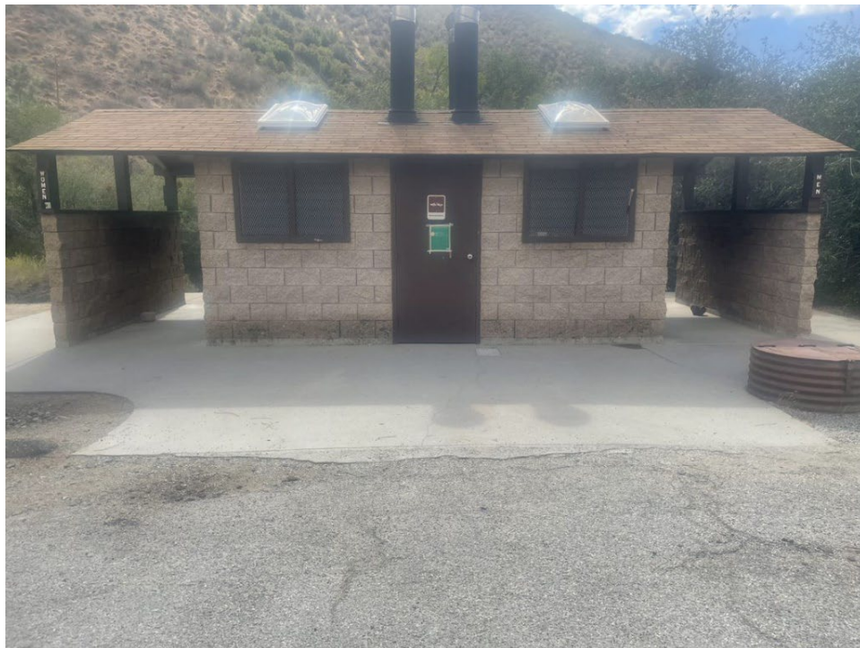
Photo C-8. Restrooms at Fairview Campground
