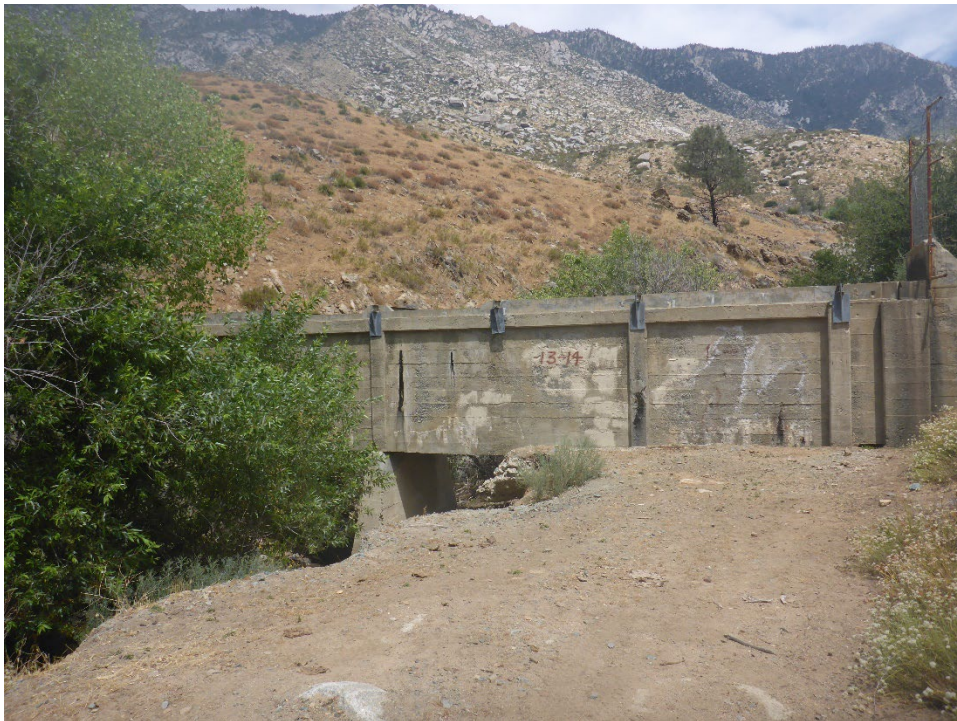
Figure A-34. Access road built on Tunnel 13/14 Spoil Site at Gold Ledge Creek (view looking upstream and showing left bank [south side] of spoil material).
