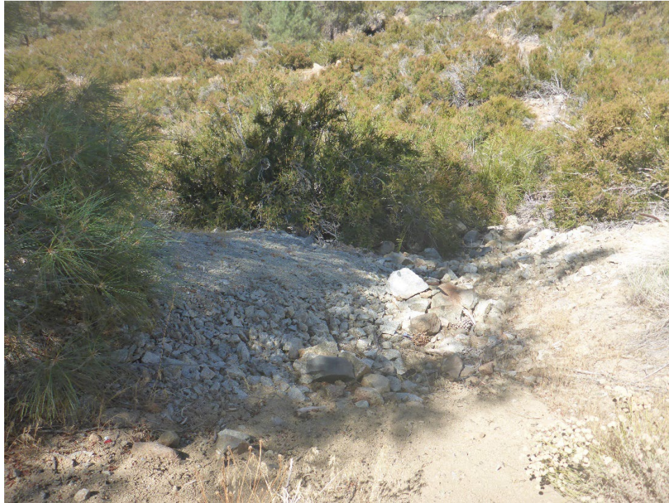
Figure A-17. Downslope margin of tunnel 8B spoil pile.
