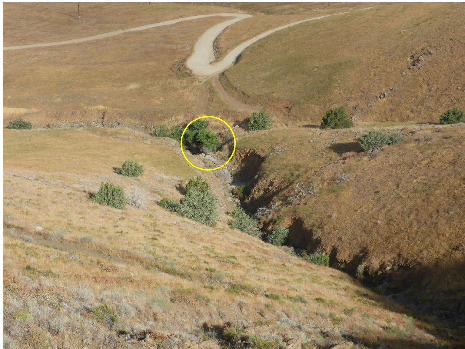
Figure A-60. Top of KR3 Powerhouse Forebay Spillway channel (looking downstream; location of knickpoint in Figure A-59 image indicated by yellow circle).
