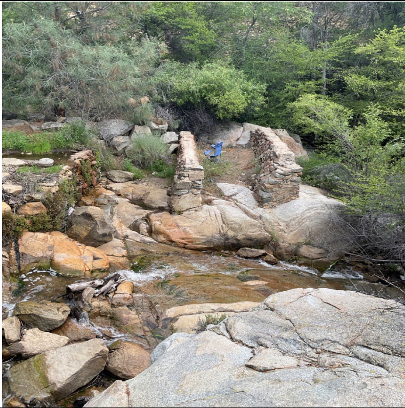
Photograph: 11 Where bridge used to be, Tunnel 8A/8B Flume Access Road, facing south. There are little erosion concerns as stream banks are protected by boulders and vegetation, dissipating the water's energy.
