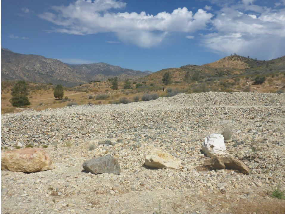
Figure A-43. Coarse spoil material at Corral North Tunnel 17 Spoil Site, located at head of broad, low-gradient upland valley swale, little-to-no active erosion.
