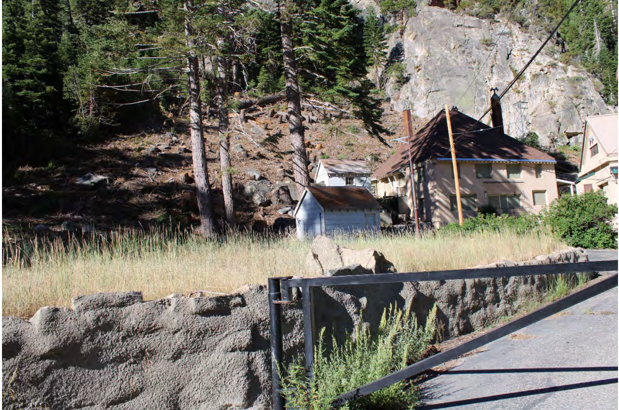
KOP 7, Upper view, looking Southwest
