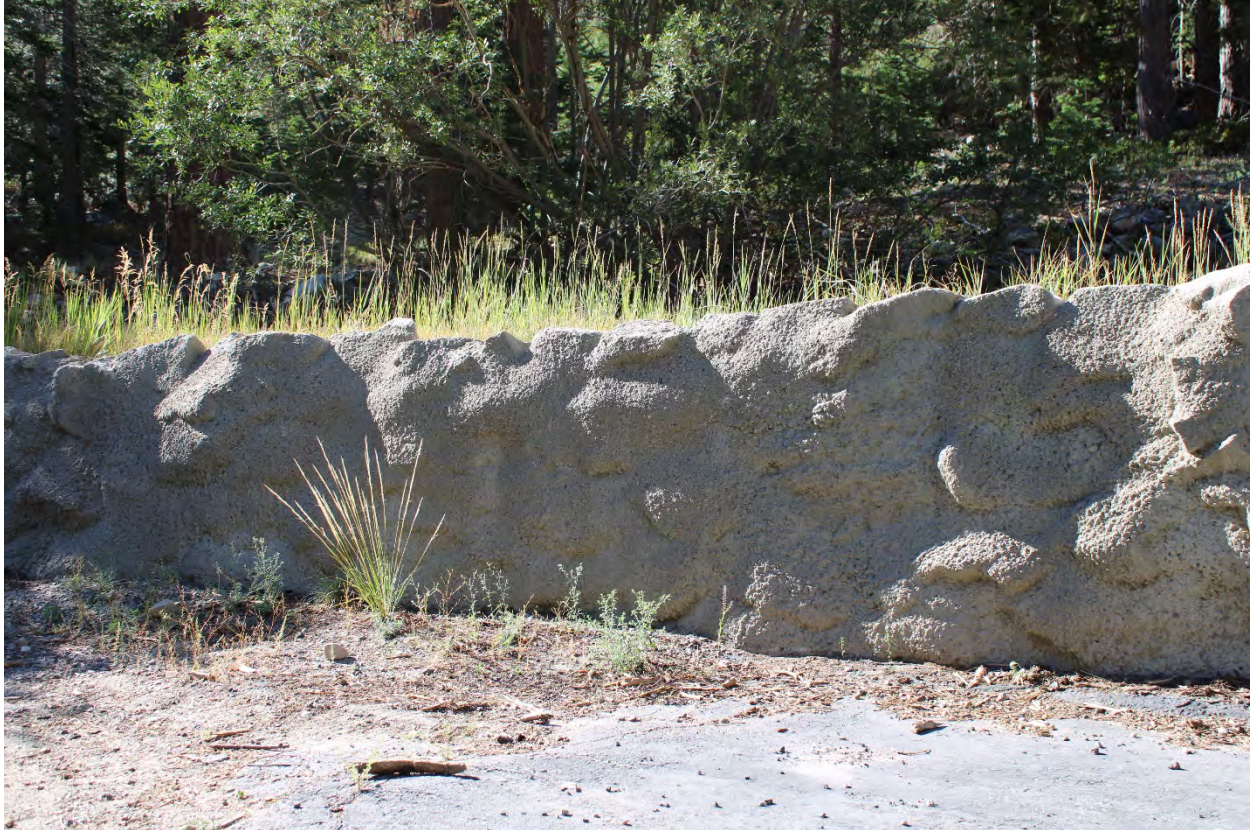
KOP 7, Lower view, looking Southeast
