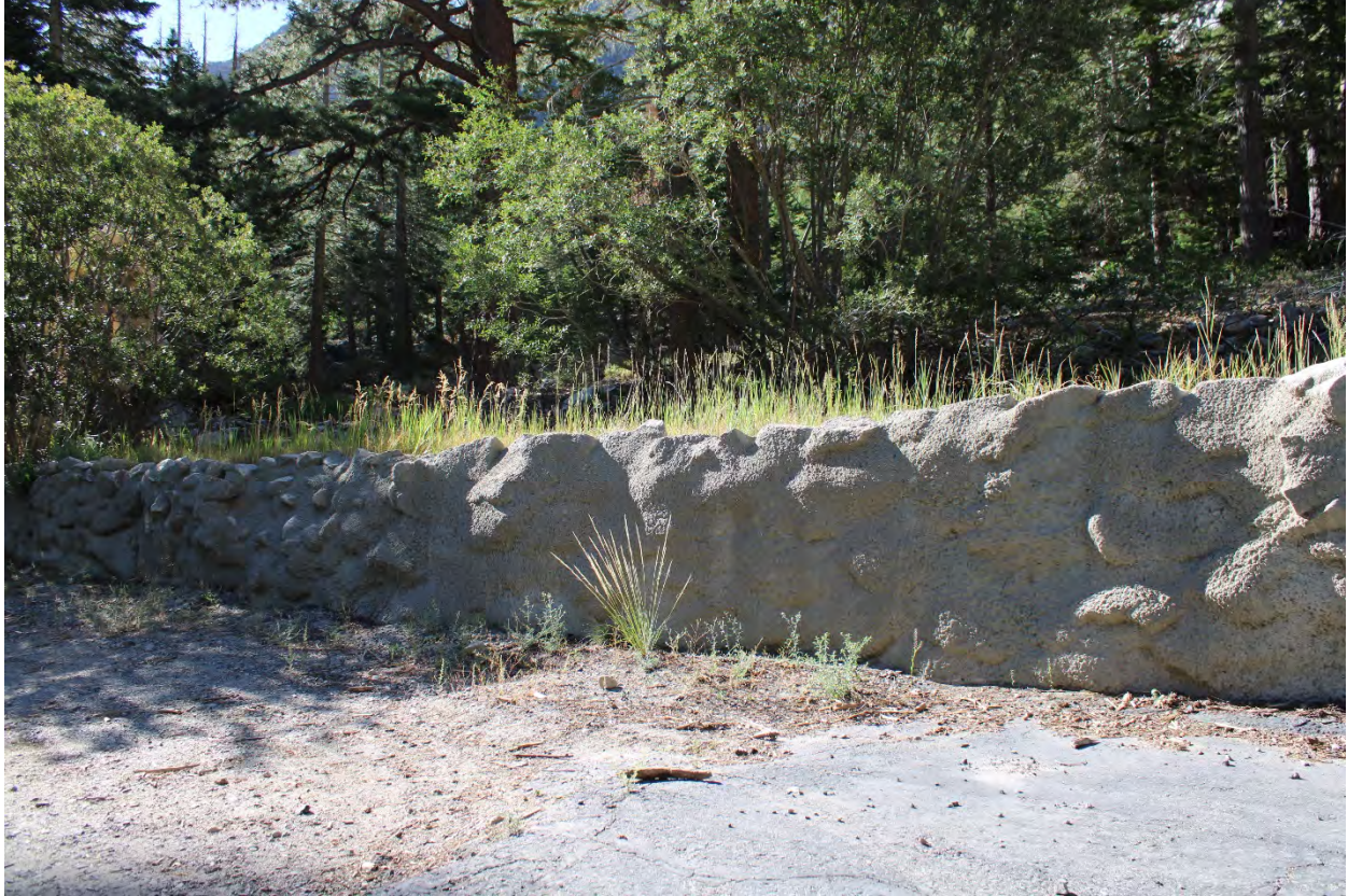
KOP 7, Middle view, looking Southeast
