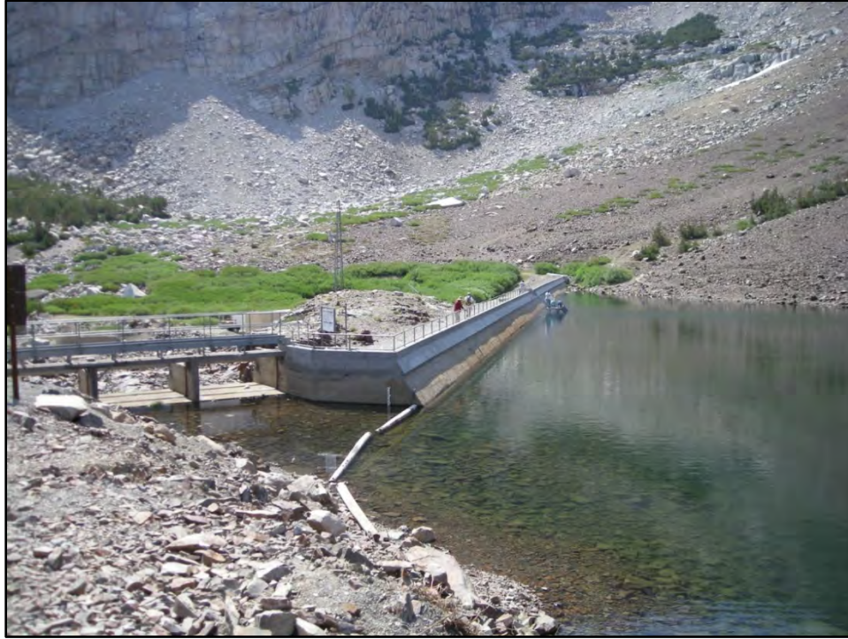
Photo 5. Rhinedollar Dam (Ellery Lake) and Spillway.
