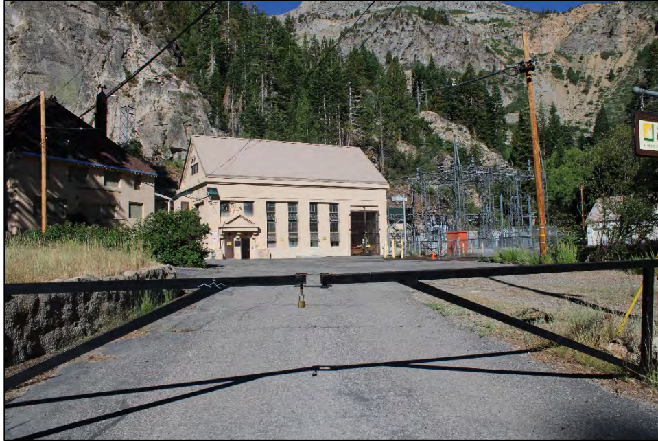
Photo 66. KOP 7 Poole Powerhouse Gate View West.
