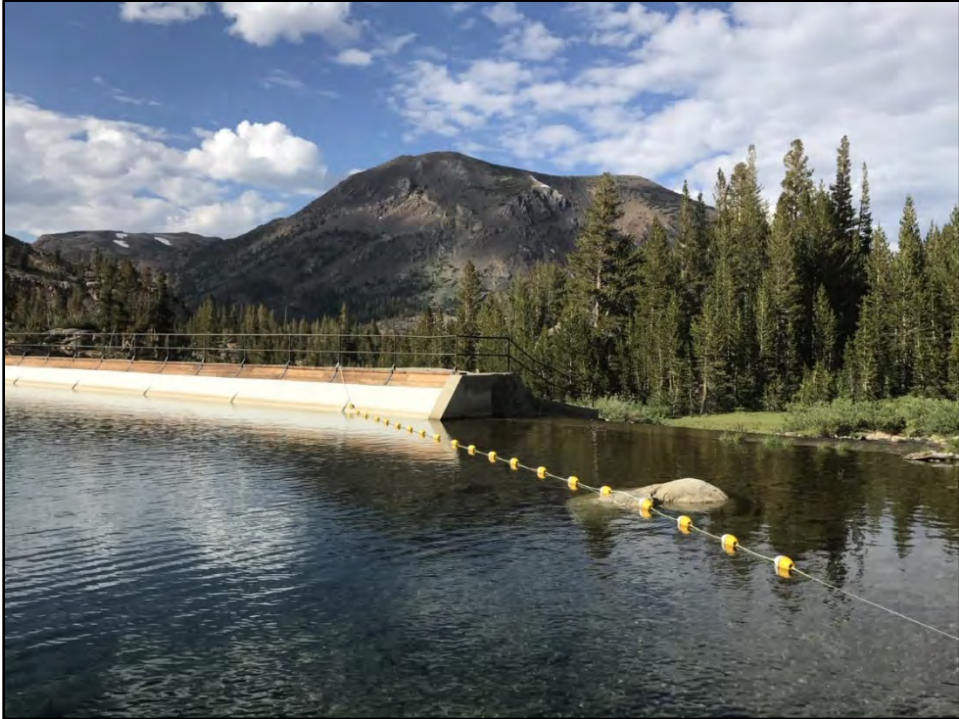
Photo 3. Tioga Dam and Spillway.
