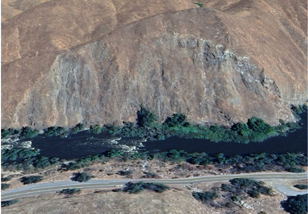
Photo A-15. Rilling/Landslide RB-1 (Google Earth Image, Date: 8/24/23)
