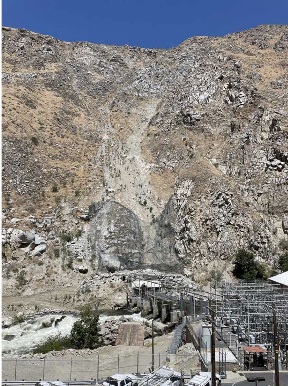
Photo A-17. Natural Rockslide at KR1 Powerhouse
