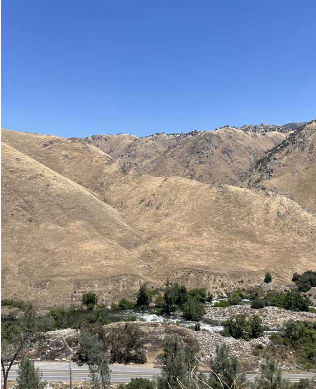
Photo A-11. Bank Erosion RB_1
