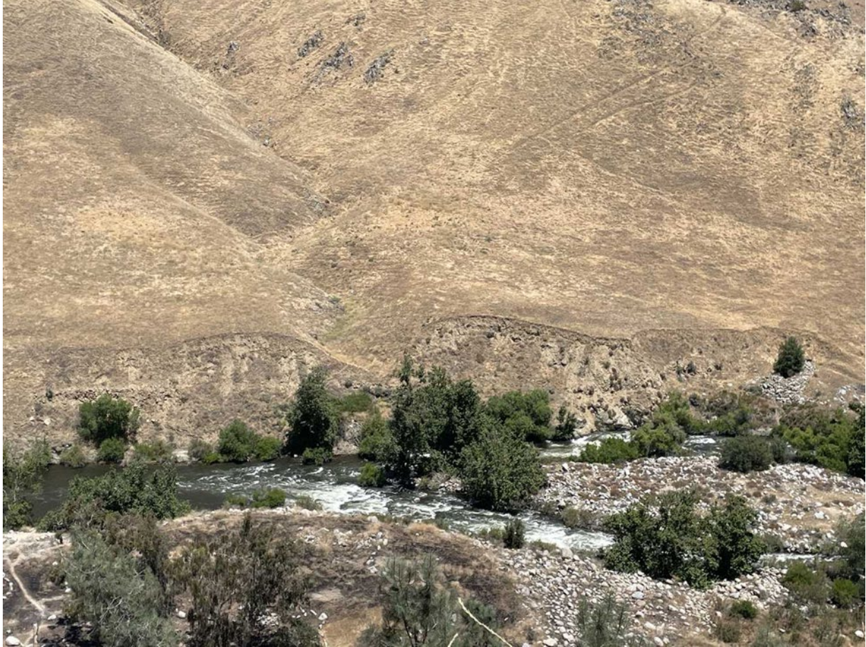
Photo A-10. Bank Erosion RB_1
