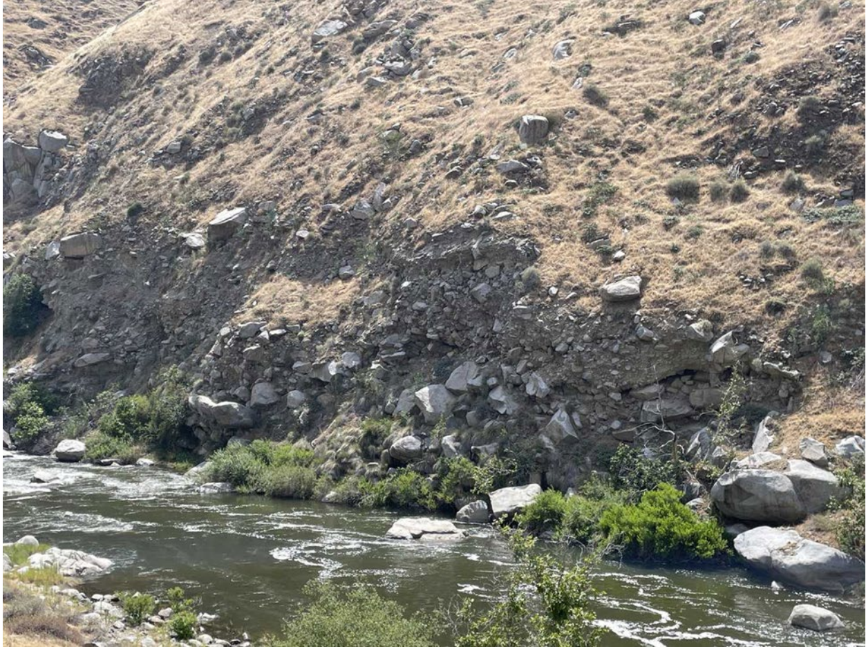
Photo A-16. Bank Erosion RB-2
