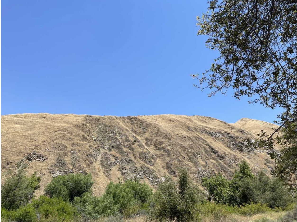
Photo A-14. Rilling/Landslide RB-1
