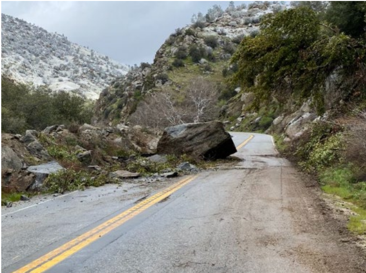
Photo A-23. Debris Slide Closing SR-178 on March 1, 2023 (Caltrans 2023)
