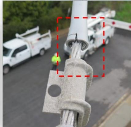
3b. SCE's Distribution Overhead Detail Inspection program includes questions related to the condition of primary conductor, including covered conductor. As part of that program, inspectors look for conditions such as corrosion (please refer to the sample question below). If any damage is observed, it is reported for remediation. Inspectors visually inspect from the ground, with the assistance of binoculars, handheld cameras and drones for closer review of primary cable.
