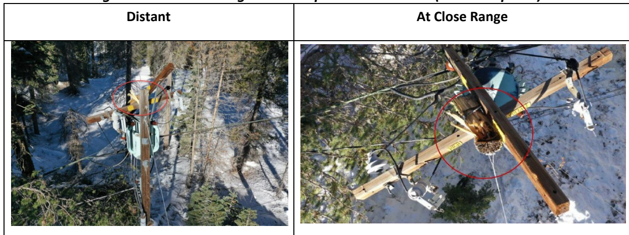
Figure SCE 8-19 Damaged Pole Top on a 4kV Circuit (Drone Capture)
