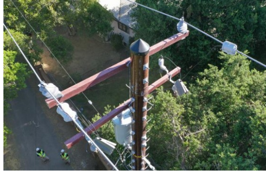
Figure SCE 8-06 Dead-end Structure (left) and Tangent Structure (right)
