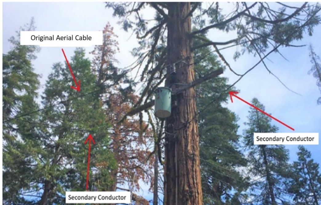
Figure SCE 8-05 An Example of a Tree Attachment Where Electrical Equipment Was Attached to a Live Tree
