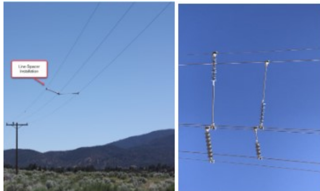
Figure SCE 8-08 A Line Spacer Installed on a Long Span to Mitigate Wire-to-Wire Contact (Left), Close Up Line Spacer View (Right)
