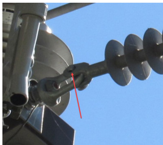
Figure 3: Example of Missing Cotter Key (Primary)
