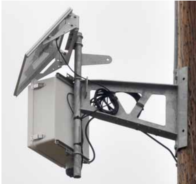
Figure AP 810-5: Typical Installation of Weather Monitoring System (NEMA Enclosure and Solar Panel) — FRO
