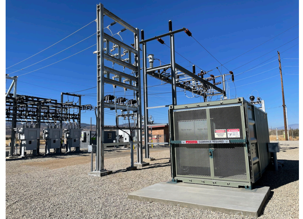
REFCL equipment installed at an SCE substation
