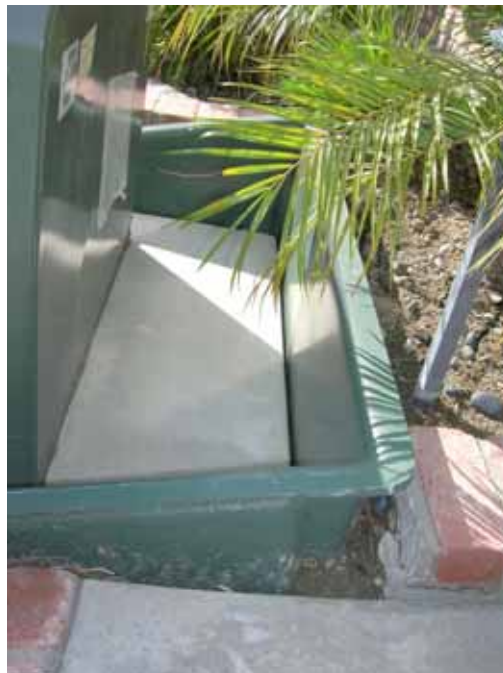
Figure SS 600–3: Side View of an Example Installation of a Protection Wall
