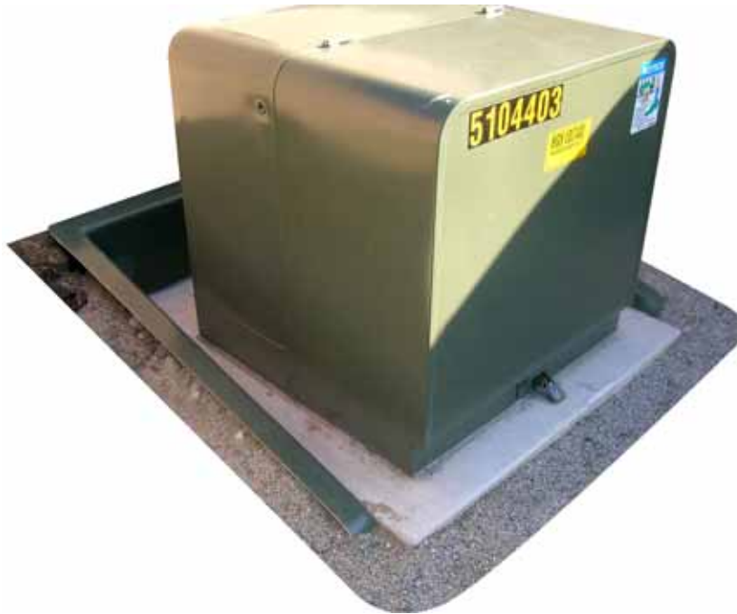
Figure SS 600–3: Side View of an Example Installation of a Protection Wall
