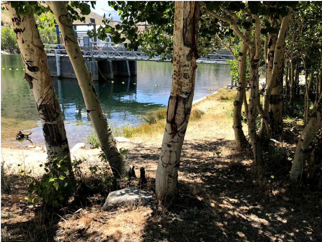
Photo 96 Access Behind Intake
