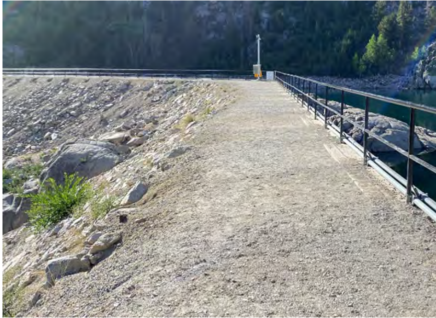
Photo 10 Crest of Sabrina Dam
