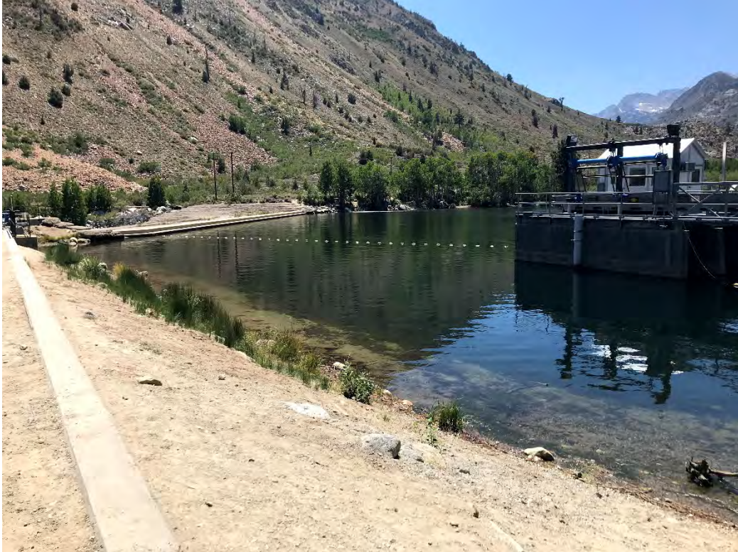
Photo 97 Access Along Intake No. 2 Dam
