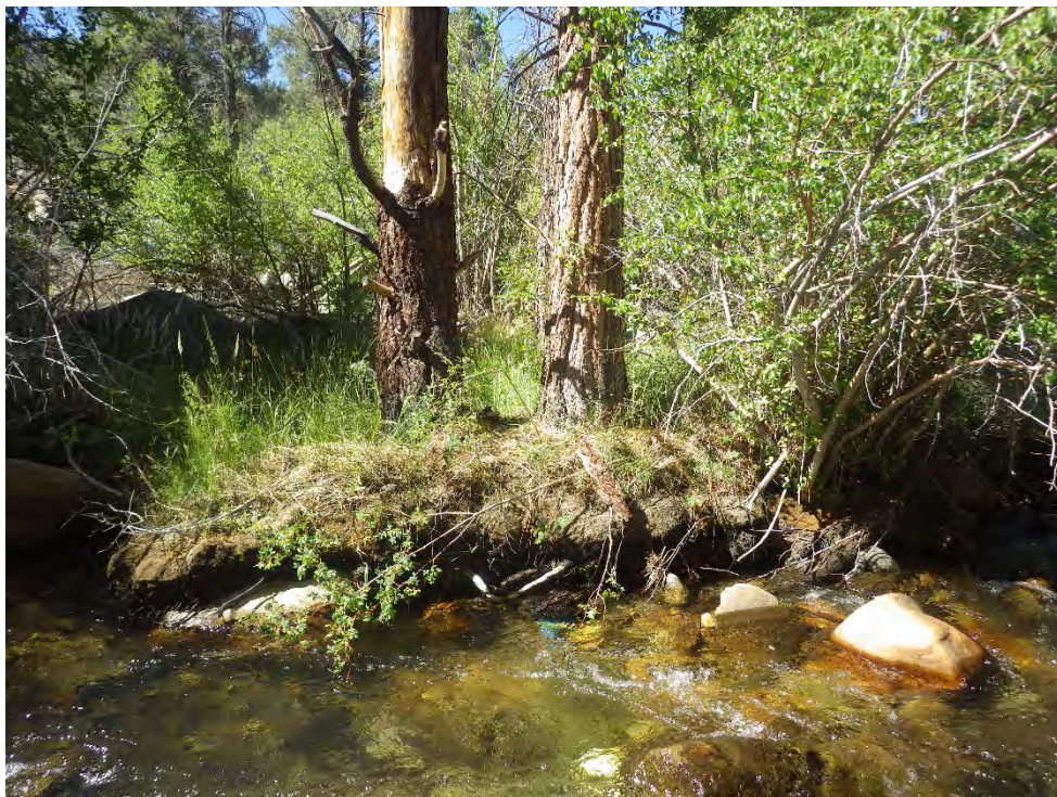
Figure A-32. Cross section 4.4 in August 2020, view of right bank from left bank.
