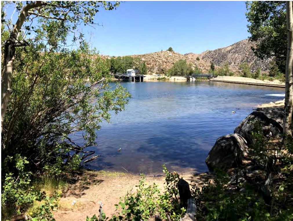
Photo 111 Access to Shoreline
