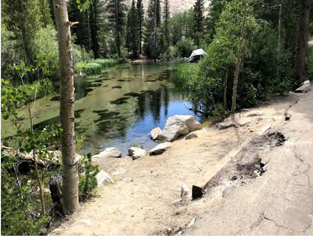
Photo 16 Access to Shoreline Upstream of Bridge
