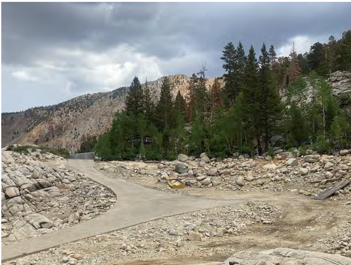
Photo 42 End of New Paving at South Lake Boat Ramp
