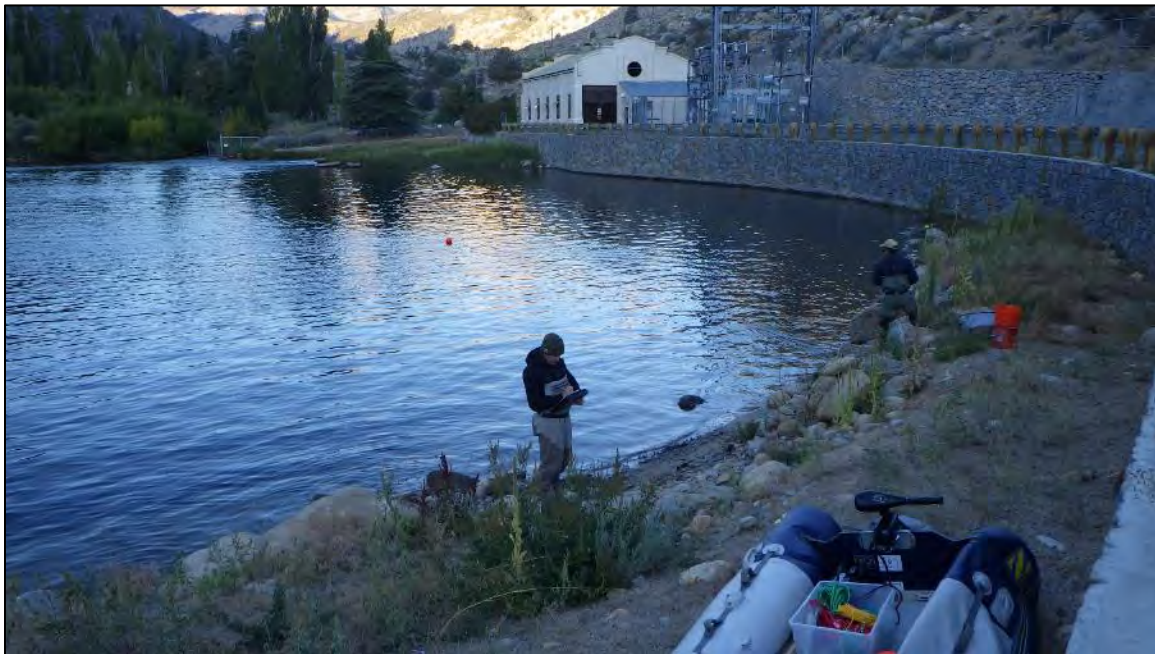
Figure A-37. Intake 4 overview photo. September 24, 2019.
