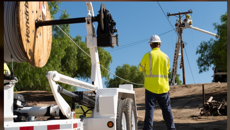
Above photos: SCE crew installing insulated wire
