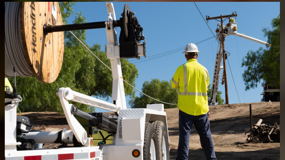
Above photos: SCE crew installing insulated wire
