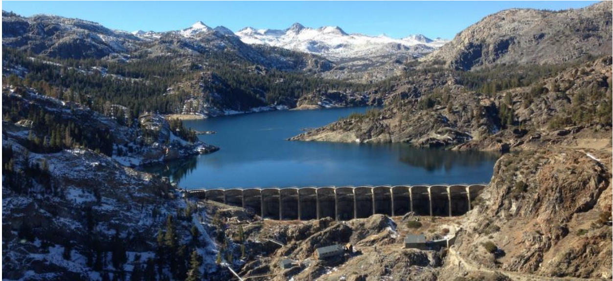
Photo A-3. Gem Dam, Gem Lake, and Ancillary Facilities below Dam, High Water Level (looking west)
