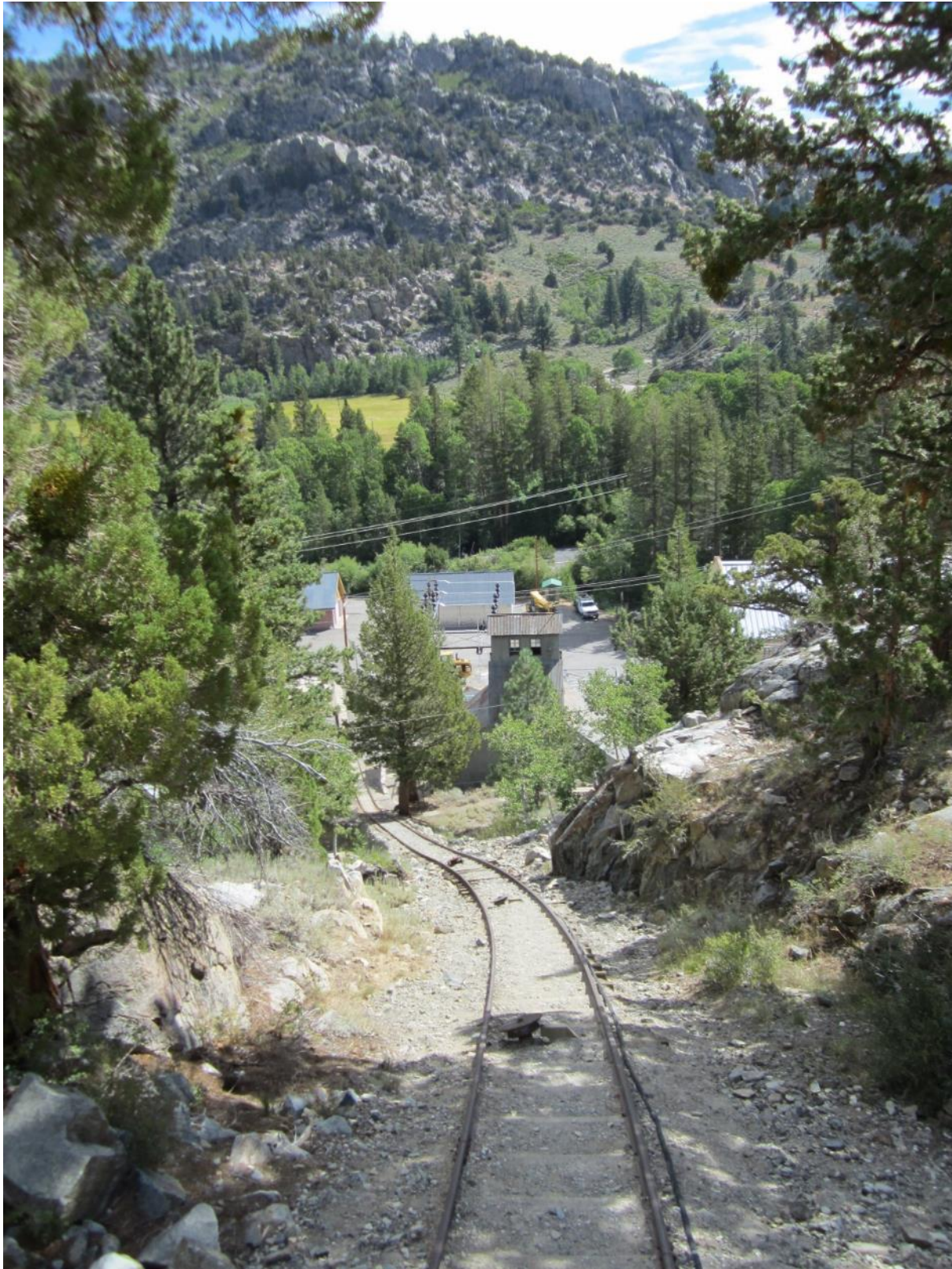
Photo A-8. Agnew Tram Tracks and Rush Creek Powerhouse Complex in the Distance (looking east)
