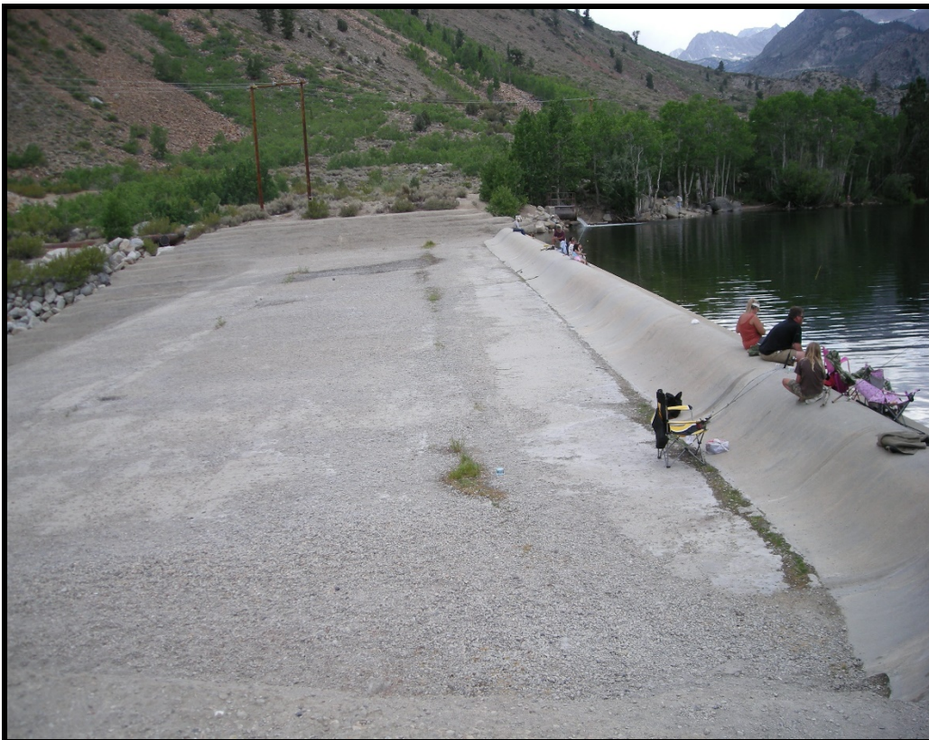
FIGURE 4-41 INTAKE NO. 2 DAM
