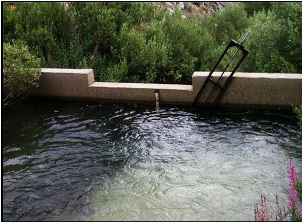
FIGURE 4-43 MCGEE CREEK DIVERSION
