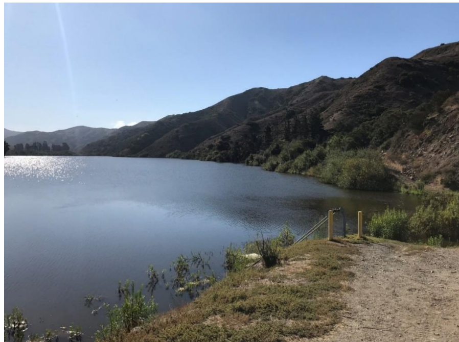
Figure 4-5 - Middle Ranch Reservoir
