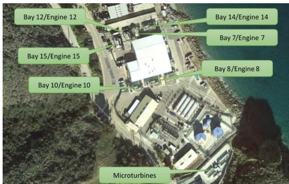
Figure 3-5 - Engine Bays and Engines
