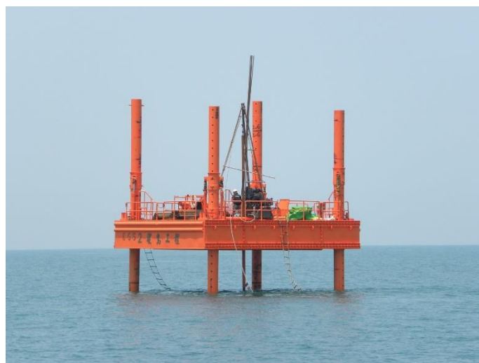
Figure 5-14 - Subsea Soil Sampling (EGS Survey)
