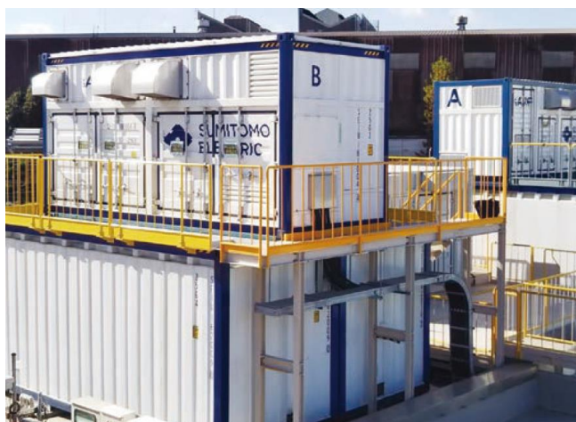
Figure 4-16 - Sumitomo Electric Industries, Inc. Vanadium Redox Flow Battery
