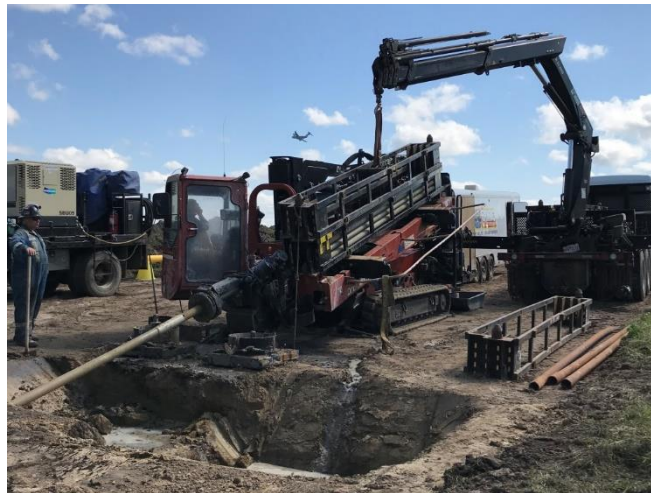
Figure 5-16 - HDD Rig and Sending Pit
