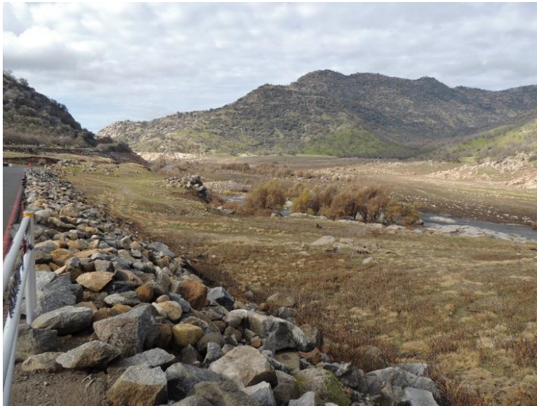
Photo B-36. Slick Rock Recreation Area, Lake/River Access
