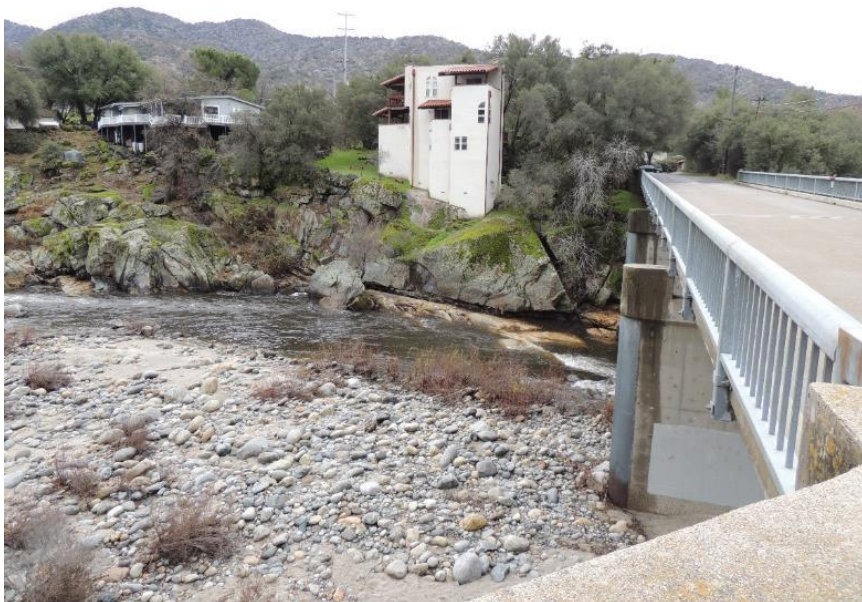
Photo B-18. Dinely Bridge, Upstream Right
