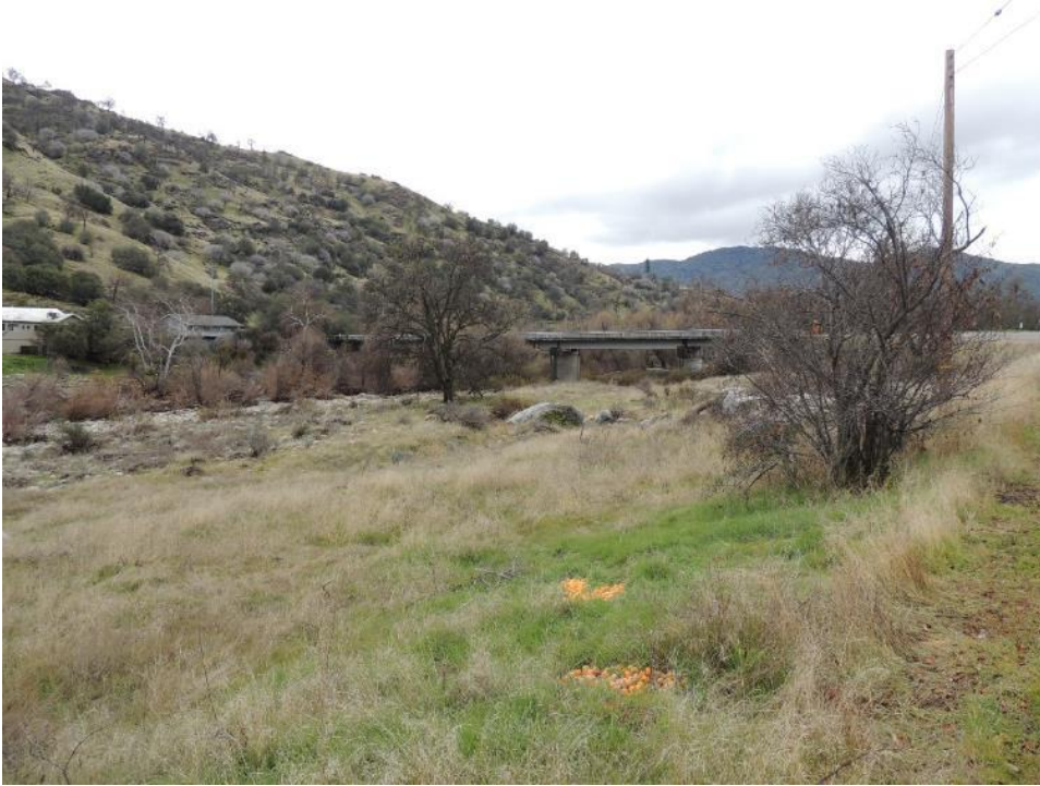
Photo B-34. North Fork Road, Upstream of Bridge
