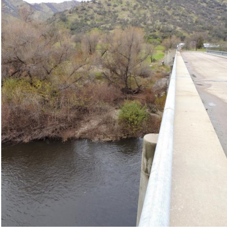
Photo B-32. North Fork Bridge, Downstream Left
