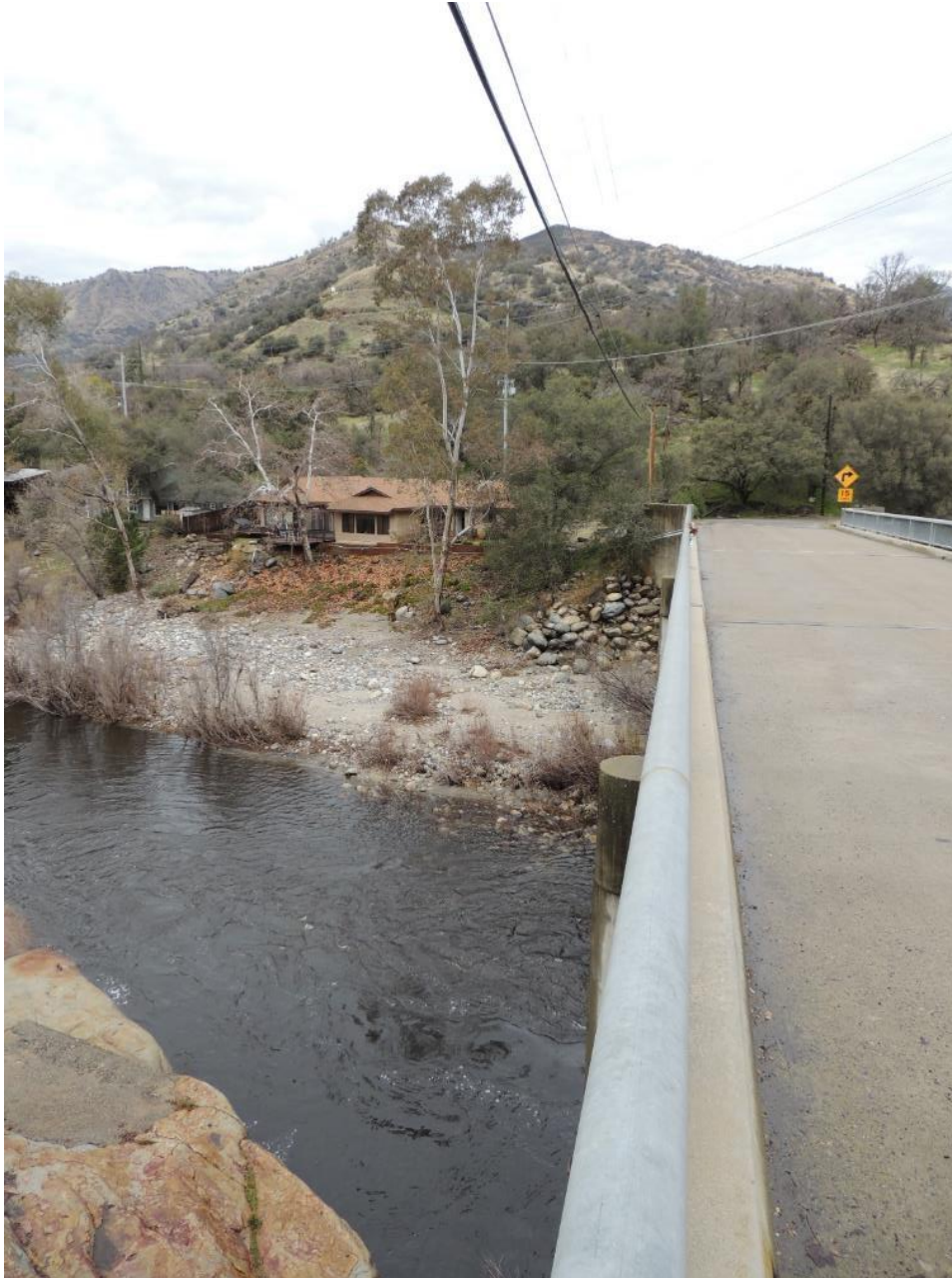
Photo B-19. Dinely Bridge, Downstream Left
