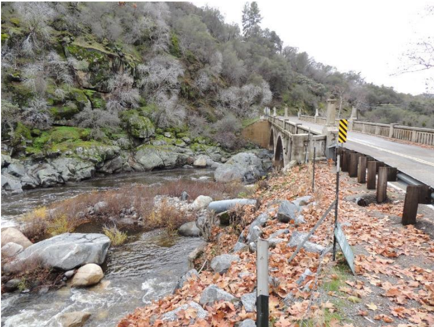
Photo B-8. Gateway Bridge, Upstream Right
