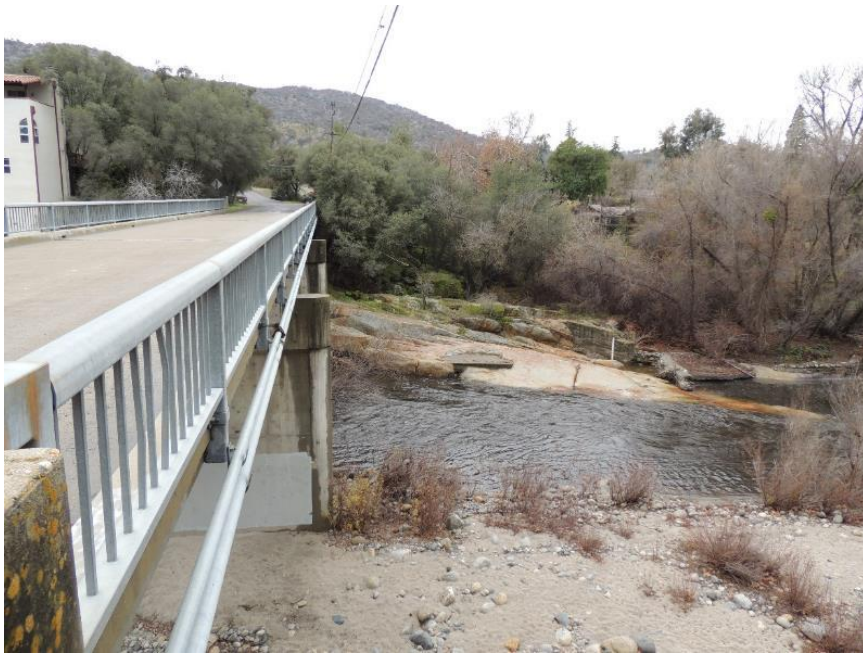
Photo B-20. Dinely Bridge, Downstream Right
