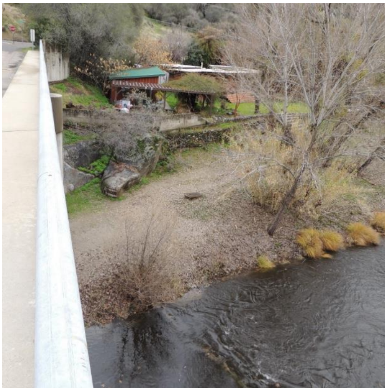
Photo B-33. North Fork Bridge, Downstream Right
