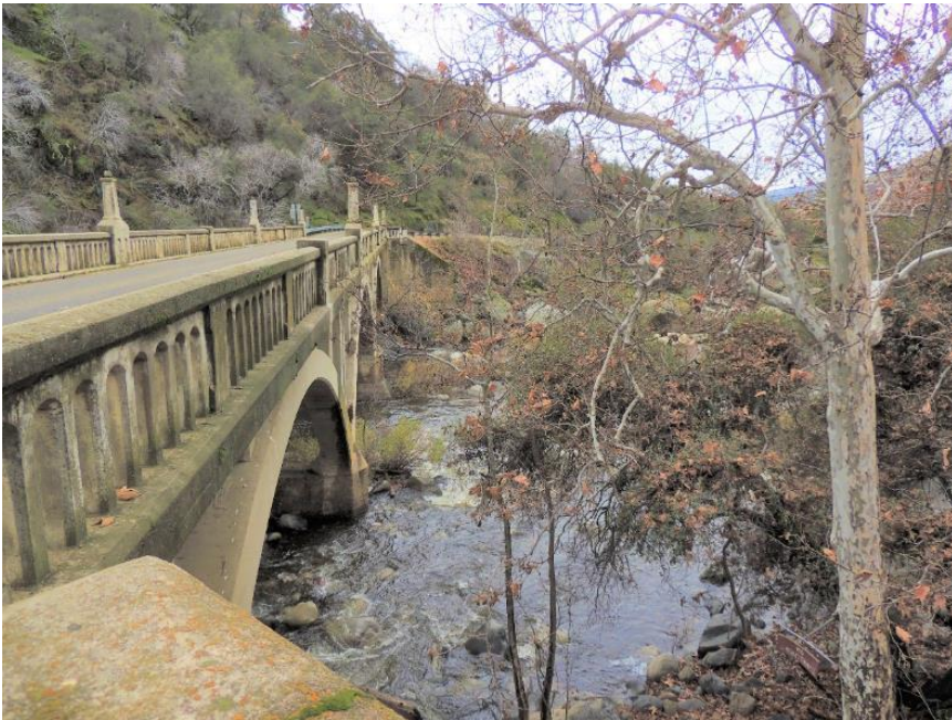
Photo B-10. Gateway Bridge, Downstream Right
