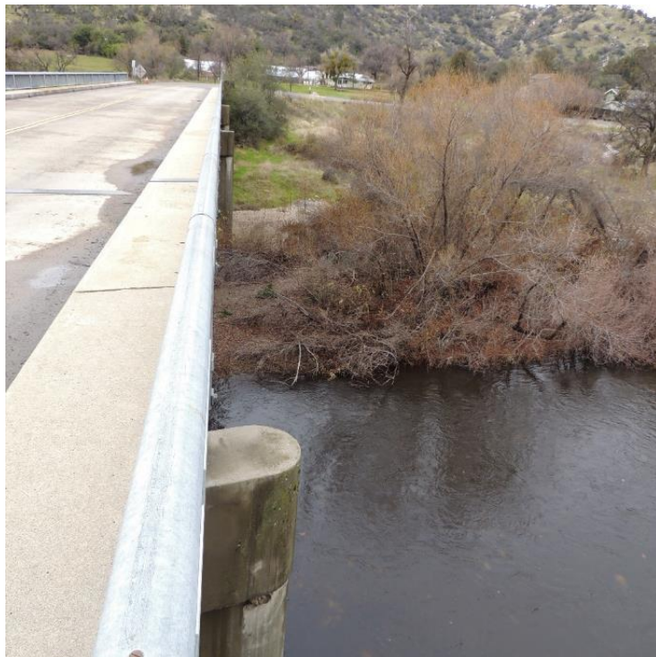
Photo B-30. North Fork Bridge, Upstream Left
