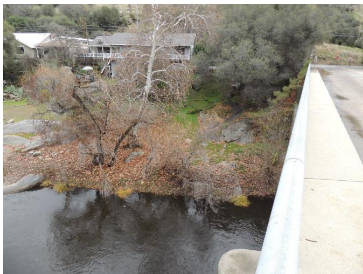
Photo B-31. North Fork Bridge, Upstream Right
