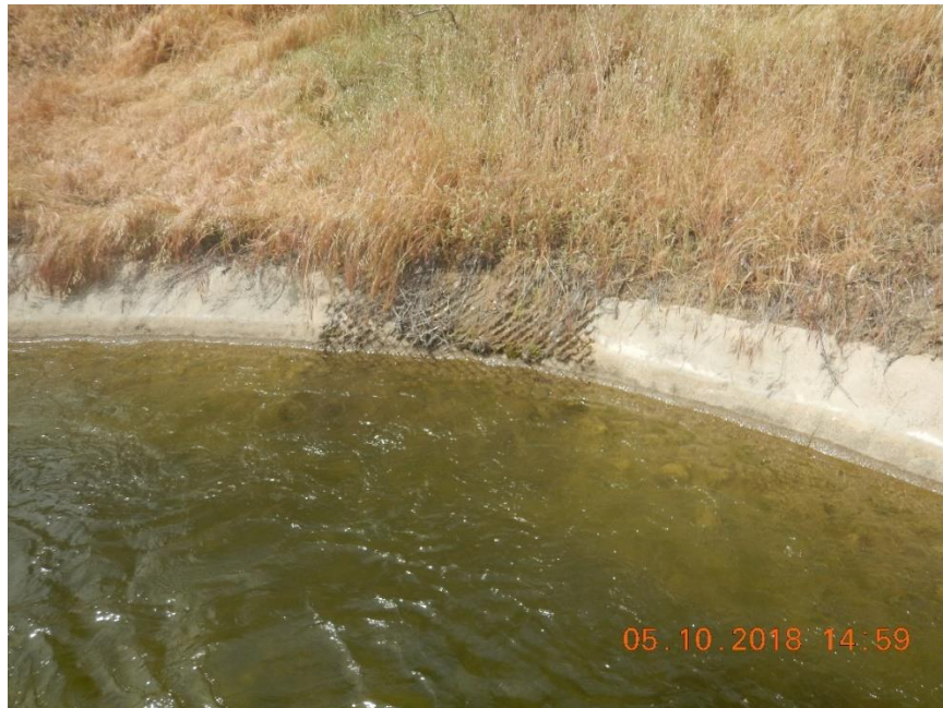
Photo B-7. Kaweah No. 2 Flowline, escape fencing, fair condition (May 10, 2018). [#1517]
