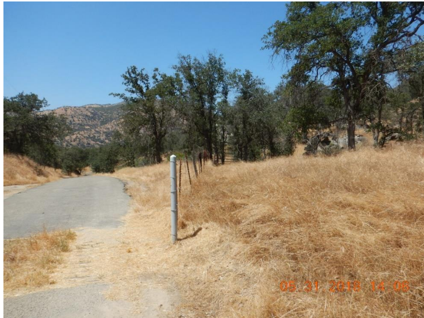
Photo B-14. Kaweah No. 1 Forebay Road, cattle guard, poor condition (May 31, 2018). [#1577]
