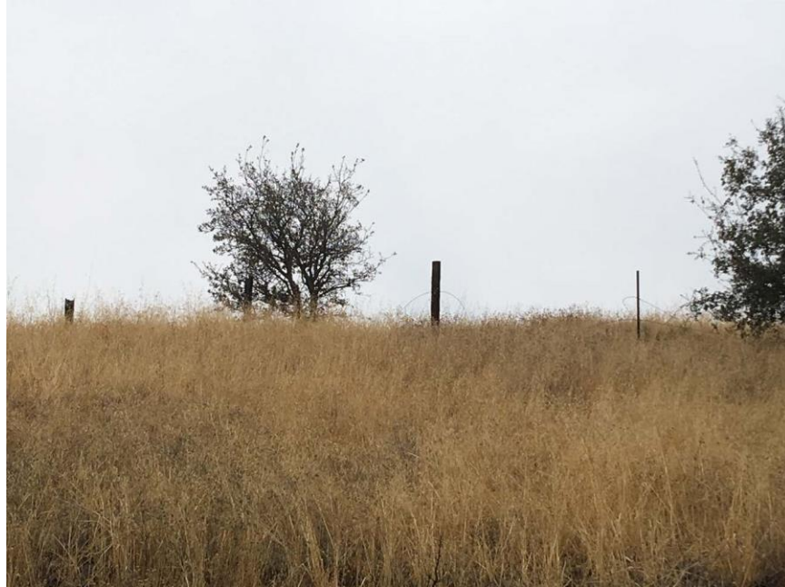
Photo B-13. Kaweah No. 2 Flowline, fence in poor condition November 11, 2018). [#111118]
