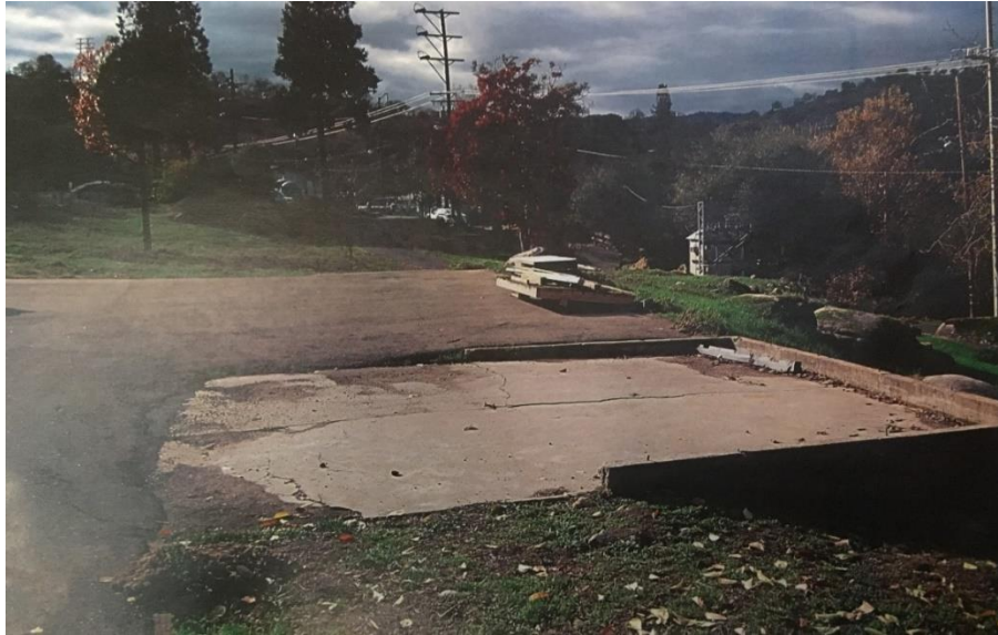
Photo B-1. Area within the Kaweah No. 1 Powerhouse Campus before the maintenance building was constructed in 2012. View is looking east from within the campus. Date unknown.
