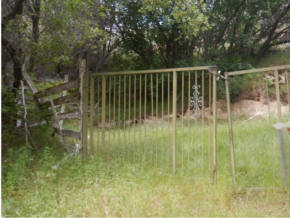
Photo D-13. Kaweah No. 1 Flowline Access Road – Unnamed, road start and gate, poor condition, May 8, 2018
