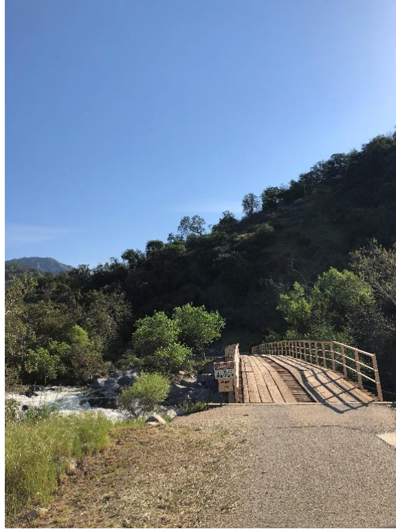
Photo D-5. Kaweah No. 3 Powerhouse Road, bridge, good condition, April 24, 2018
