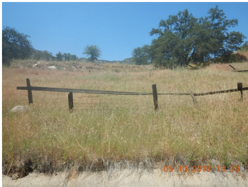
Photo B-12. Kaweah No. 2 Flowline, fence in fair condition (May 10, 2018). [#1509]
