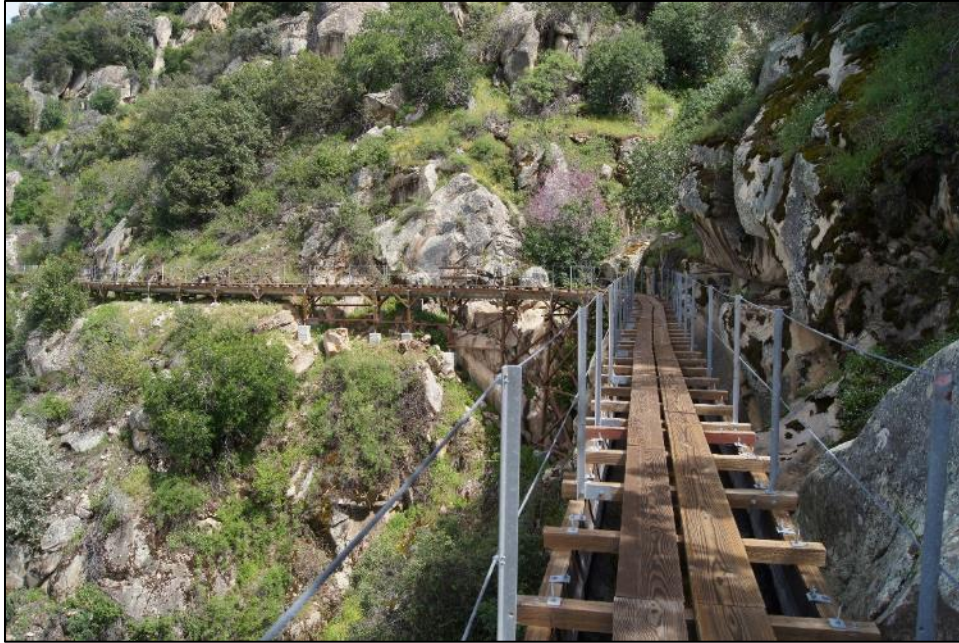
Photograph 4. Kaweah No. 1 Flowline traversing the steep hillside, camera facing east. April 18, 2018.
