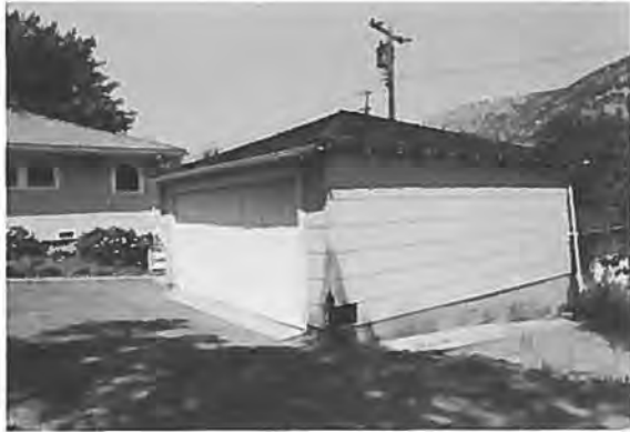
Bldg. 0123, Garage Kaweah Powerhouse No. 1 View to W Roll 1, Frame 21, 6-27-89
