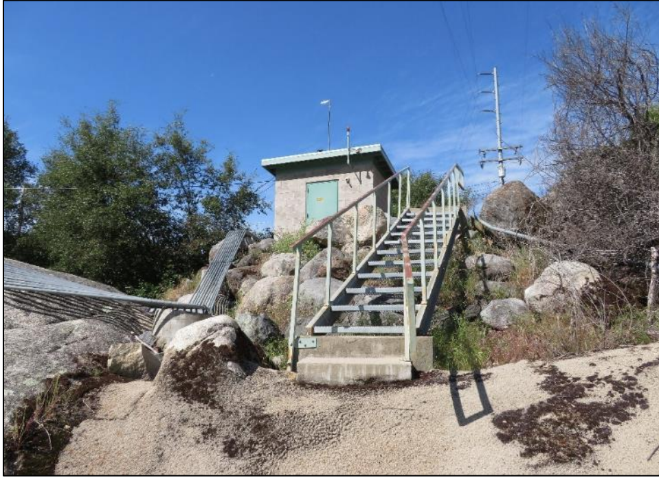
Photograph 4. Control Building. Camera facing north. April 18, 2018.
