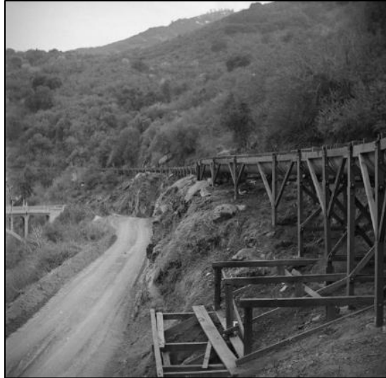
Figure 3. Kaweah No. 1 Flowline at Kaweah River Bridge following reconstruction, note metal flume, 1948 (Huntington Library, Call Number 02 - 26553).
