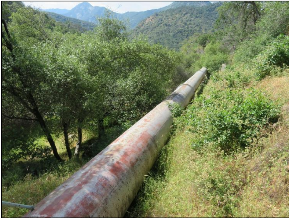
Photograph 10. Siphon pipe, camera facing southwest. May 8, 2018.
