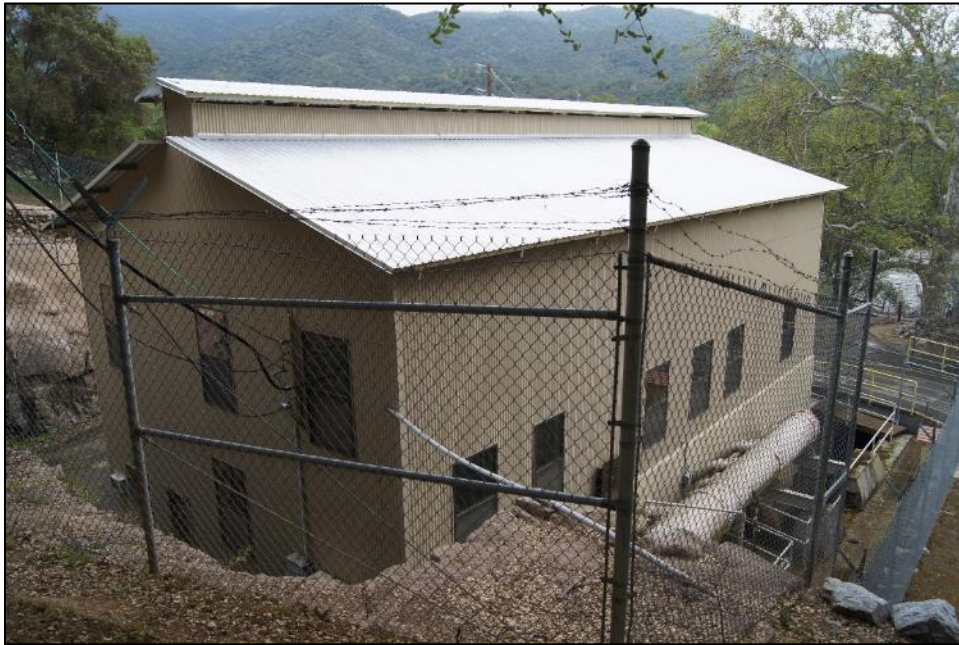
Photograph 4. Kaweah Powerhouse No. 2, camera facing west. April 19, 2018.
