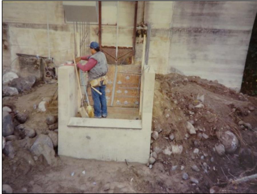
Photograph 6. Concrete tailrace channel under construction, 1991 (SCE).
