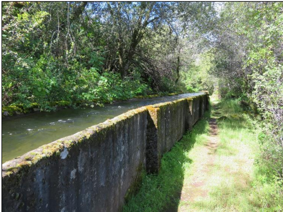
Photograph 3. Middle Fork Flowline, camera facing southwest. April 17, 2018.
