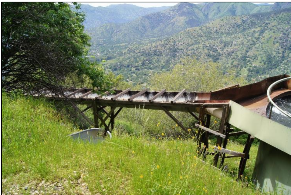
Photograph 4. Spillway chute, camera facing west. April 18, 2018.
