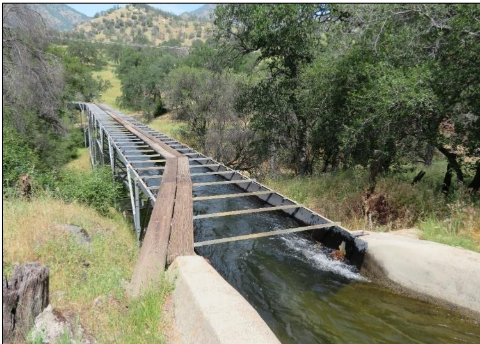
Photograph 3. Flume span along Kaweah No. 2 Flowline, camera facing northwest. May 8, 2018.
