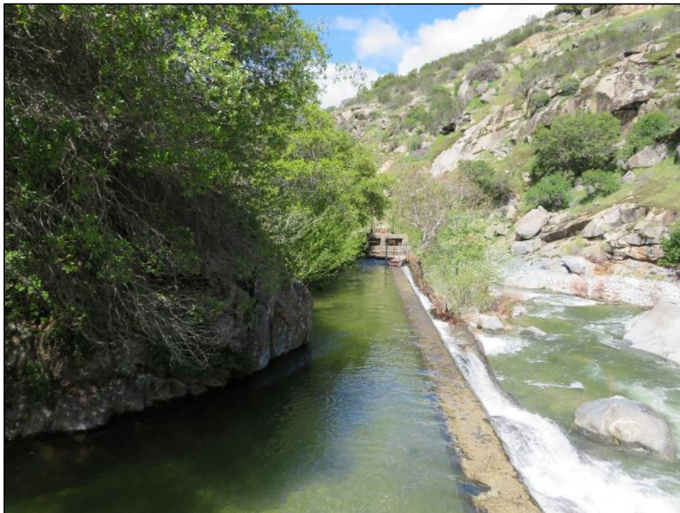
Photograph 3. Concrete sandbox, camera facing west. April 17, 2018.
