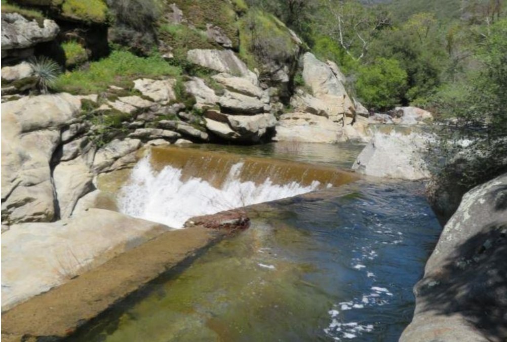
Figure CUL 5-51 Marble Fork Diversion Dam, camera facing north
