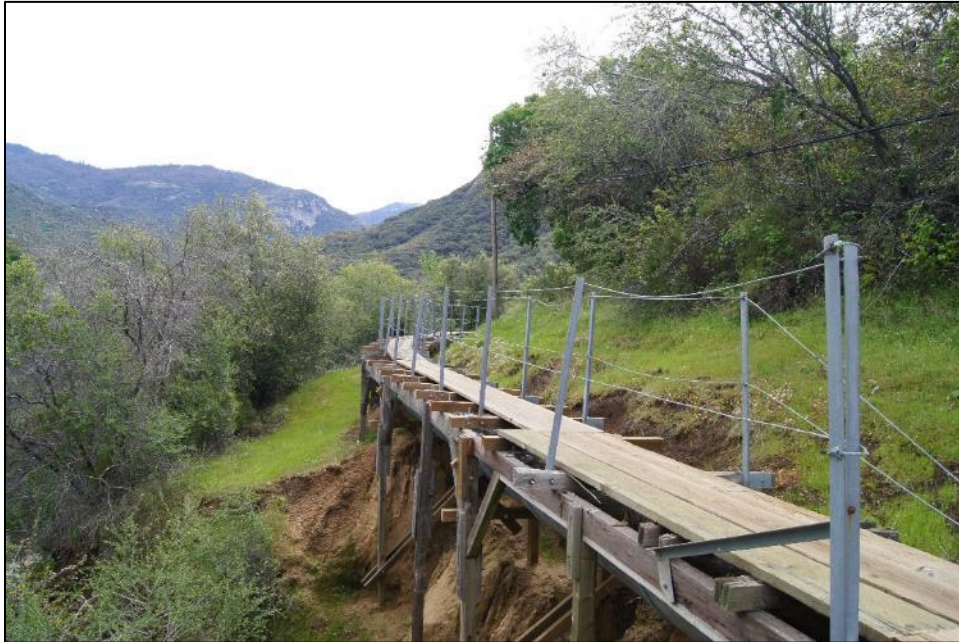
Photograph 2. Kaweah No. 1 Flowline, note bracing, camera facing northeast. April 18, 2018.
