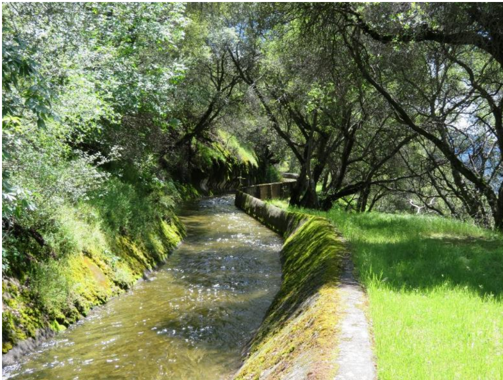
Figure CUL 5-54 Marble Fork Flowline ditch section, camera facing southwest
