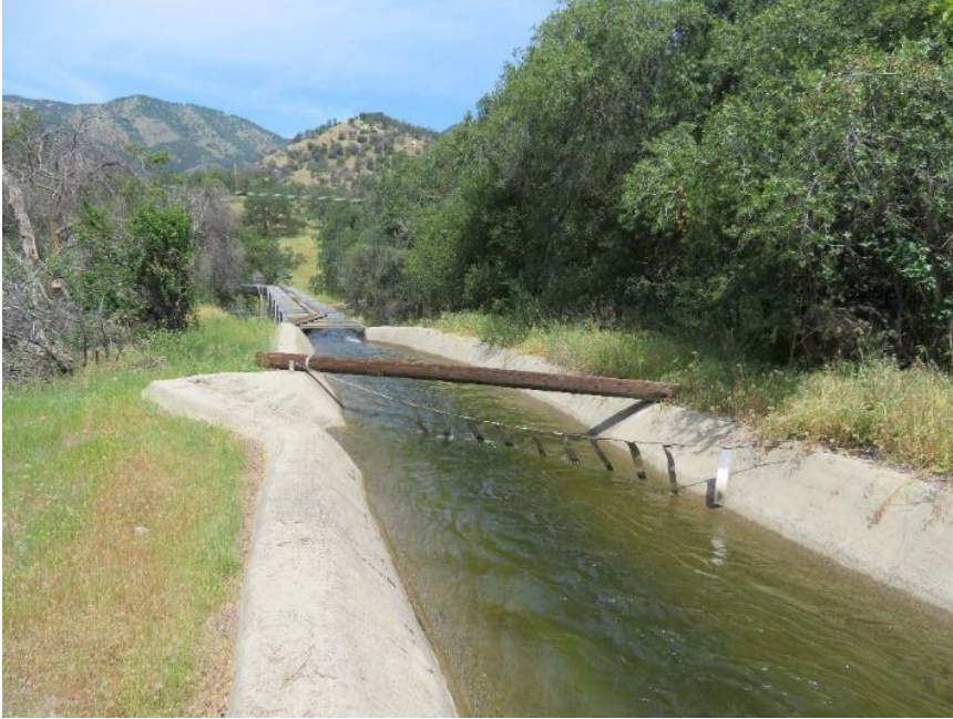
Figure CUL 5-44 Kaweah No. 2 Flowline, camera facing west
