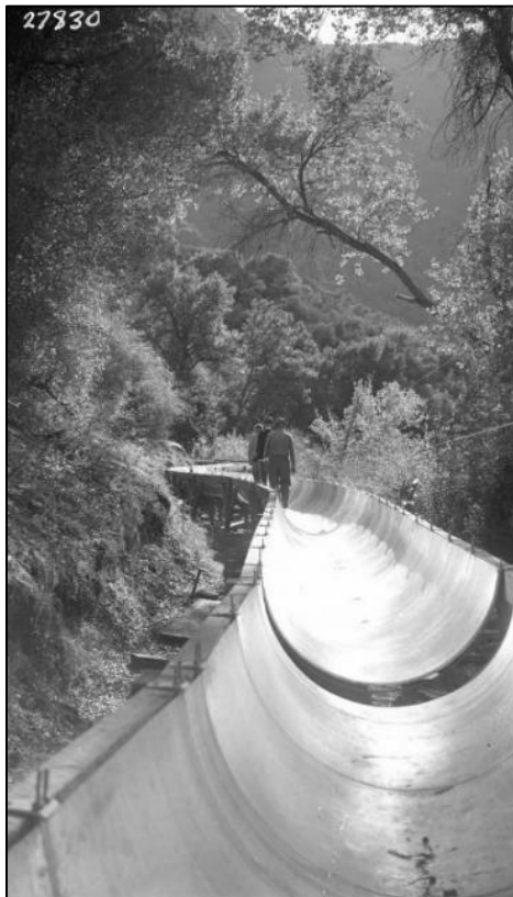
Figure 4. Kaweah No. 1 Flowline during reconstruction, 1947 (Huntington Library, Call Number 02 - 27830).
