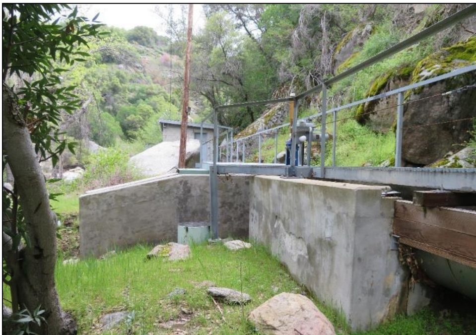
Photograph 9. Modern concrete spillway with gauge house in distance, camera facing southeast. April 18, 2018.
