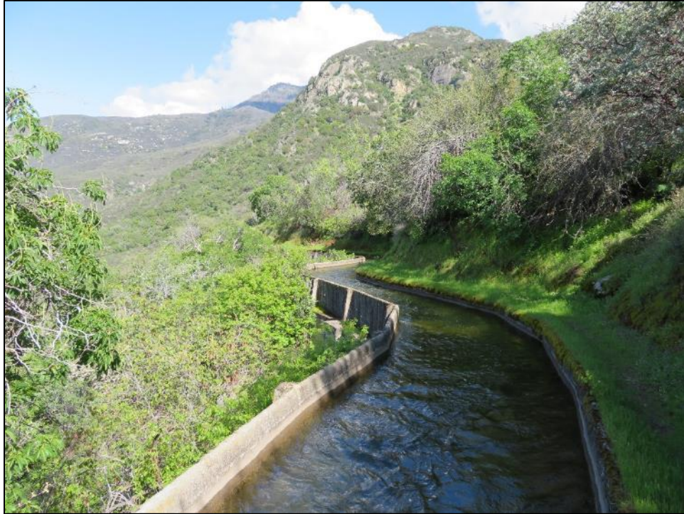
Photograph 2. Middle Fork Flowline, camera facing northeast. April 17, 2018.
