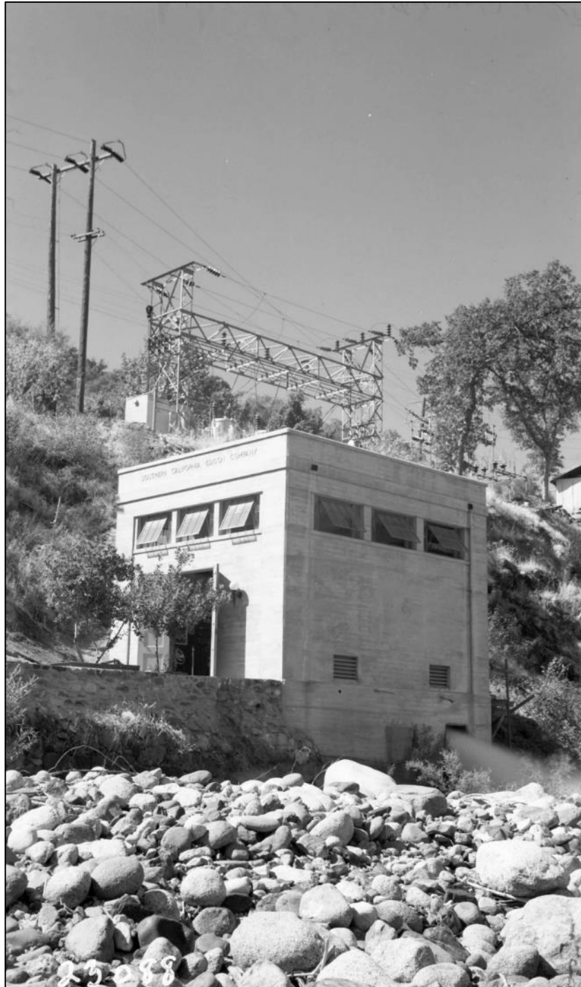
Photograph 3. Kaweah No. 1 Powerhouse and Substation, 1940 (Huntington Library, Call Number 02 - 23088).
