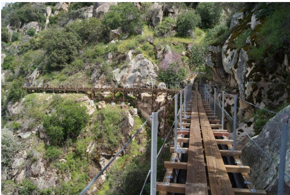
Figure CUL 5-33 Section of Kaweah No. 1 Flowline, camera facing southeast
