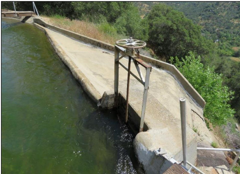
Photograph 11. Slide gate and concrete spillway along flowline, camera facing north. May 8, 2018
