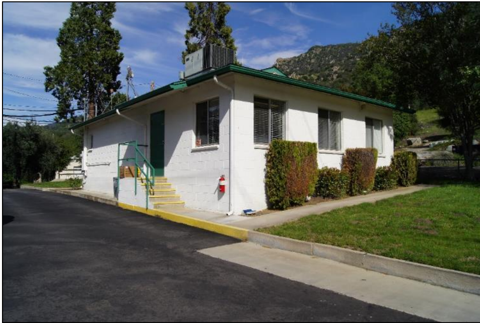
Photograph 2. Kaweah Office, showing north and west sides, camera facing southeast. April 18, 2018.
