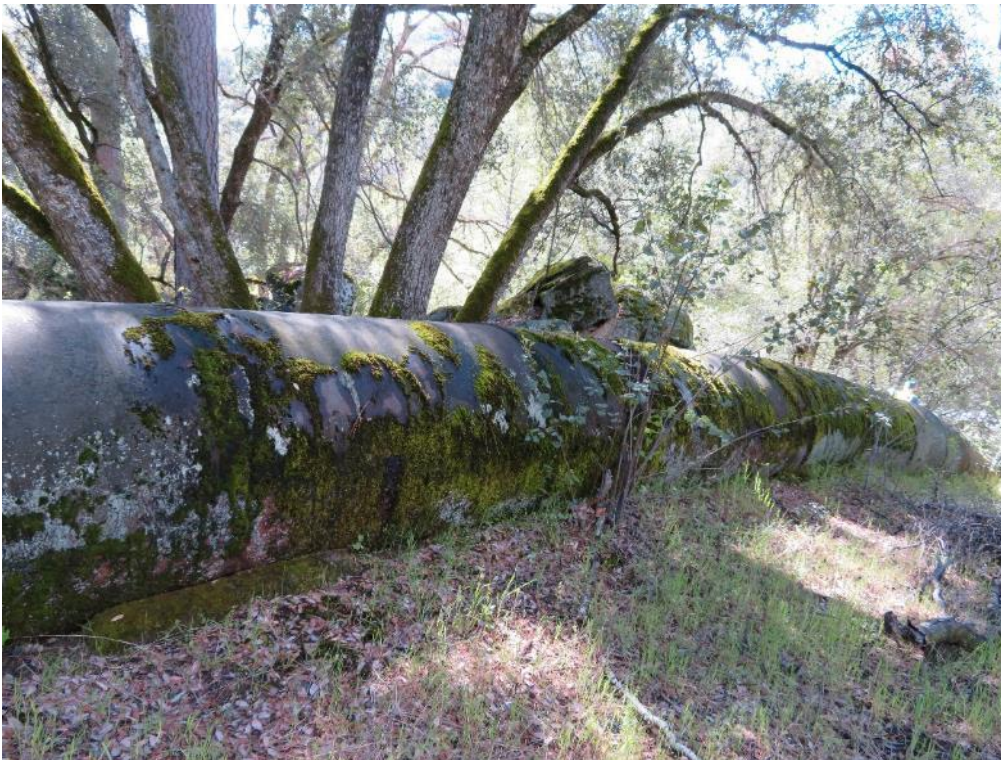
Figure CUL 5-56 Marble Fork Siphon, camera facing east
