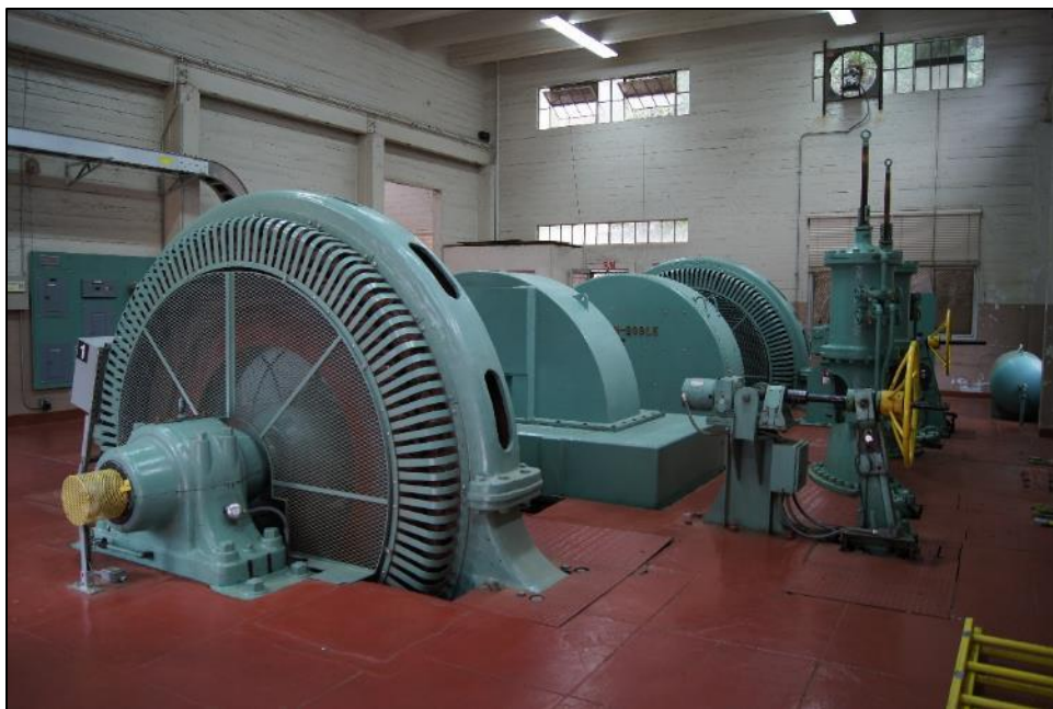
Photograph 6. Kaweah No. 3 Powerhouse interior, camera facing northwest. April 19, 2018.
