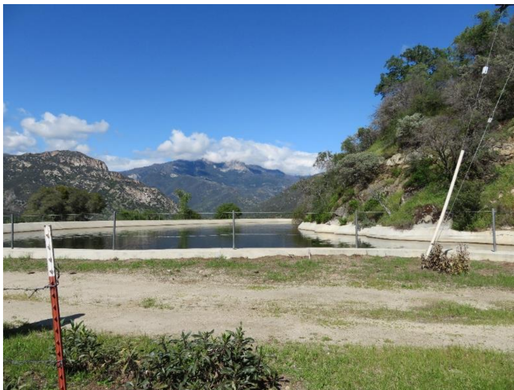
Figure CUL 5-63 Kaweah No. 3 Forebay, camera facing east
