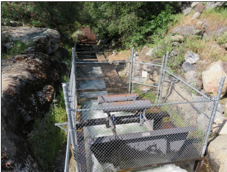
Photograph 7. Water control gate and fish wheel, camera facing southwest. May 8, 2018.
