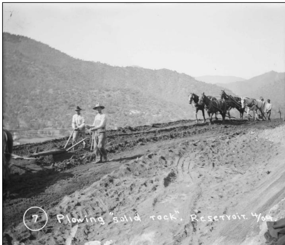
Figure 1. Grading for construction of Kaweah No. 2 Forebay, 1904 (Huntington Library, Call Number 04 - 00013).
