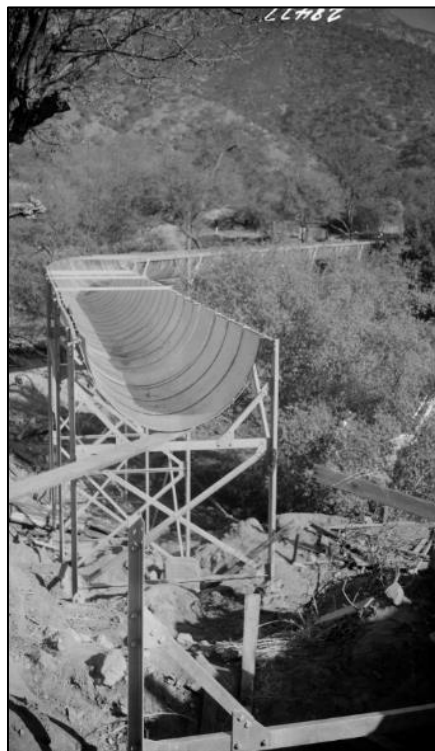
Figure 3. Reconstruction of Kaweah No. 2 Flowline, note metal flume and support structure, 1948 (Huntington Library, Call Number 02 - 28477).
