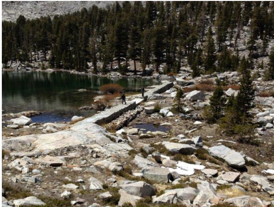
Photograph 2. Eagle Lake Dam. SCE, 2018.
