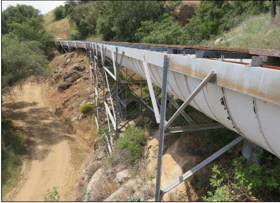
Photograph 4. Flume span along Kaweah No. 2 Flowline, note replacement metal support structure, camera facing northwest. May 8, 2018.
