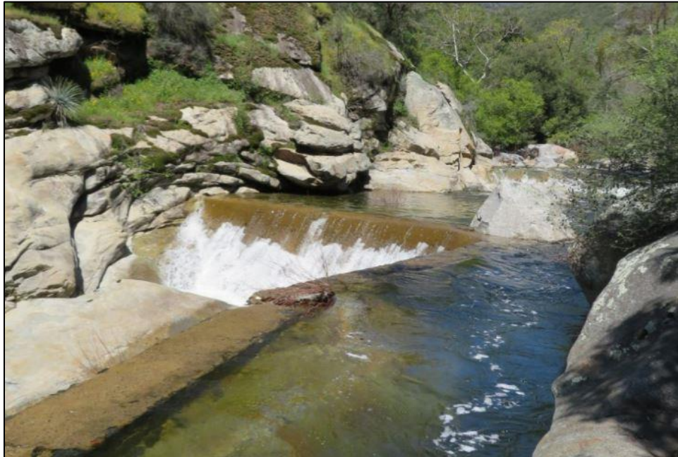
Photograph 2. Marble Fork Diversion Dam and intake, camera facing northeast. April 17, 2018.
