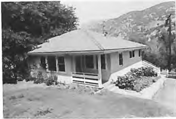
Bldg. 0121, Cottage Kaweah Powerhouse No. 1 View to NW Roll 1, Frame 20, 6-27-89
