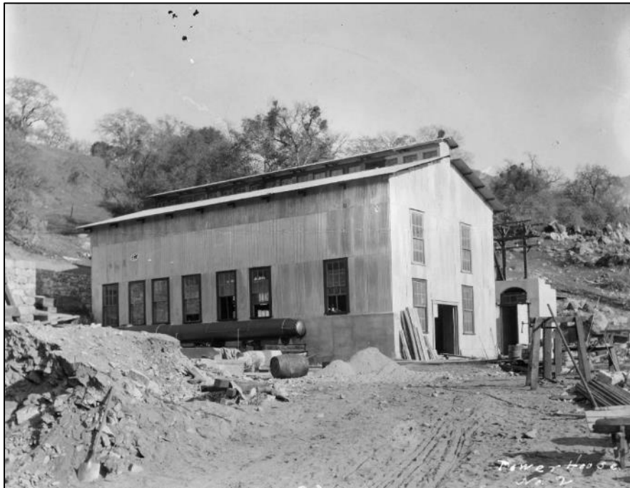
Figure 2. Kaweah No. 2 Powerhouse nearing completion, 1904 (Huntington Library, Call Number 04 - 00069).
