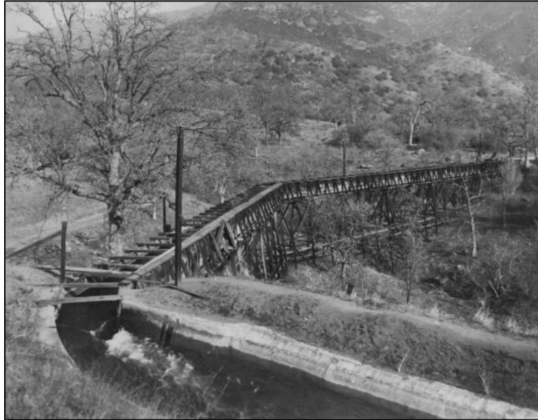
Figure 2. Kaweah No. 2 Flowline, ca. 1908 (Huntington Library, Call Number 04 - 00732).
