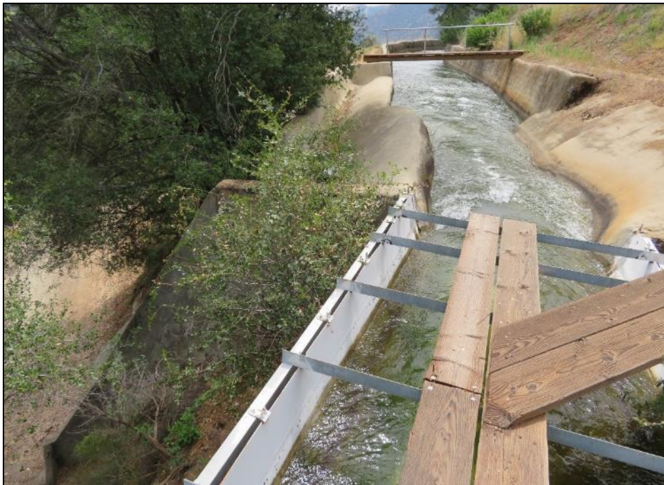
Photograph 5. Spillway at east end of forebay, camera facing northwest. May 8, 2018.
