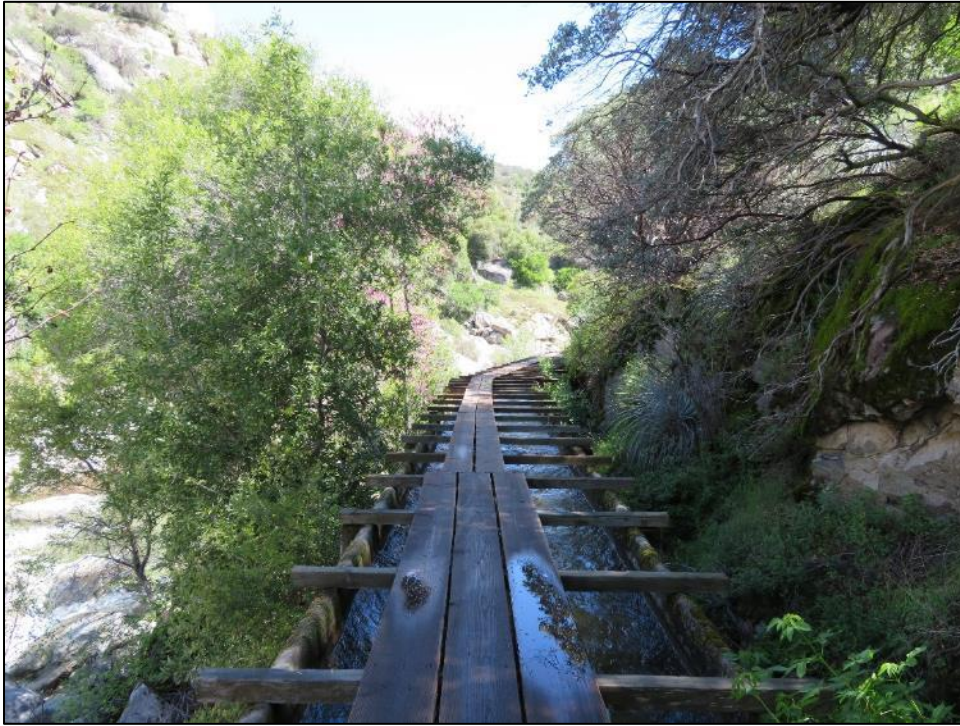
Photograph 4. Middle Fork Flowline catwalk near Middle Fork Diversion, camera facing northeast. April 17, 2018.
