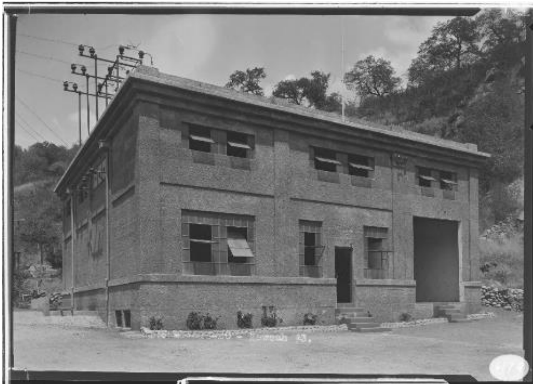
Figure 15: Kaweah No. 3 Powerhouse, 1920 (Huntington Digital Library, SCE Photograph Collection, Call Number 02 - 06179)
