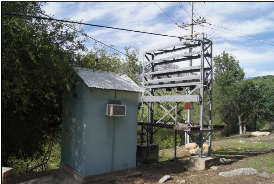
Photograph 9. Communications House and tower, camera facing northeast. April 18, 2018.
