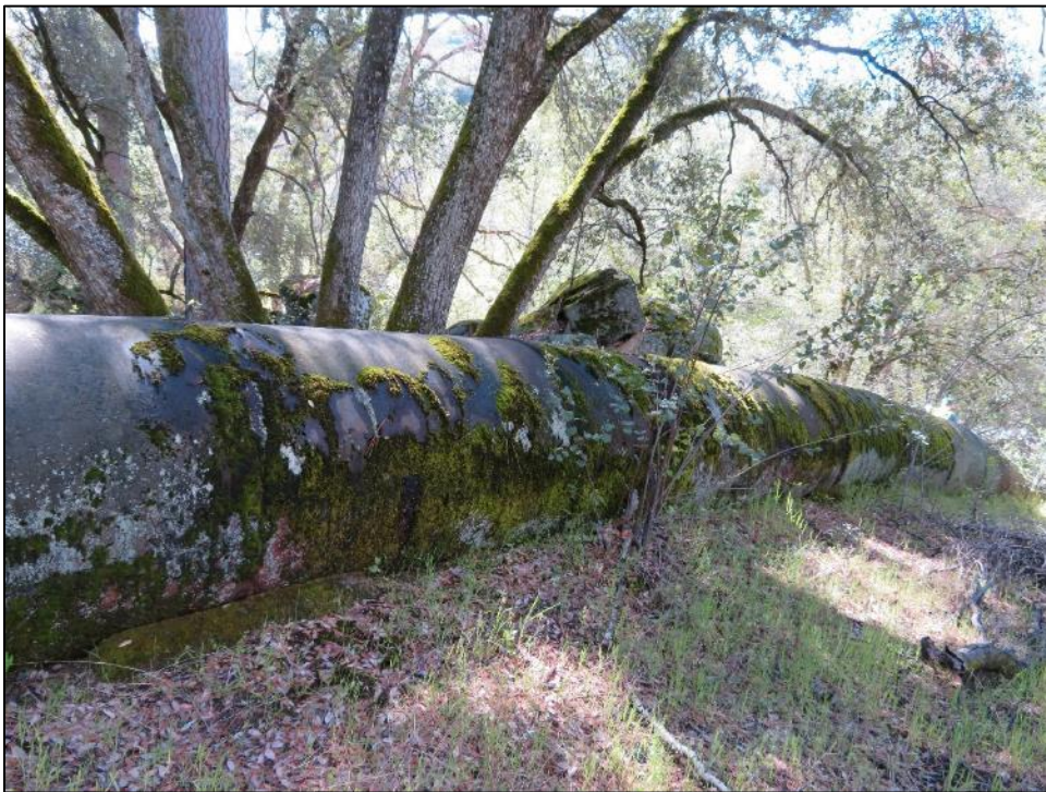
Photograph 7. Marble Fork Siphon, camera facing southeast. April 17, 2018.
