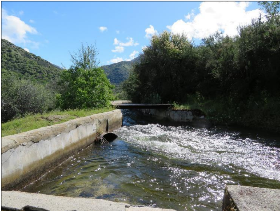
Photograph 7. Junction of Marble Fork Siphon and the Middle Fork Flowline, camera facing east. April 17, 2018.
