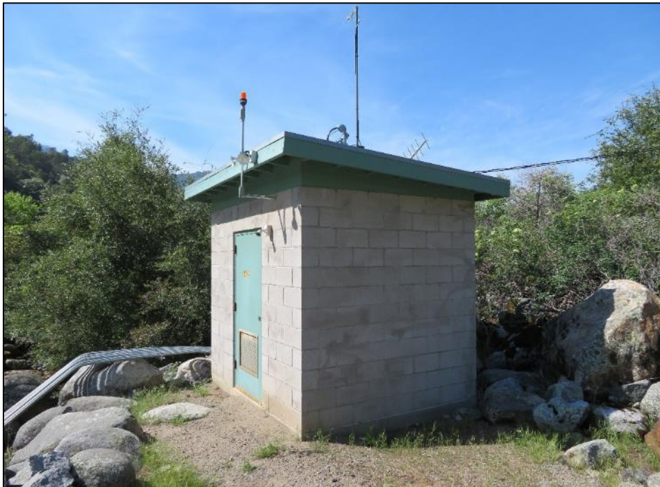
Photograph 5. Control Building. Camera facing west. April 18, 2018.
