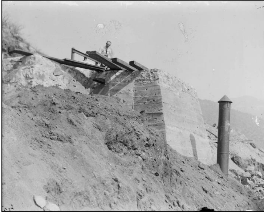
Figure 2. Kaweah No. 2 Forebay nearing completion, 1904 (Huntington Library, Call Number 04 - 00072).
