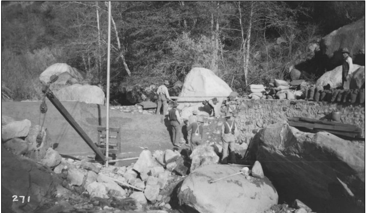
Figure 1. Middle Fork Diversion under construction, ca. 1912 (Huntington Library, Call Number 04 - 00271).
