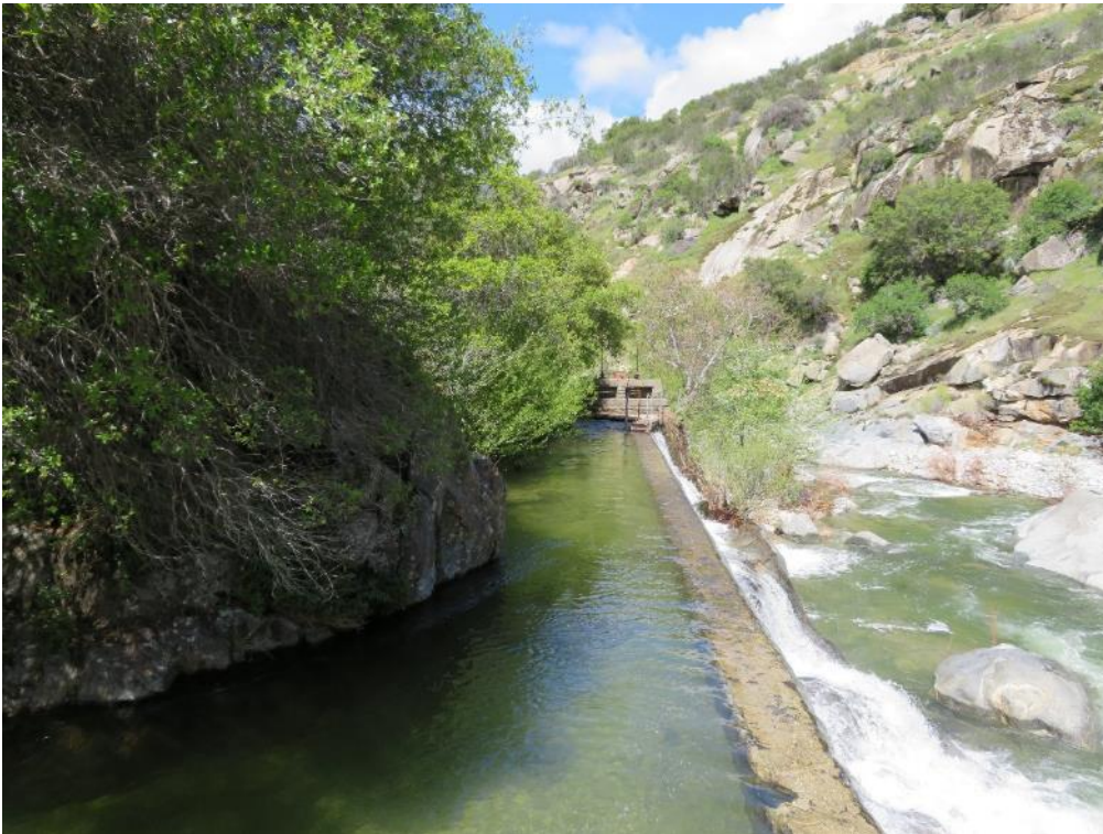
Figure CUL 5-59 Middle Fork Diversion Dam Sandbox, camera facing west
