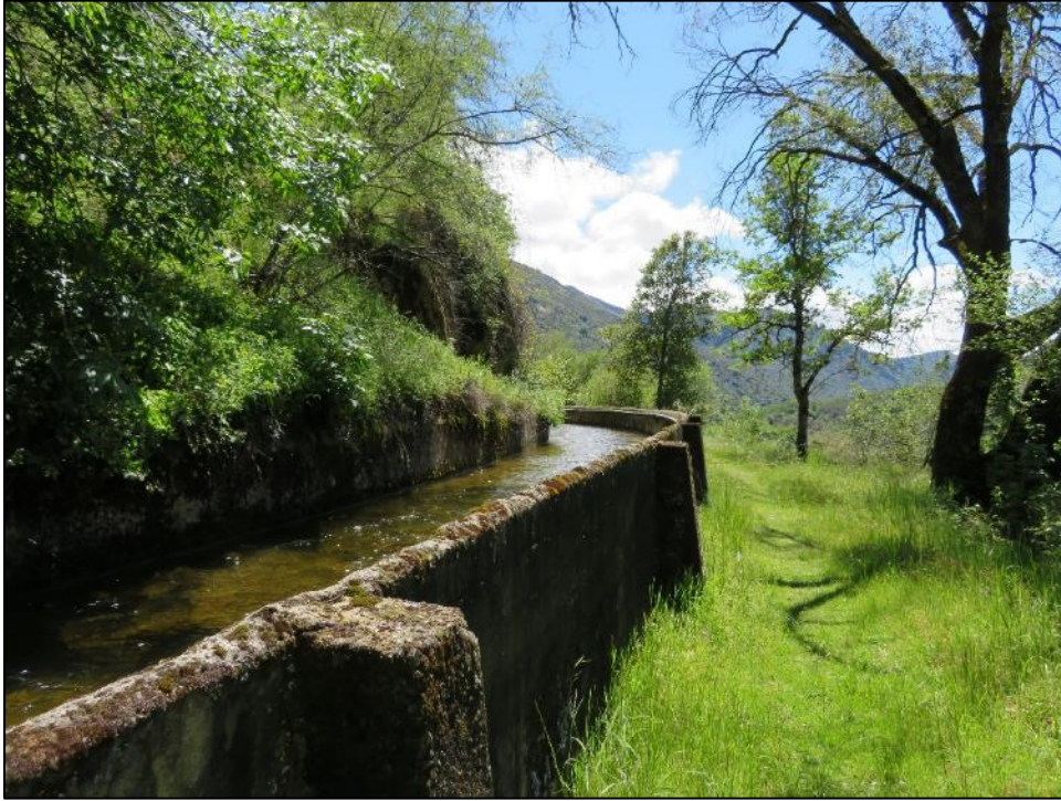
Photograph 2. Marble Fork Flowline showing flume section, camera facing southeast. April 17, 2018.
