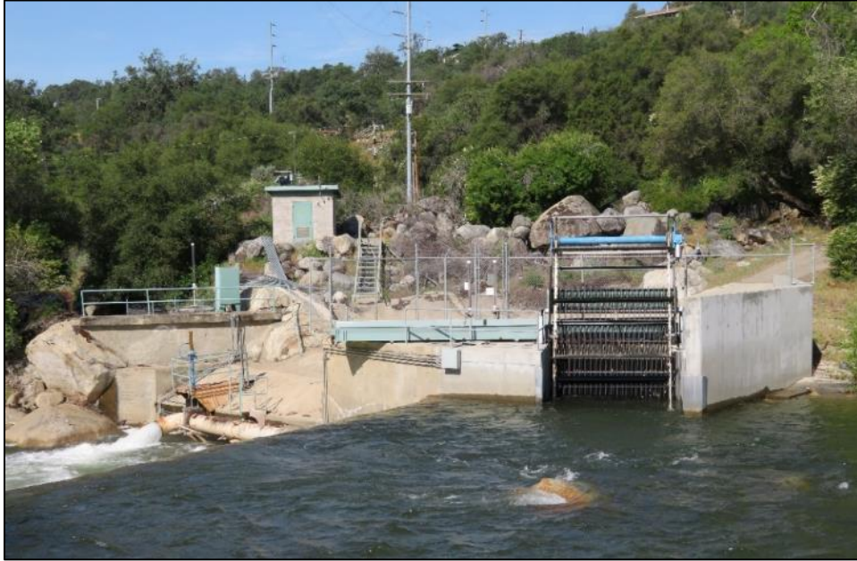
Photograph 2. Kaweah No. 2 Diversion intake structure, note metal trash rack, camera facing east. April 18, 2018.
