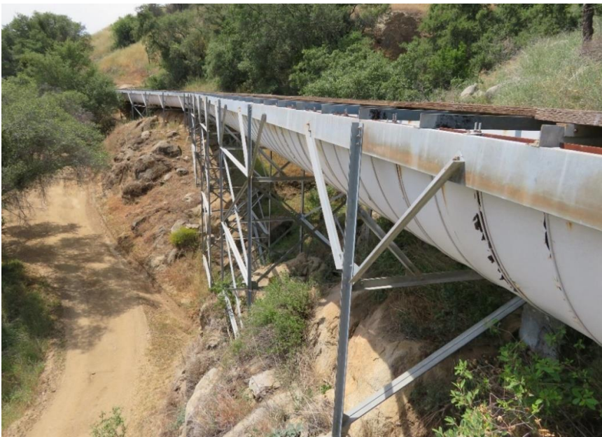
Figure CUL 5-45 Flume Section of Kaweah No. 2 Flowline, camera facing west
