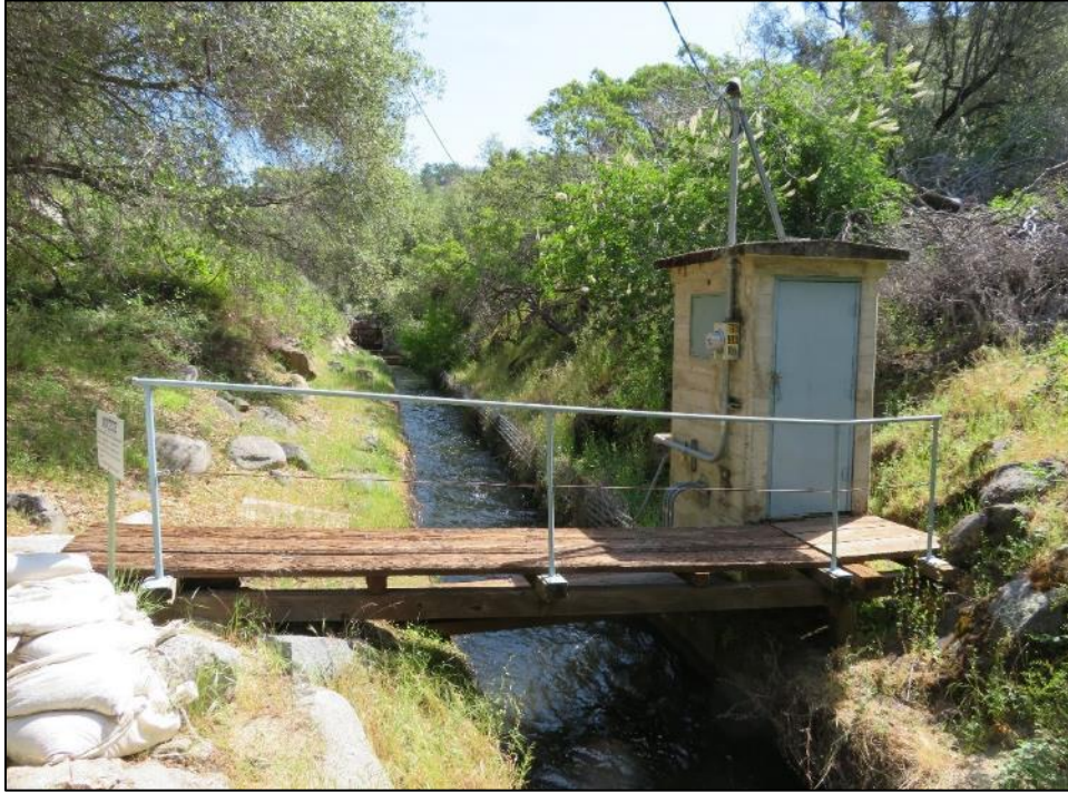
Photograph 8. Recorder building along first concrete ditch segment, camera facing northeast. May 8, 2018.
