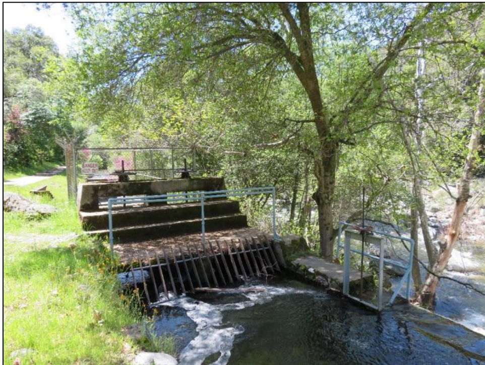
Photograph 6. Trash rack and slide gates at Marble Fork Diversion, camera facing southwest. April 17, 2018.
