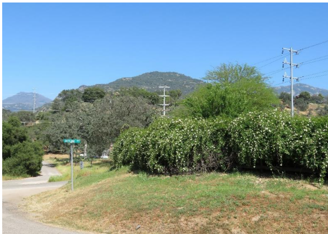
Figure CUL 5-67 Kaweah Powerhouse No. 3 to Three Rivers Substation Transmission Line, camera facing south
