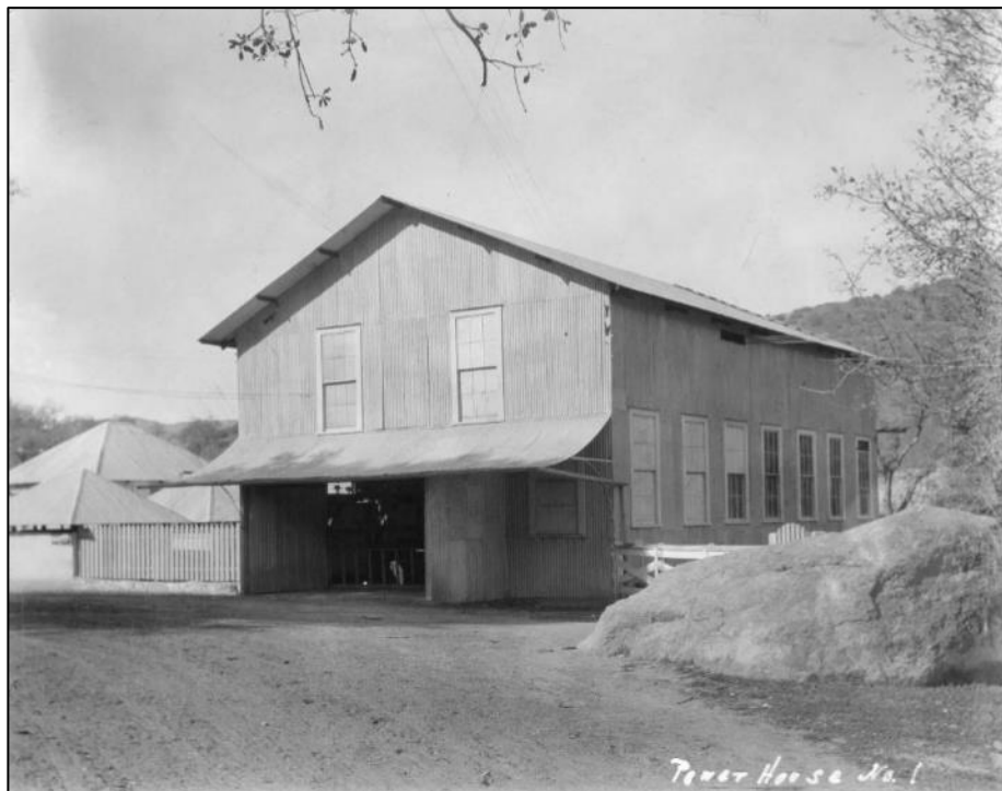
Photograph 2. Original corrugated metal powerhouse, 1904 (Huntington Library, Call Number 04 - 00041).
