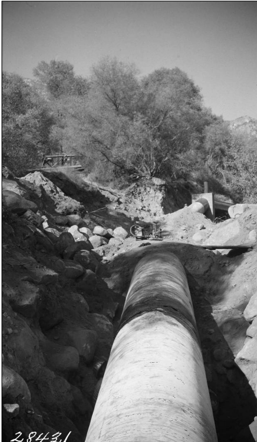
Figure 4. Replacing Flume 1 with metal siphon, 1948 (Huntington Library, Call Number 02 - 28431).
