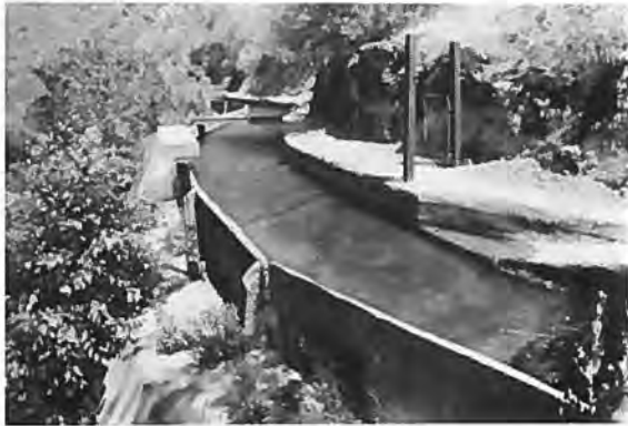
Marble Fork Flume Kaweah Powerhouse No. 3 View to NNW Roll 2, Frame 16, 6-27-89
