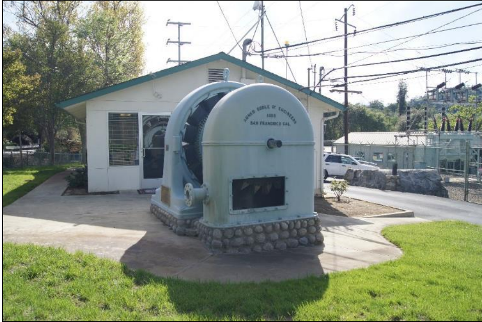
Photograph 4. Original Kaweah No. 1 Powerhouse generator, camera facing southwest. April 18, 2018.
