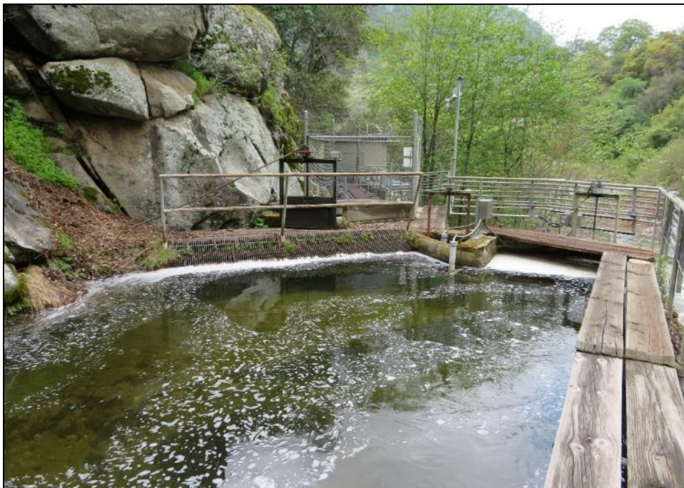
Photograph 7. West end of sandbox showing trash rack and slide gate, camera facing southwest. April 18, 2018.
