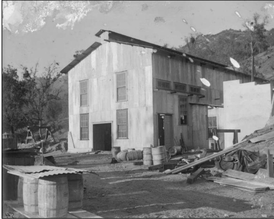
Figure 1. Kaweah No. 2 Powerhouse nearing completion, 1904 (Huntington Library, Call Number 04 - 00054).
