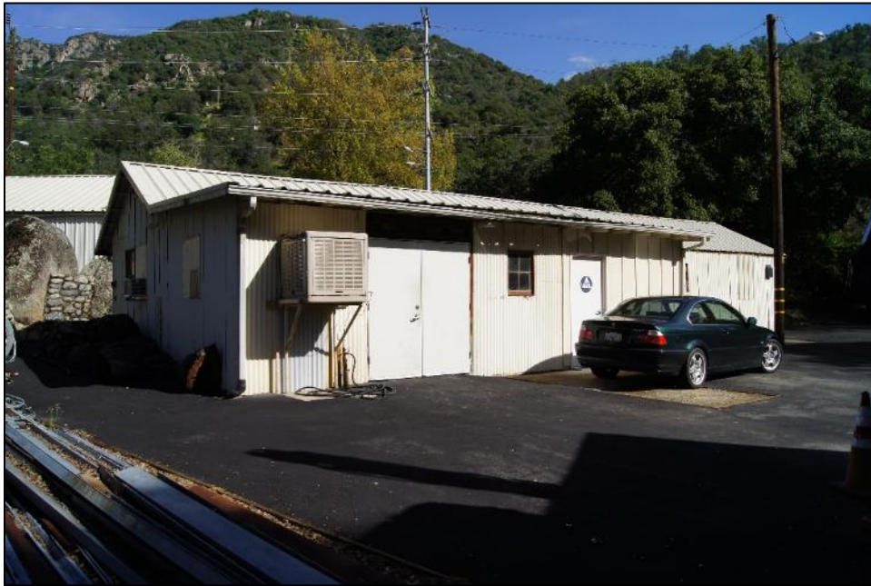
Photograph 8. Work Shop, camera facing southeast. April 18, 2018.
