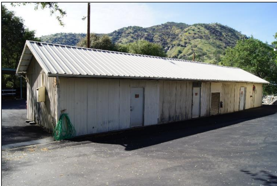
Photograph 7. Workshop, showing south and east sides, camera facing northwest. April 18, 2018.
