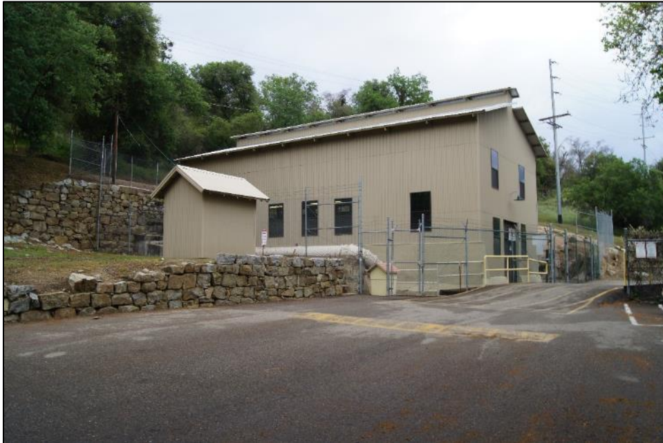
Photograph 2. Kaweah Powerhouse No. 2, camera facing west. April 19, 2018.
