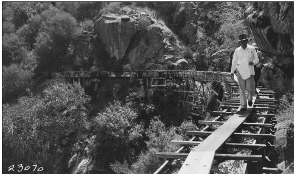
Figure 2. Men walking on Kaweah No. 1 Flowline, note redwood box flume, 1940 (Huntington Library, Call Number 02 - 23070).
