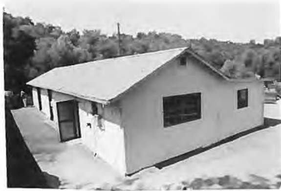
Bldg. 0110, Carpenter Shop/Garage Kaweah Powerhouse No. 1 View to SW Roll 1, Frame 12, 6-27-89
