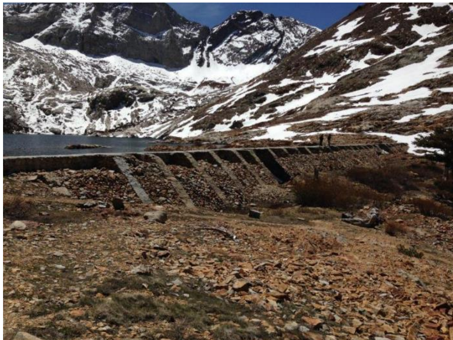
Photograph 3. Upper Monarch Lake Dam. SCE, 2018.
