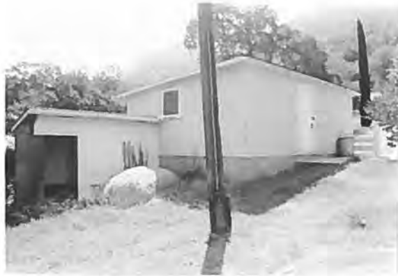
Bldg. 0123, Garage Kaweah Powerhouse No. 1 View to E Roll 1, Frame 22, 6-27-89
