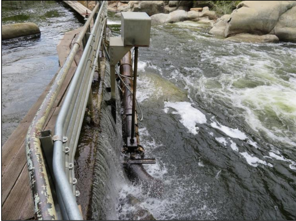
Photograph 6. Former fish passage pipe, camera facing southwest. April 18, 2018.
