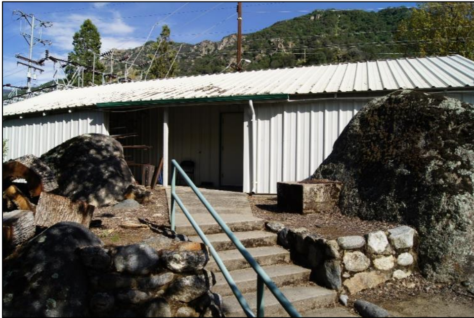
Photograph 6. North side of Operator's Office, camera facing southeast. April 18, 2018.
