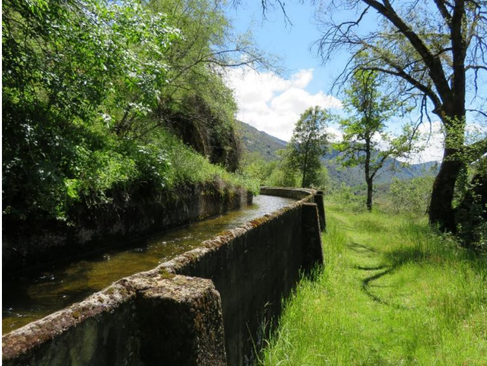
Figure CUL 5-53 Marble Fork Flowline flume section, camera facing southwest
