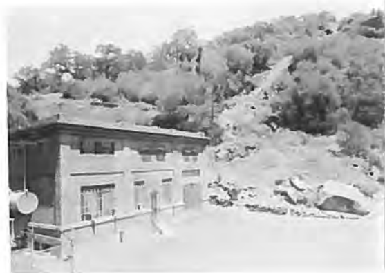
Bldg. 0101 Kaweah Powerhouse No. 3 View to E Roll 2, Frame 13, 6-27-89
