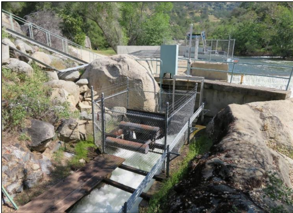
Photograph 3. Diversion Outlet to Kaweah No. 2 Flowline, camera facing south. April 18, 2018.
