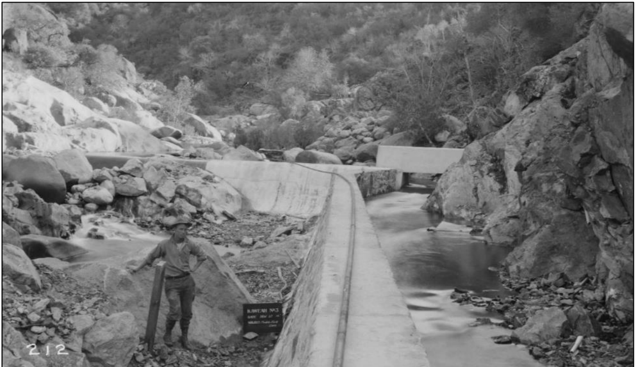
Figure 2. Middle Fork Diversion nearly complete, ca. 1912 (Huntington Library, Call Number 04 - 00212).
