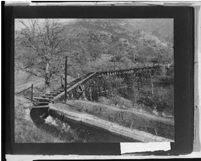
Figure 11: Kaweah No. 2 Concrete Ditch and Flume Section, circa 1908 (Huntington Digital Library, SCE Photograph Collection, Call Number 04 - 00732)
