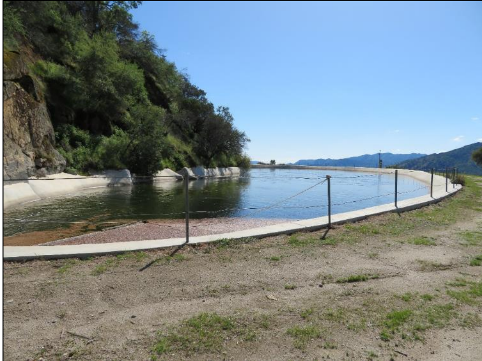
Photograph 2. Kaweah No. 3 Forebay, camera facing west. April 17, 2018.
