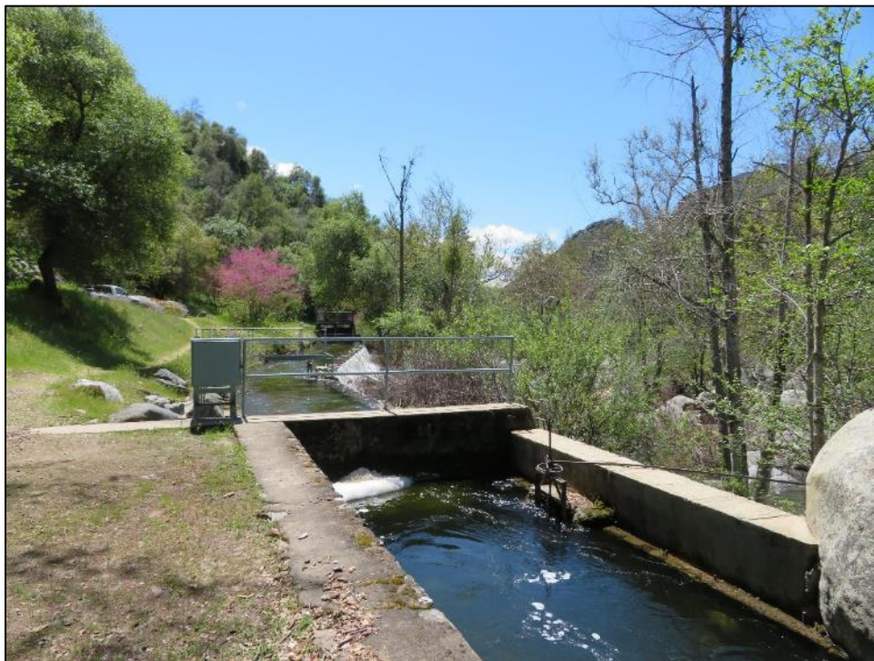
Photograph 3. Marble Fork Diversion Sandbox showing concrete barrier, camera facing south. April 17, 2018.
