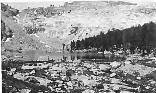
Eagle Lake Dam SCE Historical Photo Album View to S 7-21-33
