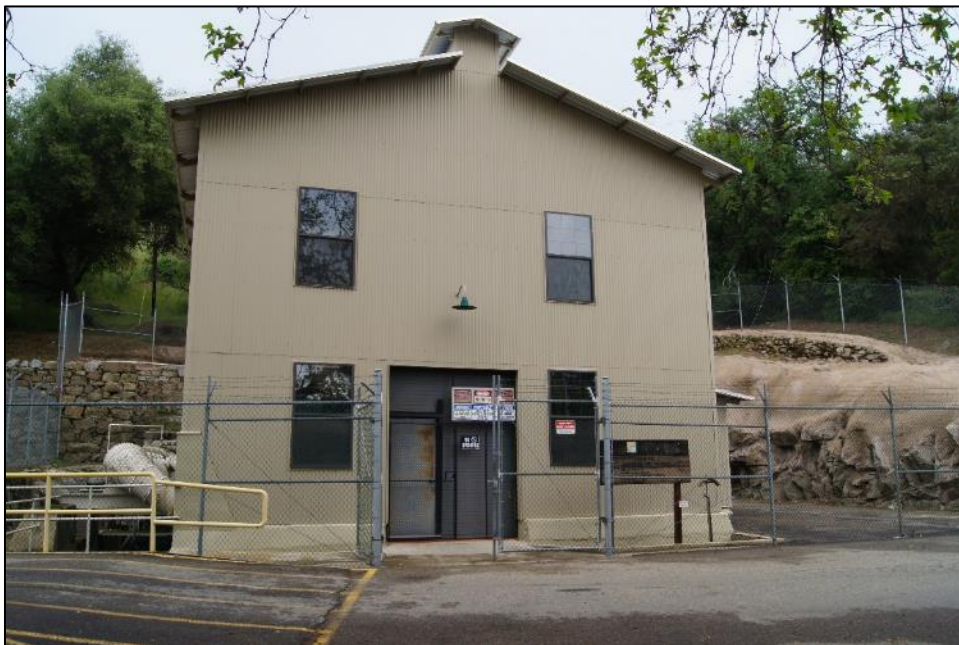
Photograph 3. West side of Kaweah Powerhouse No. 2, camera facing northeast. April 19, 2018.
