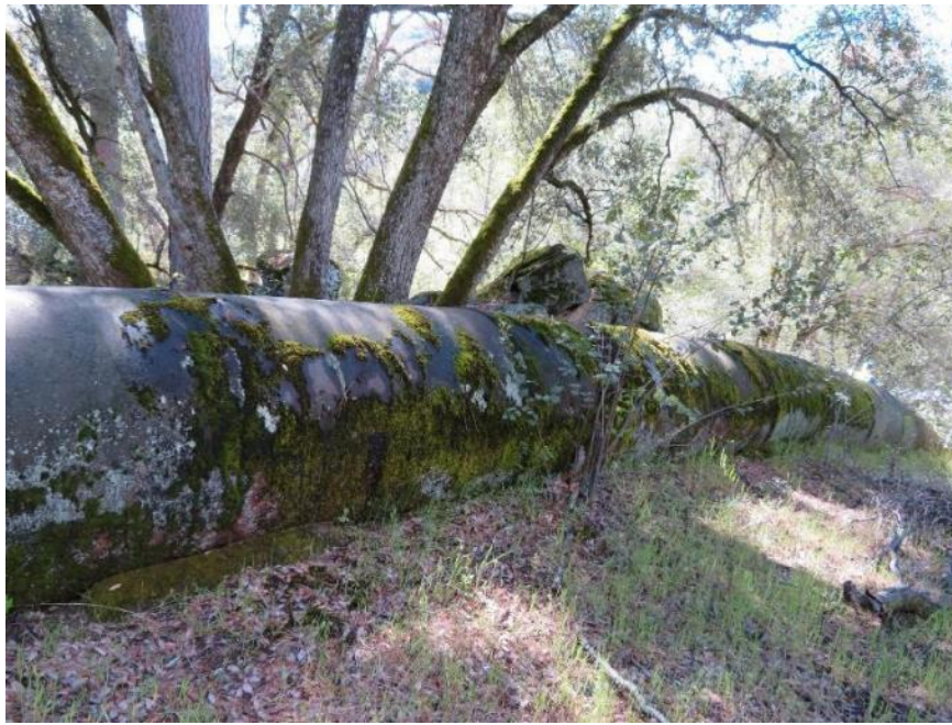
Photograph 4. Marble Fork Siphon, camera facing east. April 17, 2018.
