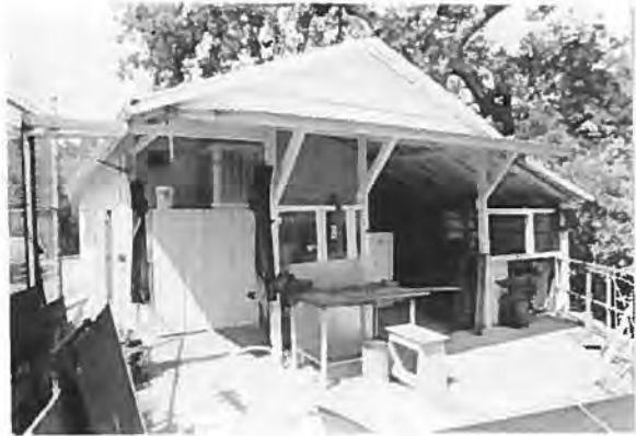
Bldg. 0107, Shop Kaweah Powerhouse No. 1 View to S Roll 1, Frame 16, 6-27-89
