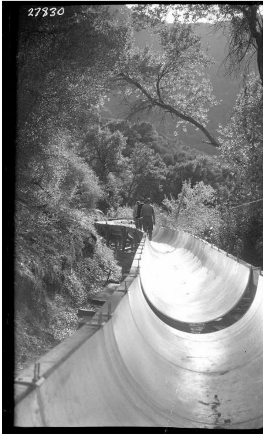
Figure 25: Rebuilt Kaweah No. 1 Flume, 1948 (Huntington Digital Library, SCE Photograph Collection, Call Number 02-27830)
