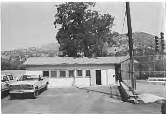
Bldg. 0107, Shop Kaweah Powerhouse No. 1 View to NW Roll 1, Frame 17, 6-27-89
