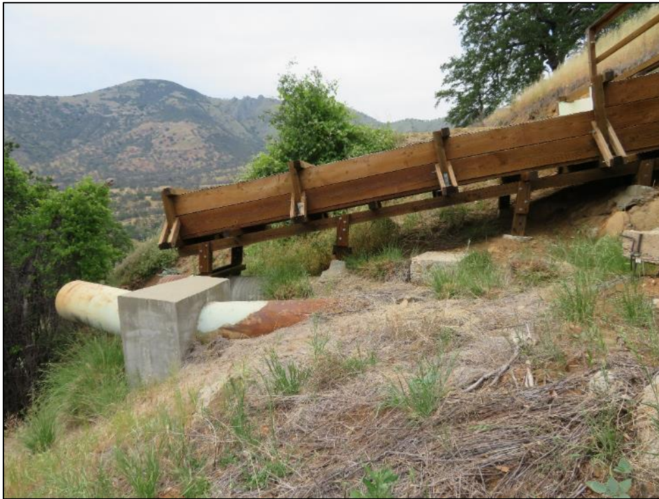
Photograph 4. Modern spillway chute and drainage pipes, camera facing west. May 8, 2018.
