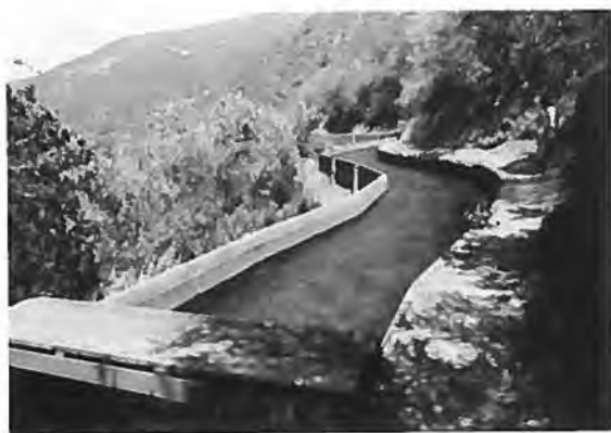
Middle Fork Flume Kaweah Powerhouse No. 3 View to NE Roll 2, Frame 17, 6-27-89
