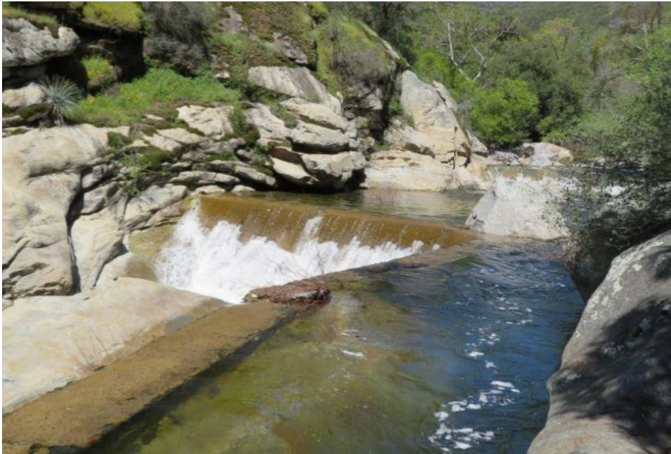
Photograph 2. Marble Fork Diversion Dam, camera facing north. April 17, 2018.
