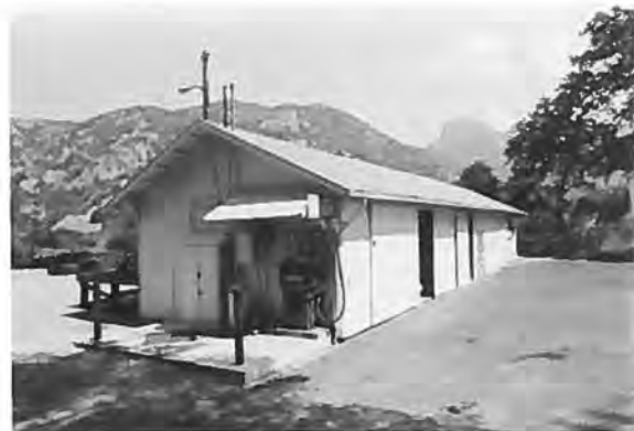
Bldg. 0110, Carpenter Shop/Garage Kaweah Powerhouse No. 1 View to NNW Roll 1, Frame 14, 6-27-89
