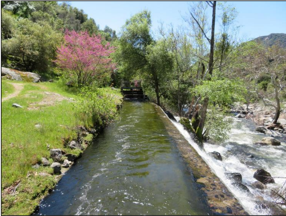
Photograph 4. Marble Fork Diversion Sandbox showing overflow spillway, camera facing south. April 17, 2018.
