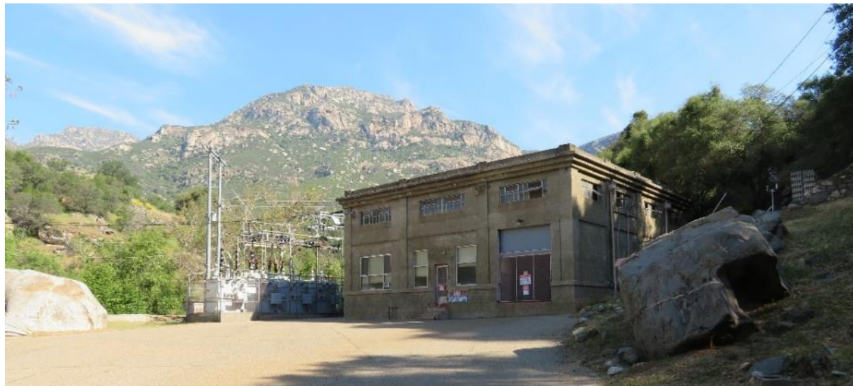
Figure CUL 5-47 Kaweah No. 3 Powerhouse, camera facing north
