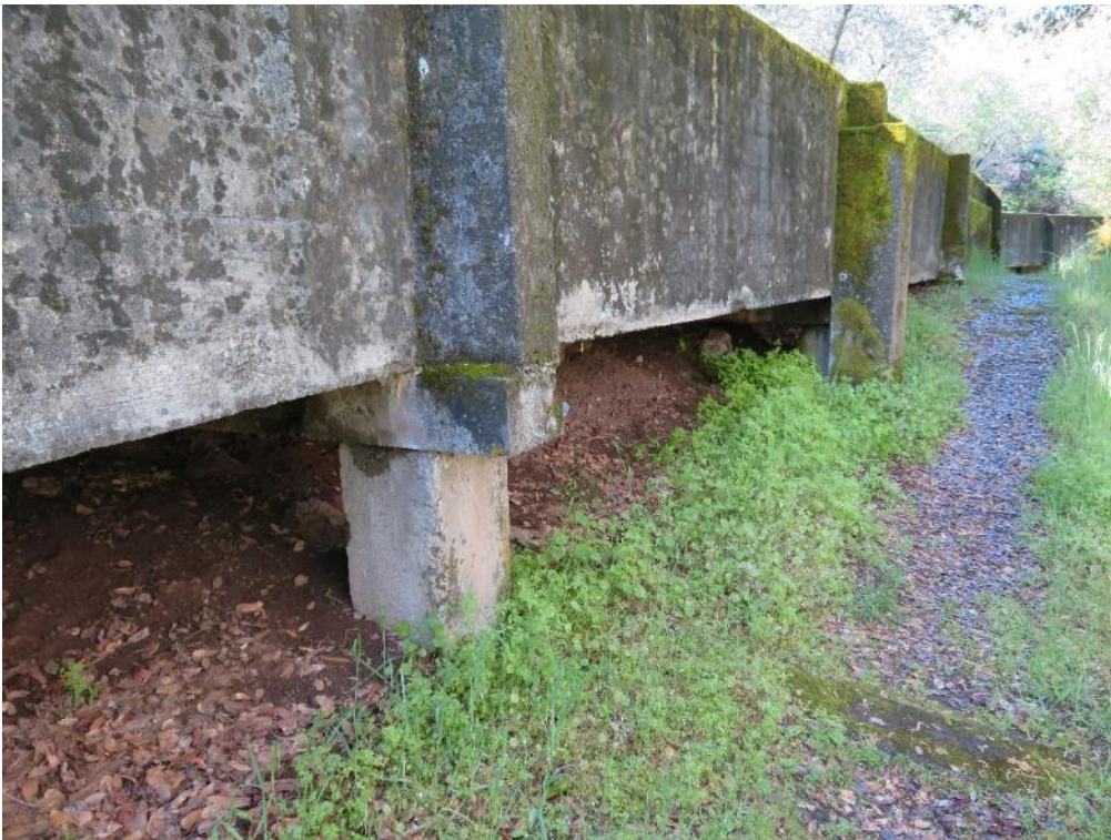
Figure CUL 5-62 Middle Fork Flowline, representative buttress and pier, camera facing west
