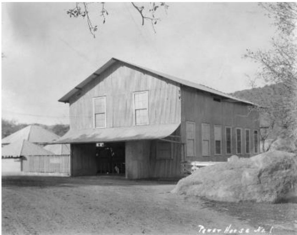
Figure 3: Kaweah No. 1 Powerhouse, 1904 (Huntington Digital Library, SCE Photograph Collection, Call Number 04–00041)
