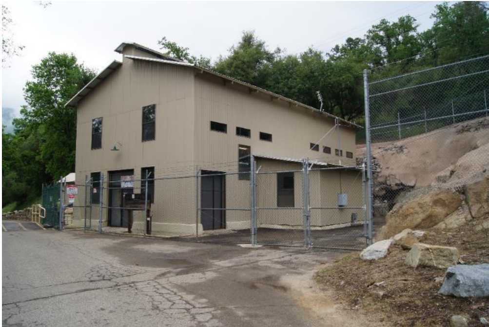
Figure CUL 5-40 Kaweah No. 2 Powerhouse, camera facing west
