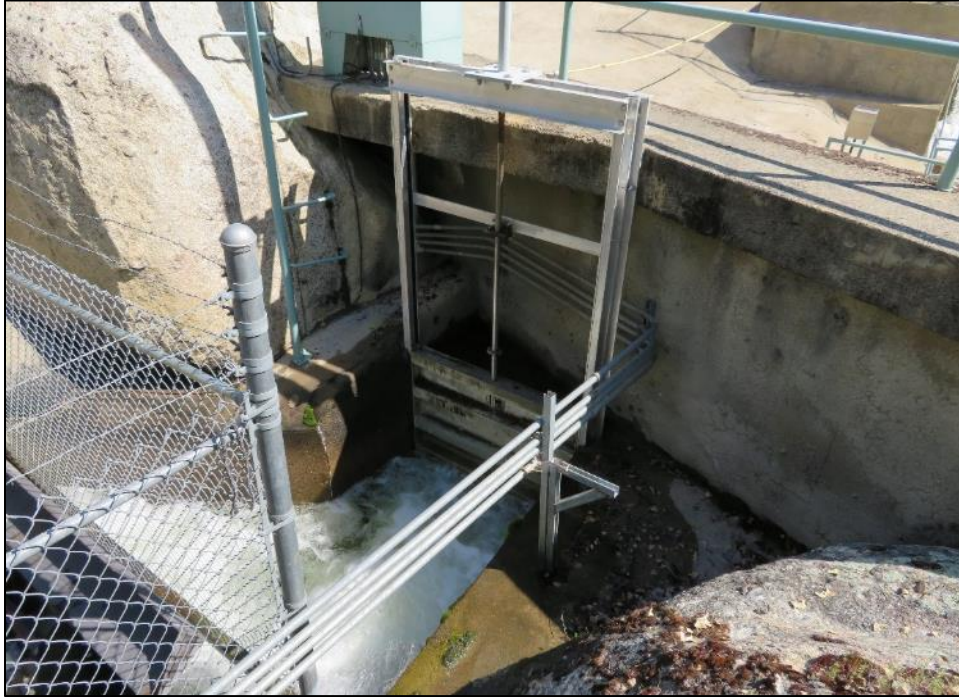
Photograph 6. Slide gate release to Kaweah No. 2 Flowline, camera facing north. May 8, 2018.
