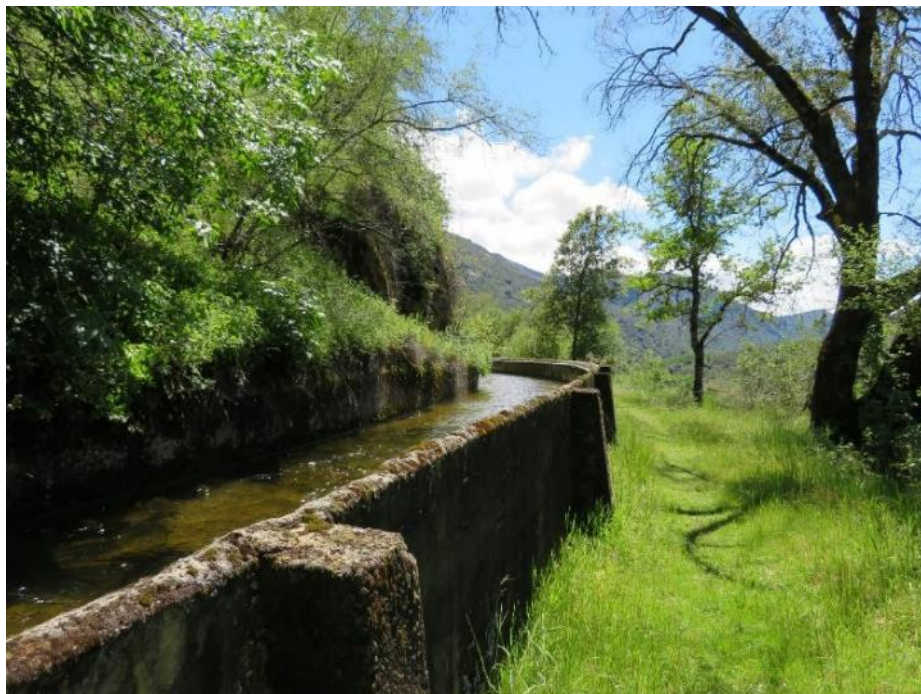
Photograph 3. Marble Fork Flowline, camera facing southwest. April 17, 2018.
