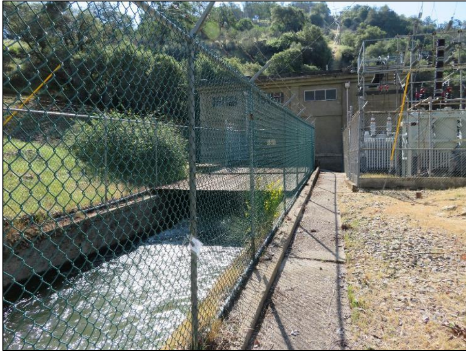
Photograph 7. Tailrace canal extending from Kaweah No. 3 Powerhouse, camera facing northeast. April 18, 2018.
