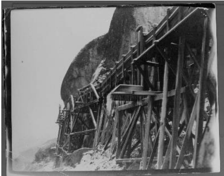
Figure 6: Representative Trestle Section of Kaweah No. 1 Flume, circa 1908 (Huntington Digital Library, SCE Photograph Collection, Call Number 04 - 00721)
