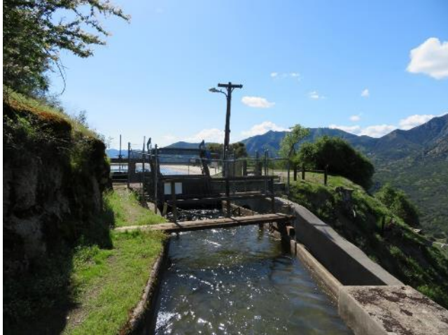
Figure CUL 5-64 Terminus of Kaweah No. 3 / Middle Fork Flowline at Kaweah No. 3 Forebay, camera facing west
