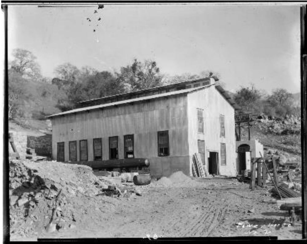
Figure 8: Kaweah No. 2 Powerhouse, 1904 (Huntington Digital Library, SCE Photograph Collection, Call Number 04 - 00069)
