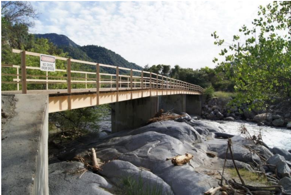
Figure CUL 5-50 Kaweah No. 3 Powerhouse Bridge, camera facing west
