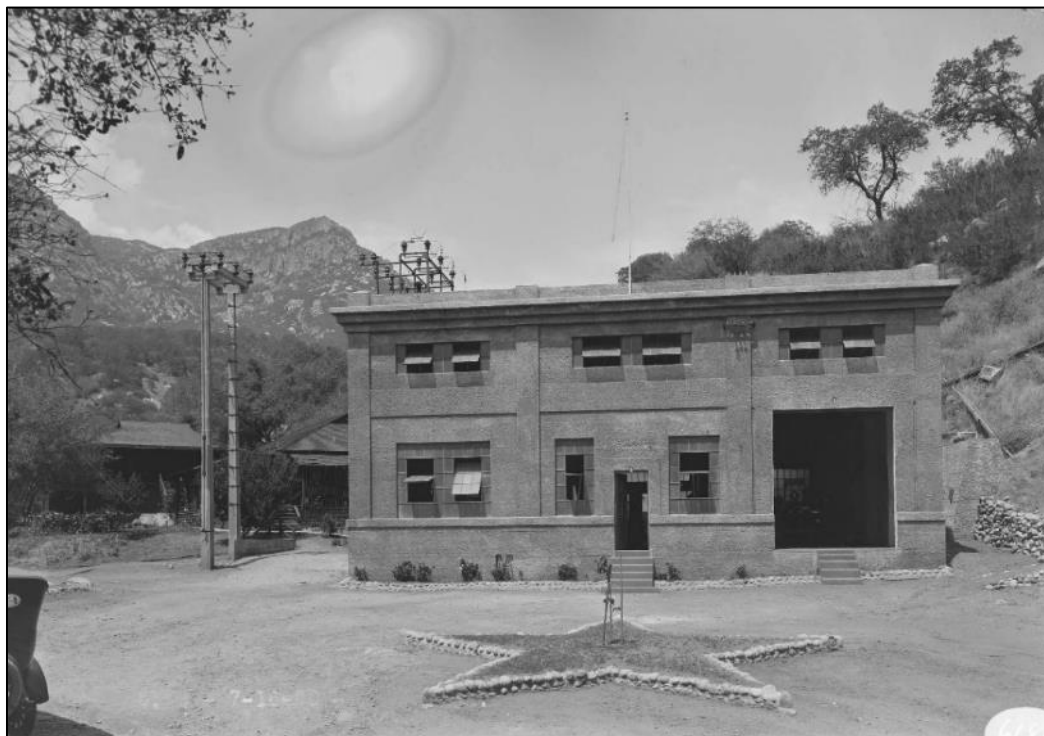
Figure 2. Kaweah No. 3 Powerhouse, 1920 (Huntington Library, Call Number 02 - 06180).
