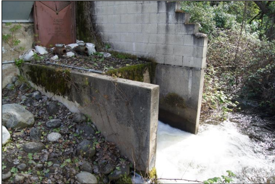
Photograph 10. Concrete tailrace channel, April 18, 2018.
