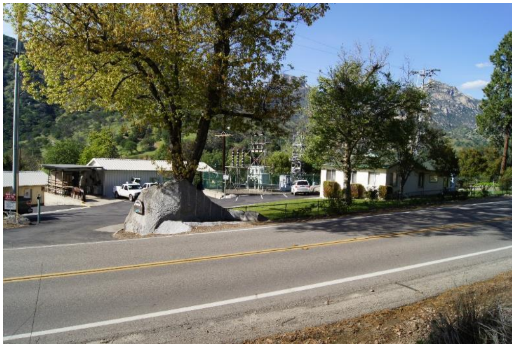
Figure CUL 5-35 Kaweah No. 1 Powerhouse Campus, camera facing northeast
