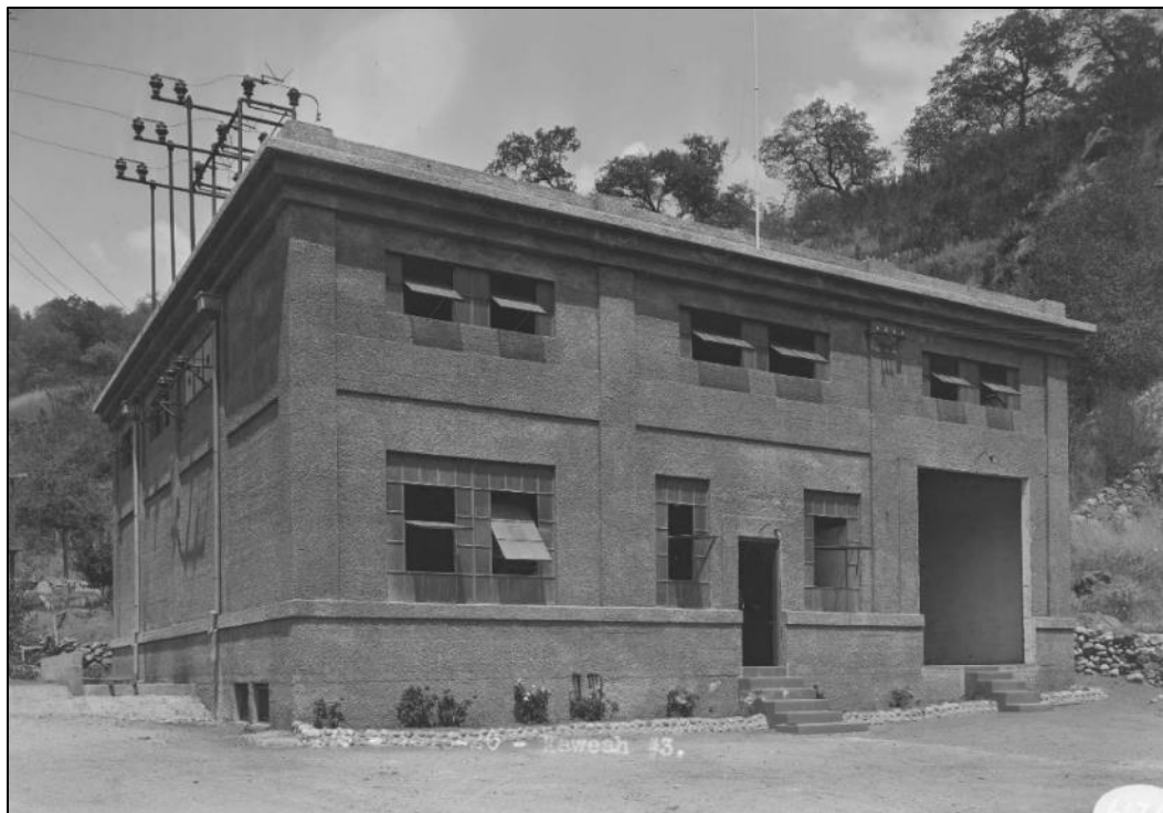
Figure 1. Kaweah No. 3 Powerhouse, 1920 (Huntington Library, Call Number 02 - 06179).
