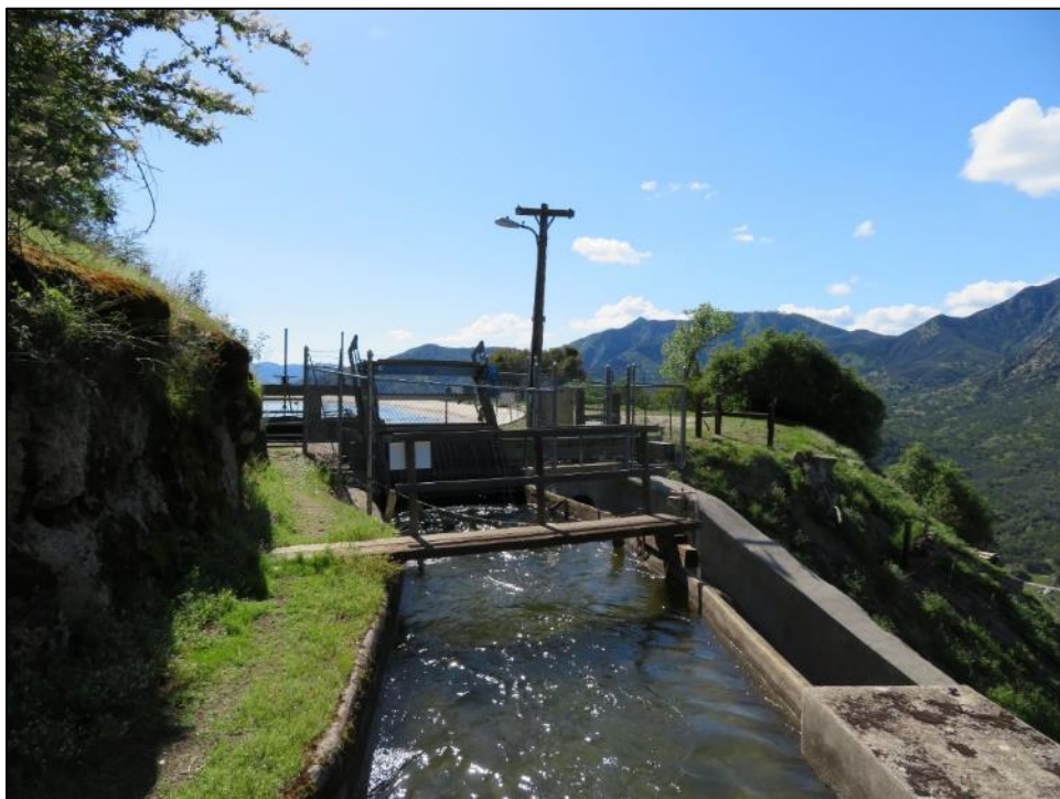
Photograph 3. Connection of Middle Fork Conduit with Kaweah No. 3 Forebay, camera facing west. April 17, 2018.
