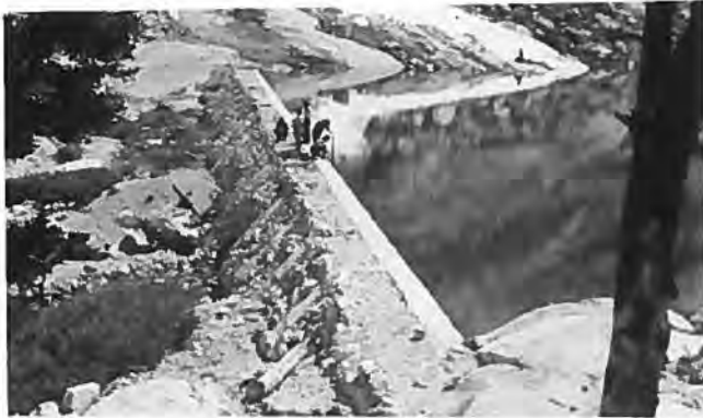
Monarch Lake Dam SCE Historical Photo Album View to NE 7-22-33
