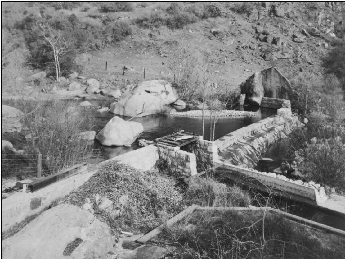
Figure 1. Kaweah No. 2 Diversion, 1904 (Huntington Library)
