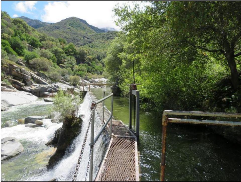
Photograph 4. Sandbox, note ungated spillway and two slide gates, camera facing east. April 17, 2018.
