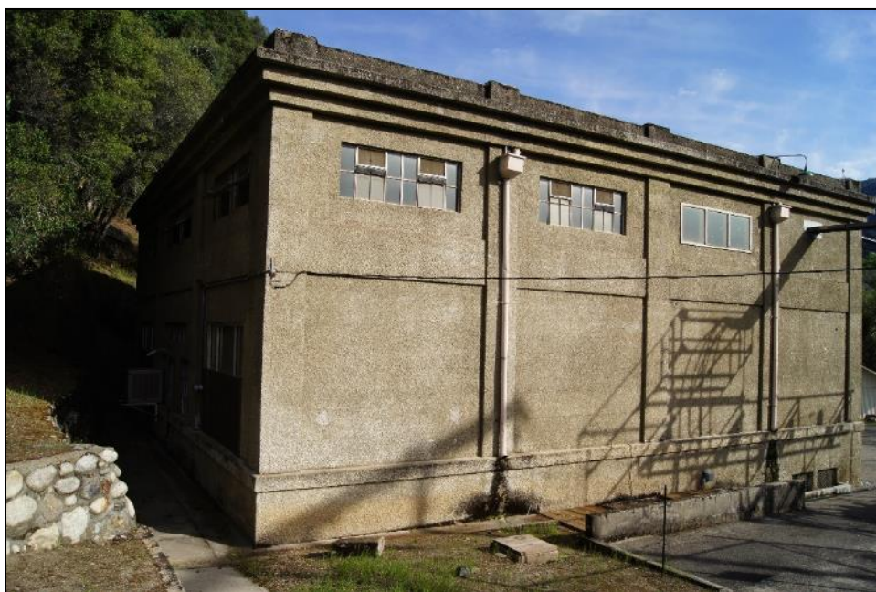
Photograph 3. Kaweah No. 3 Powerhouse, note bands of windows, camera facing southeast. April 18, 2018.
