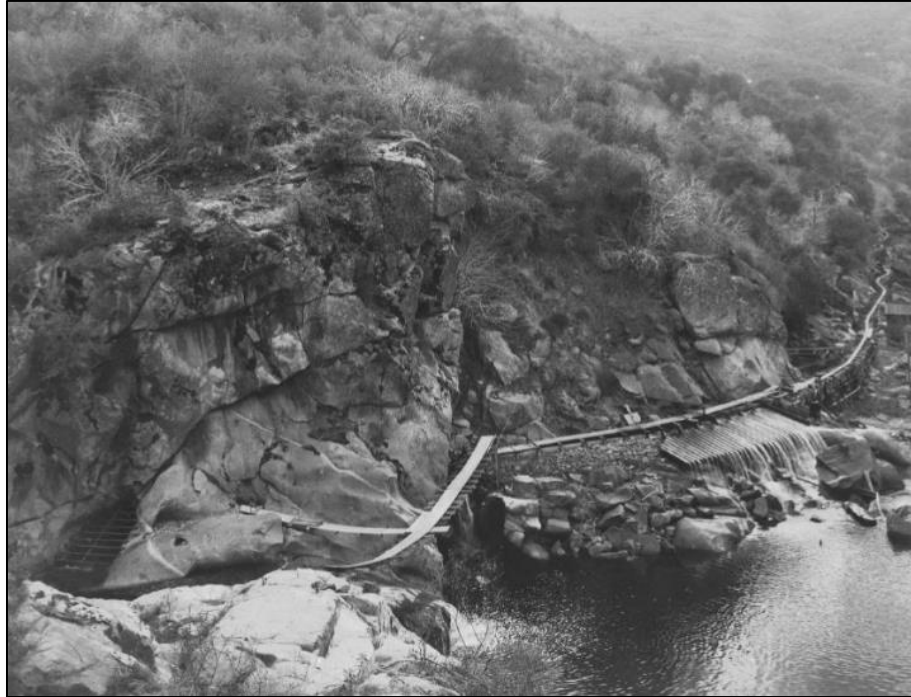
Figure 2. Kaweah No. 1 Diversion Intake, note lack of sandbox, 1904 (Huntington Library, Call Number 04 - 00720).
