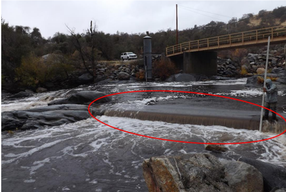
Figure C-3. Image across width of stream at entire project barrier at Kaweah No. 2 Diversion Dam Gage Pool Weir. Circled portion identifies location of measurements.
