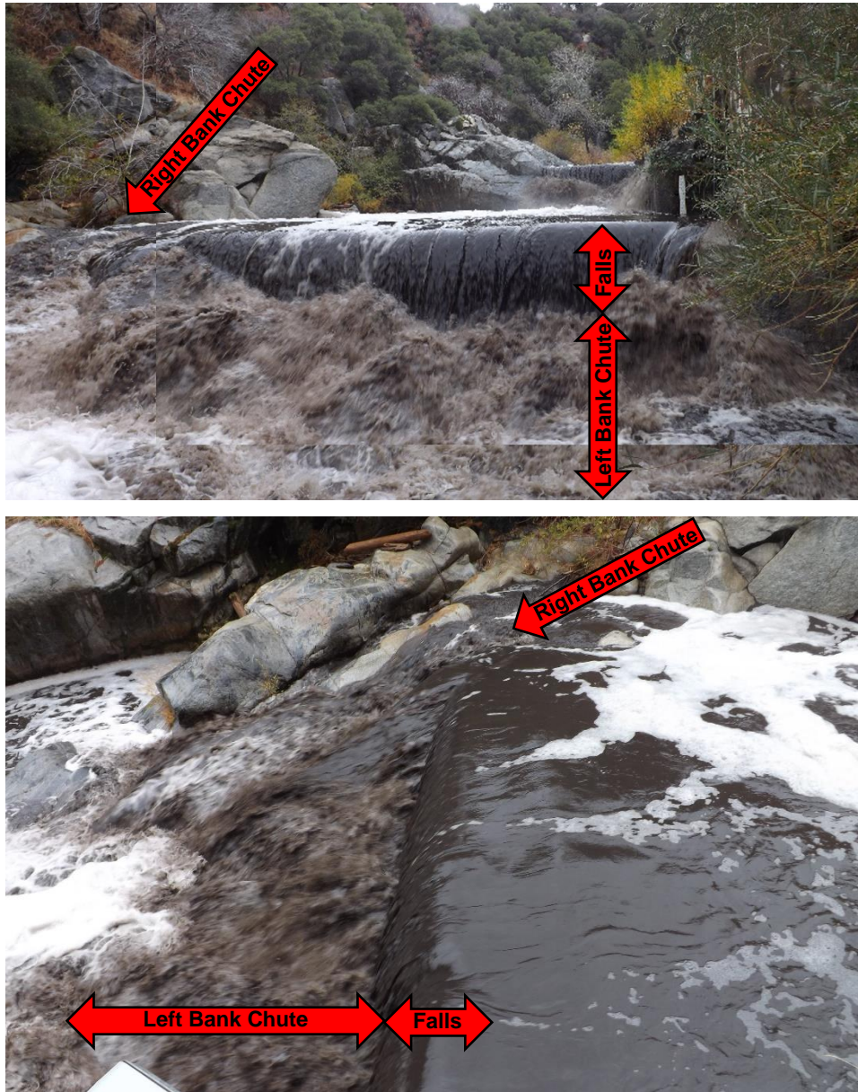
Figure C-6. TOP: Image of project barrier at Kaweah No. 1 Diversion Dam Gage Pool Weir. Kaweah No. 1 Diversion Dam project barrier is visible in background. BOTTOM: Image across width of project barrier at Kaweah No. 1 Diversion Dam Gage Pool Weir towards the right bank.
