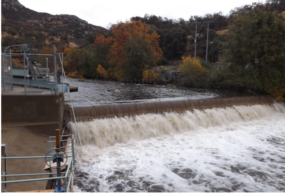
Figure C-2. Image of project barrier at Kaweah No. 2 Diversion Dam. Staff holding stadia rod on left side of image for scale.
