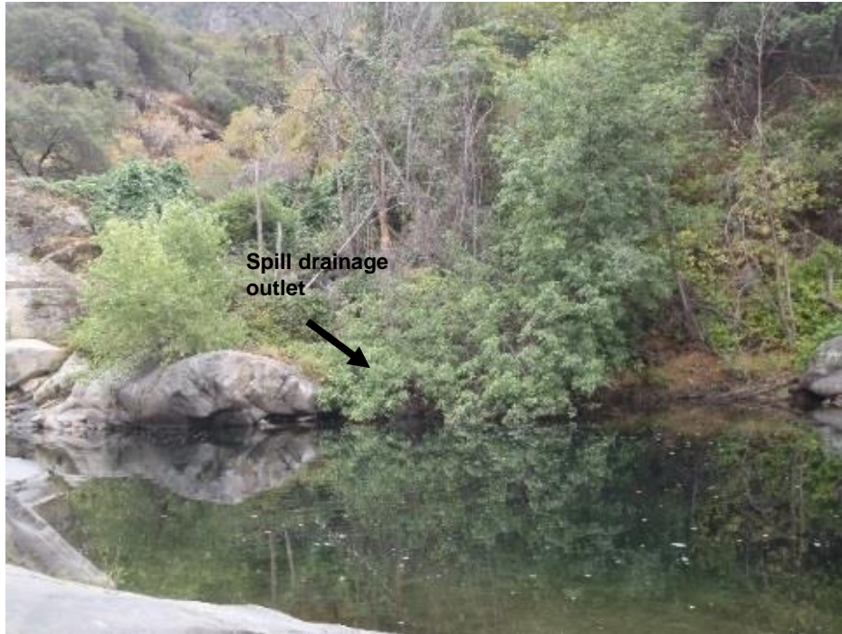
Figure AQ 5-7e. Outlet of the natural drainage channel that receives flow from the Kaweah No. 3 Forebay at the Kaweah River.
