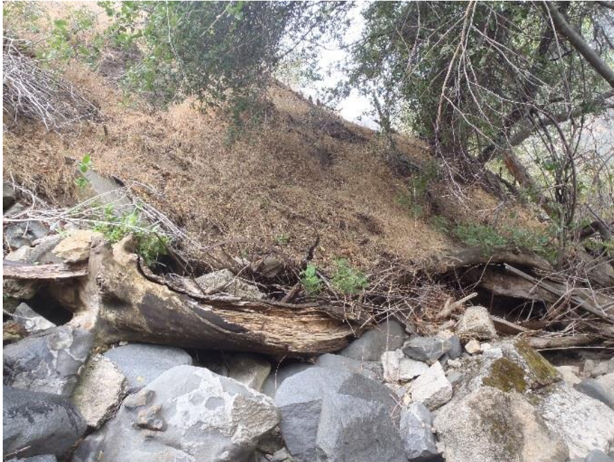
Figure AQ 5-7c. Representative section of the natural drainage channel that receives flow from the Kaweah No. 3 Forebay showing boulders along the side slopes of the drainage.
