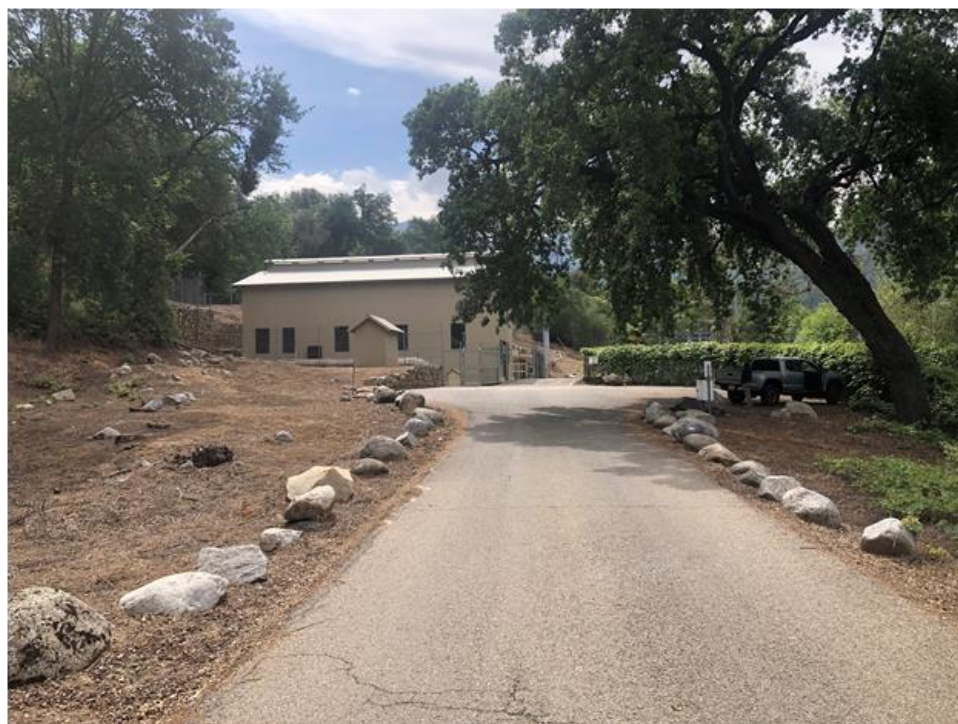
Photo A-11. Kaweah No. 2 Powerhouse as seen driving east on Kaweah River Drive. May 16, 2019.
