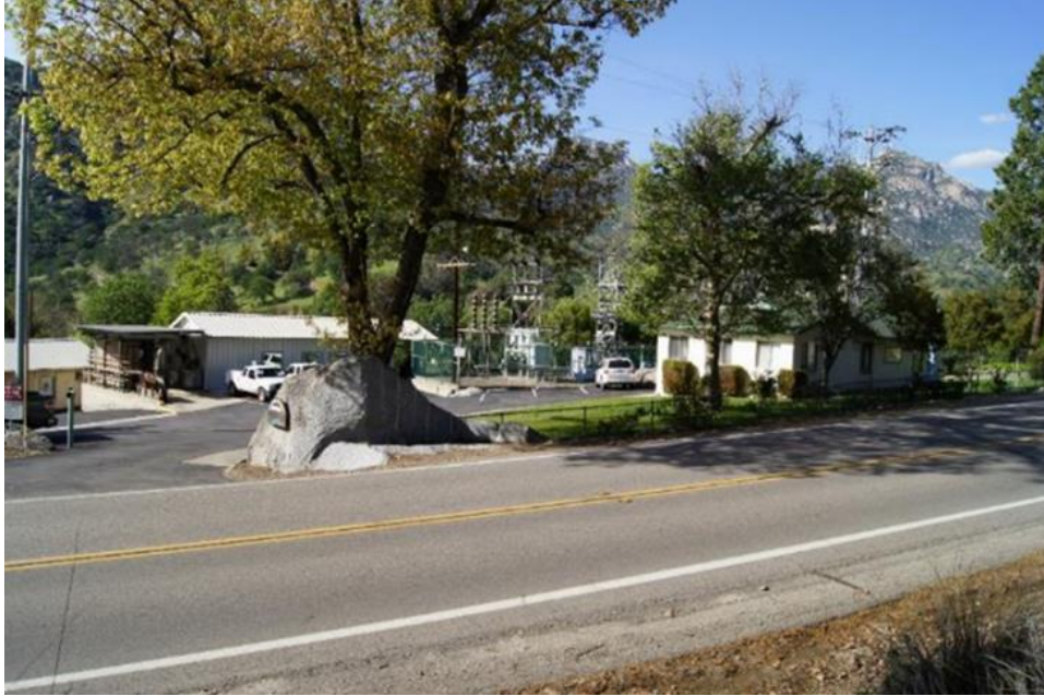
Photo A-6. Kaweah No. 1 Powerhouse Campus as seen travelling east on Highway 198. Camera facing northeast. April 18, 2018.
