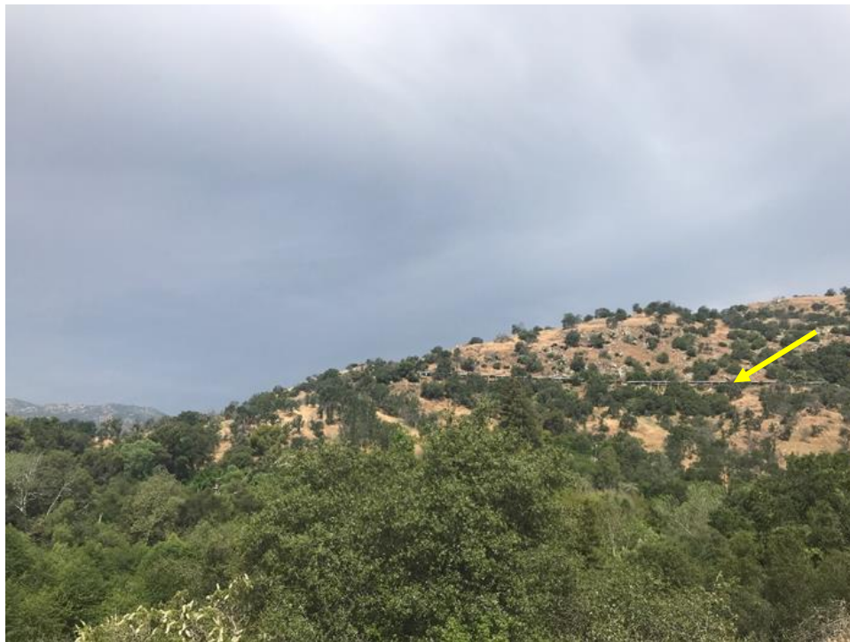
Photo A-9. Kaweah No. 2 Flowline as seen from Highway 198. Camera facing northwest. May 16, 2019.
