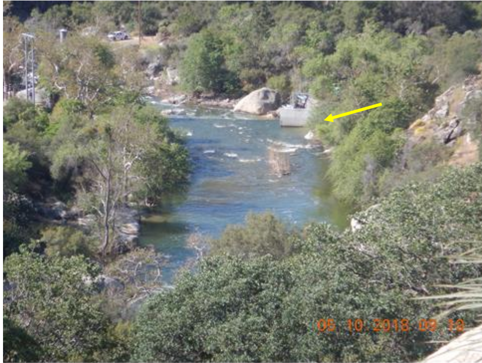
Photo A-8. Kaweah No. 2 Diversion Dam and intake structure on the Kaweah River as seen from the Indian Head Trailhead Parking Area. Camera facing southwest. May 10, 2018.
