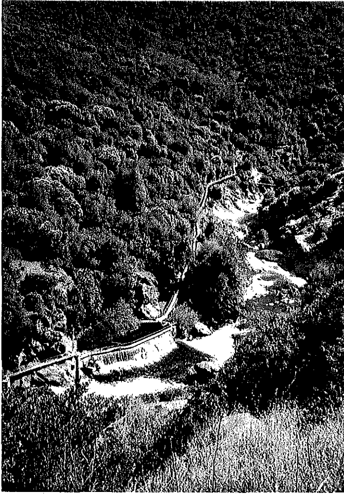
2A - East Fork Intake and Flume
