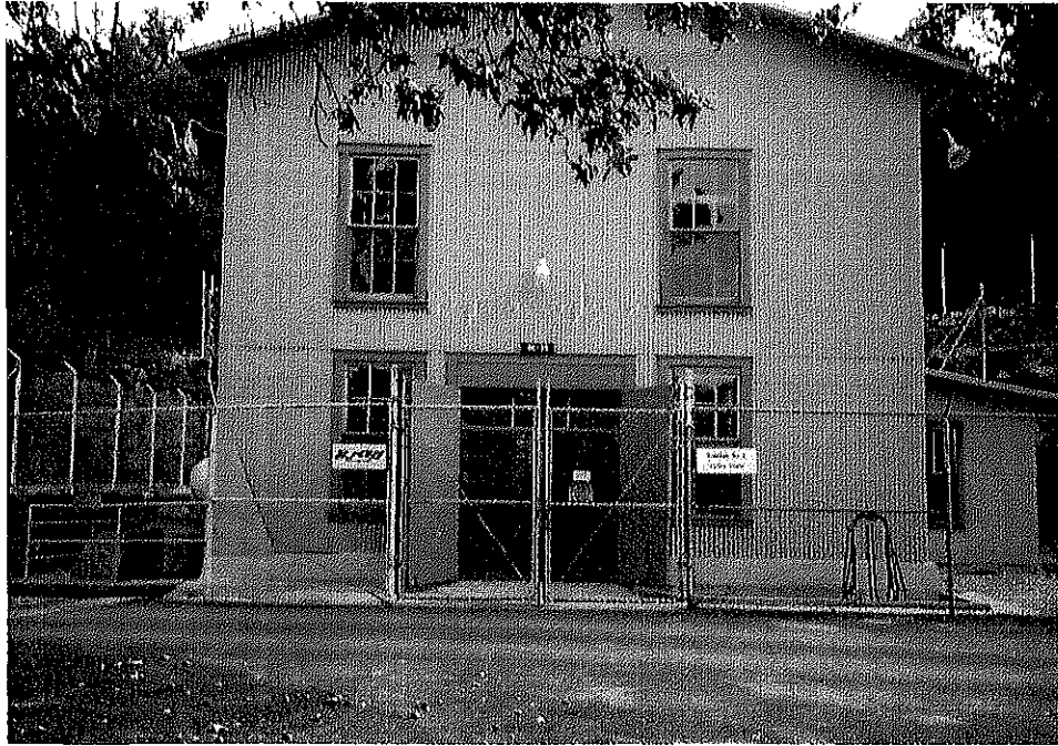
3C - Kaweah No. 2 Powerhouse
