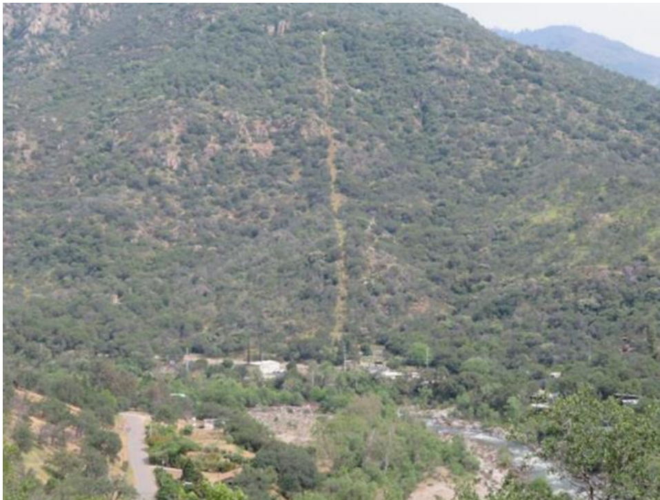
Photo A-5. Kaweah No. 1 forebay, penstock alignment and powerhouse as viewed from Dinely Road. The Kaweah River is in the foreground. Camera facing southeast. May 8, 2018.
