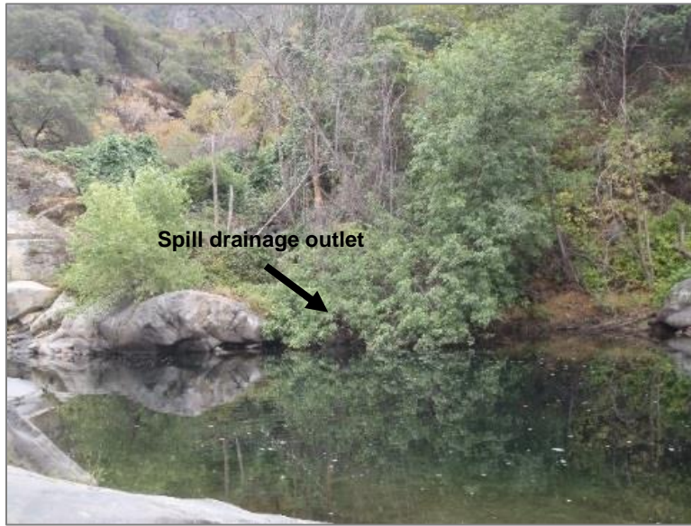
(e) Outlet of the Kaweah No. 3 natural drainage channel at the Kaweah River.
