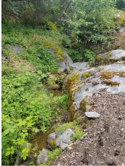
(a) Representative photograph of the portion of the Kaweah No. 1 natural drainage channel upstream of the Kaweah No. 1 Powerhouse
