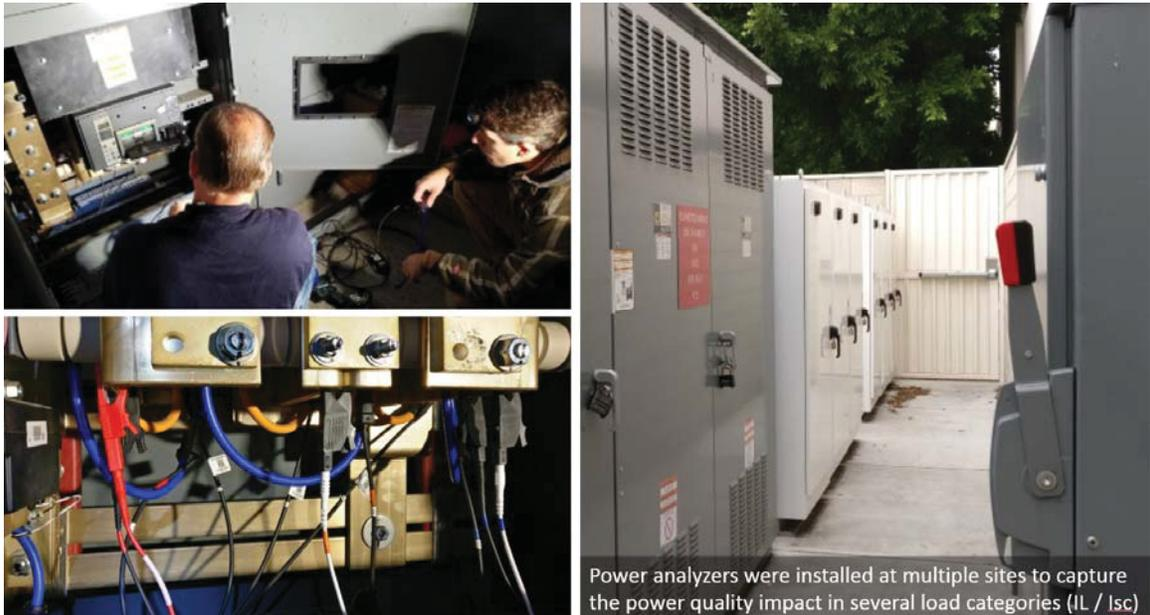
**Figure 3 - Power Analyzer installation**
