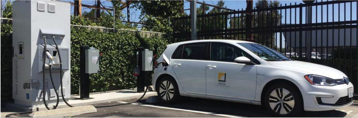
**Figure 12 - Efacec DC fast charger installed at SCE's Electric Vehicle Technical Center (EVTC) in Pomona**
