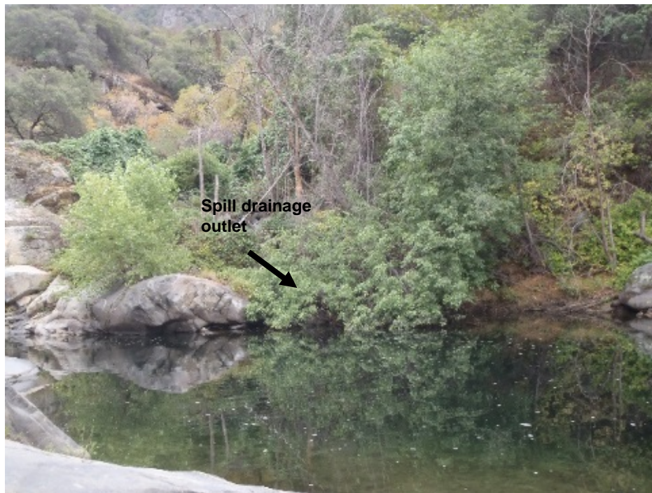
e. Outlet of the Kaweah No. 3 spill drainage at the Kaweah River
