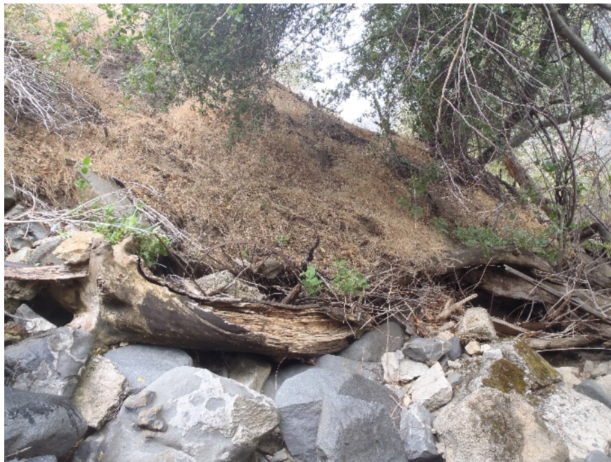
c. Representative section of the Kaweah No. 3 spill drainage showing boulders along the side slopes of the drainage.
