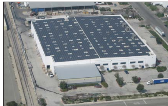
The 800-kilowatt solar energy system recently installed on this Sierra Aluminum Co. manufacturing plant in Fontana, Calif., is expected to generate 1.4 million kWh per year and meet approximately 60% to 70% of the building's total energy requirements.
