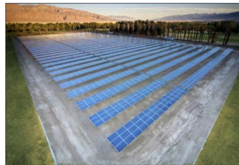
The new 1-megawatt solar photovoltaic system at Furnace Creek Inn & Ranch Resort in Death Valley National Park will generate nearly 2.5 million kilowatt-hours annually and reduce greenhouse gas emissions by 58 million pounds over the next 25 years.
