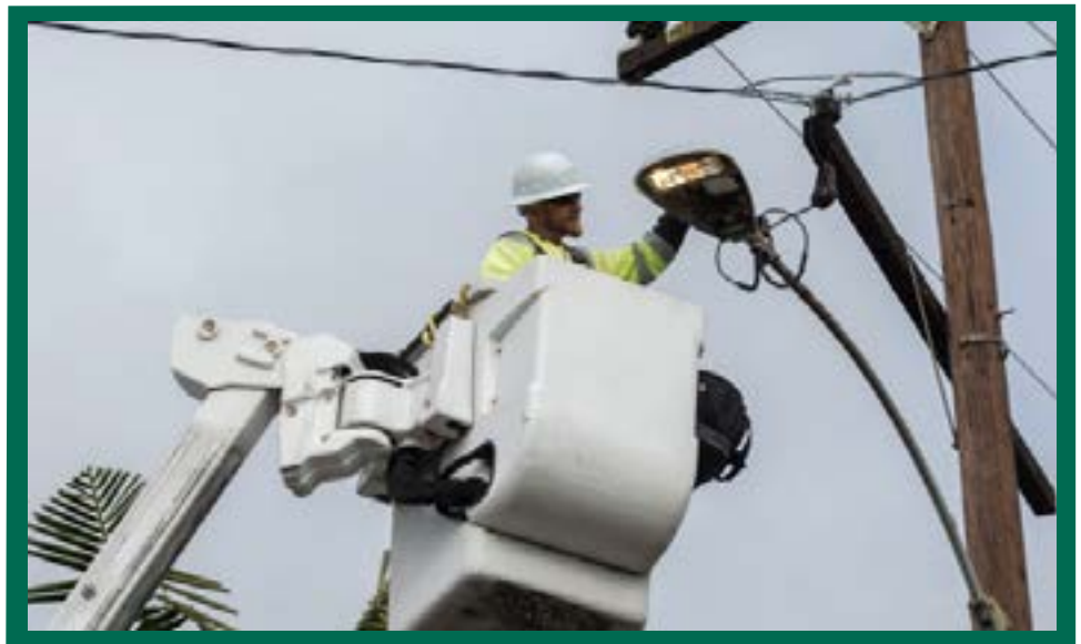
Some cities may save more than $5 million over the life of SCE's streetlight upgrade program, which allows government agencies to request replacement of older, less-efficient bulbs with new LED fixtures. Photo credit: Maria Hedrick
