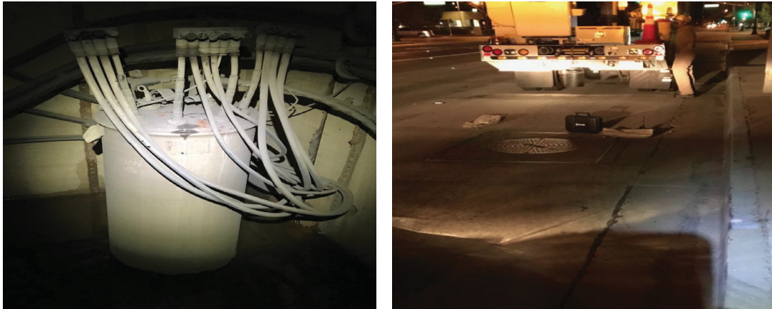
Figure II-4 – BURD Transformer (left) installed in an SCE underground structure (right)
