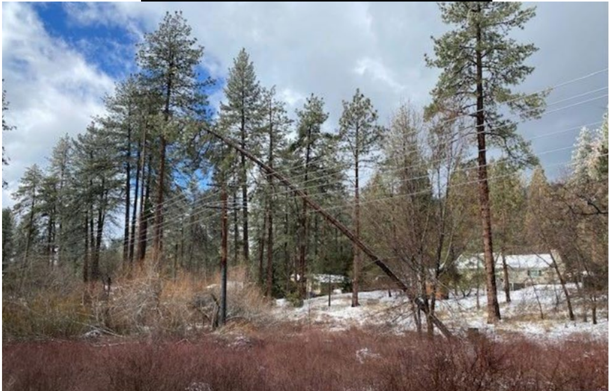
Figure I – Tree fell into lines (Covered Conductor)
