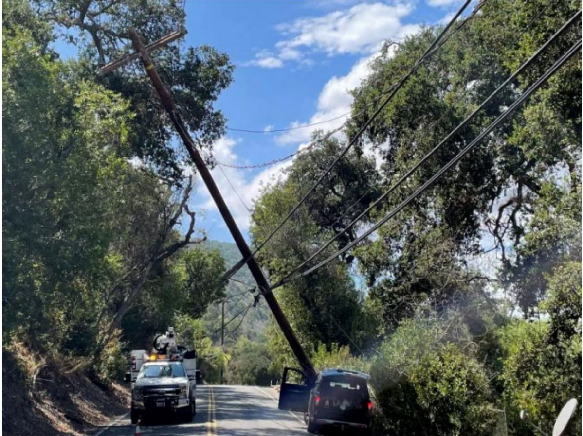
Figure II – Down wire with car hit pole event (Covered Conductor)
