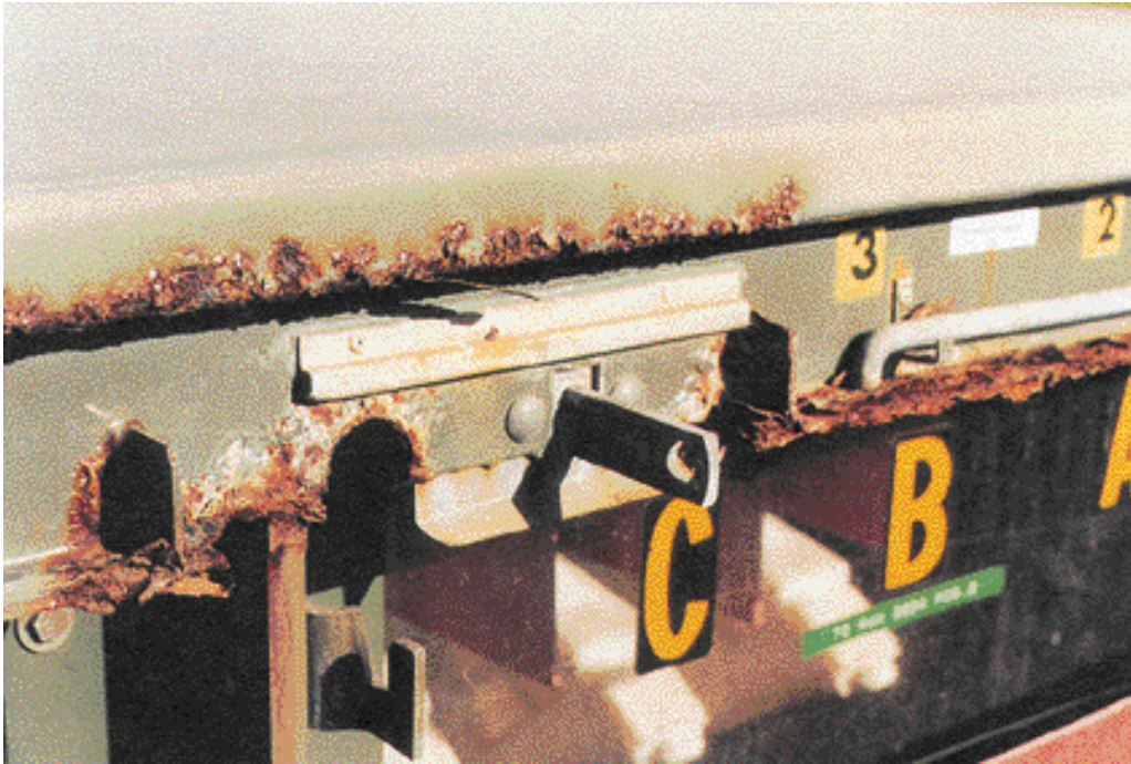
Figure 6–8: Metal Flaking Away at Nonhazardous Locations
