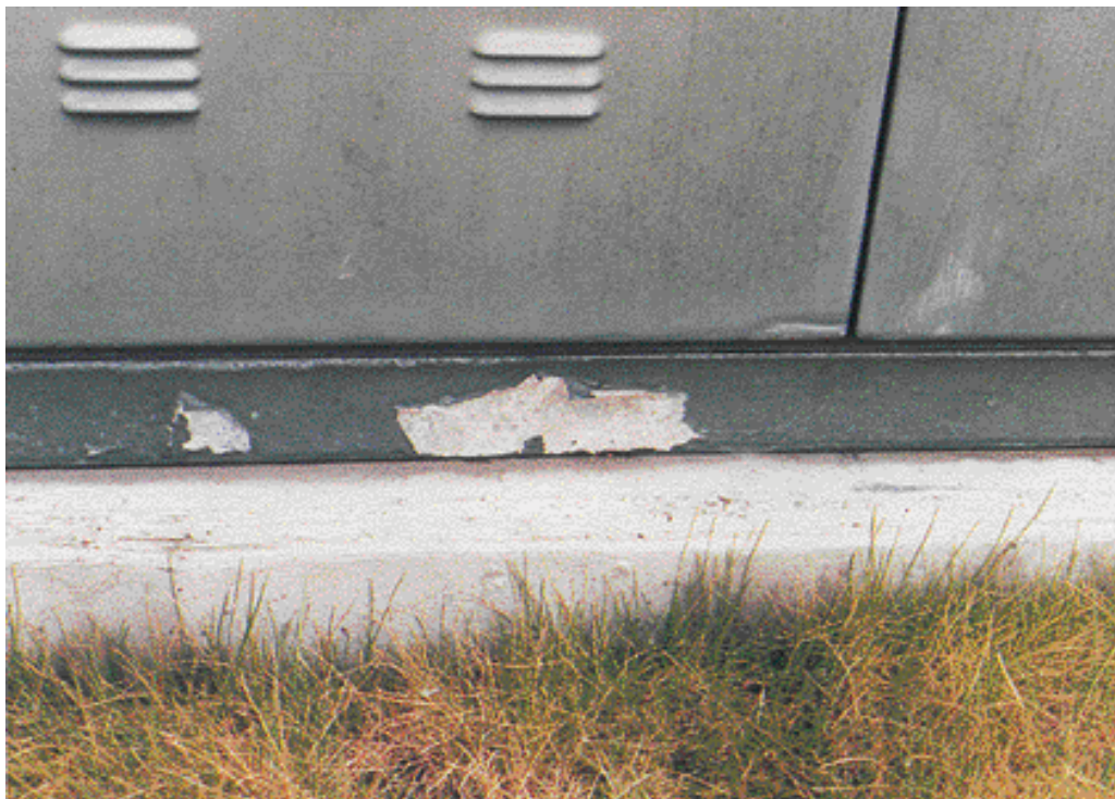
Figure 6–26: Limited Peeling of Paint
