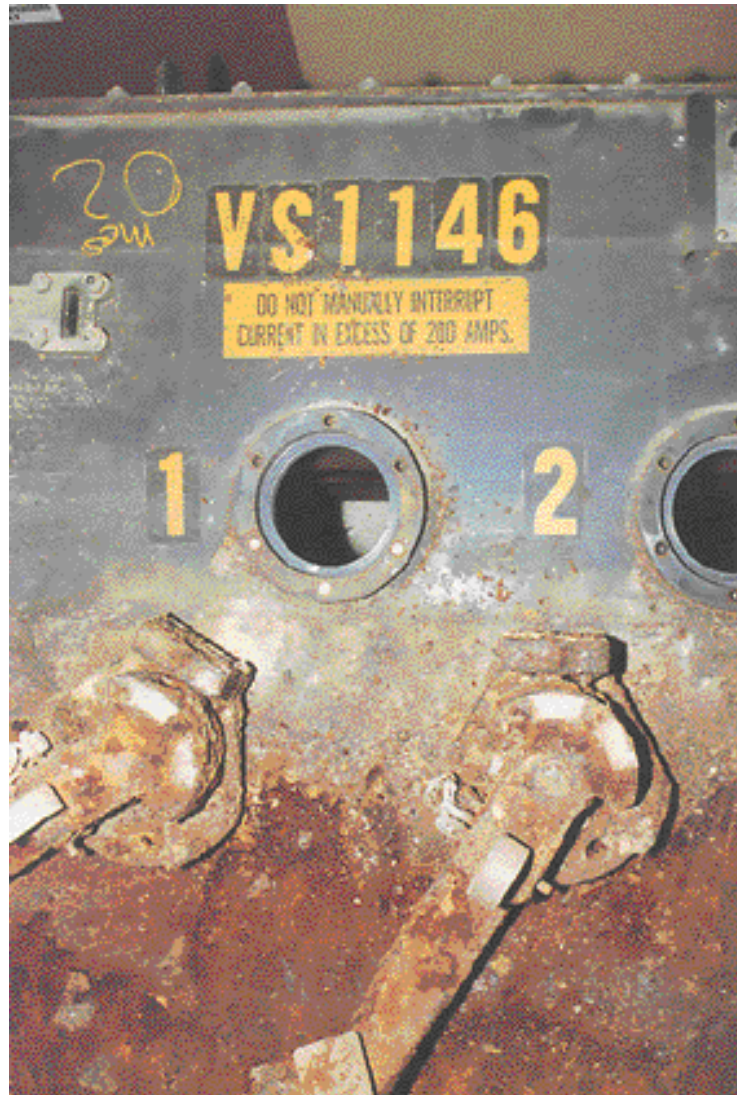
Figure 5–7: Moderate Corrosion — Example 1 of 3
