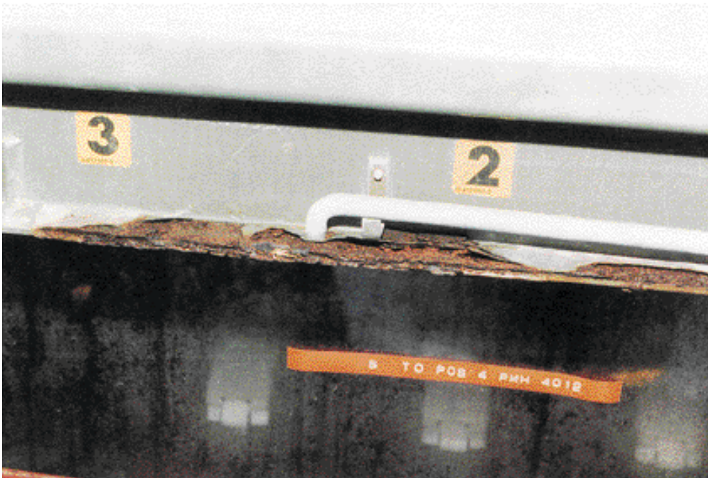
Figure 6–15: Loss of Metal
