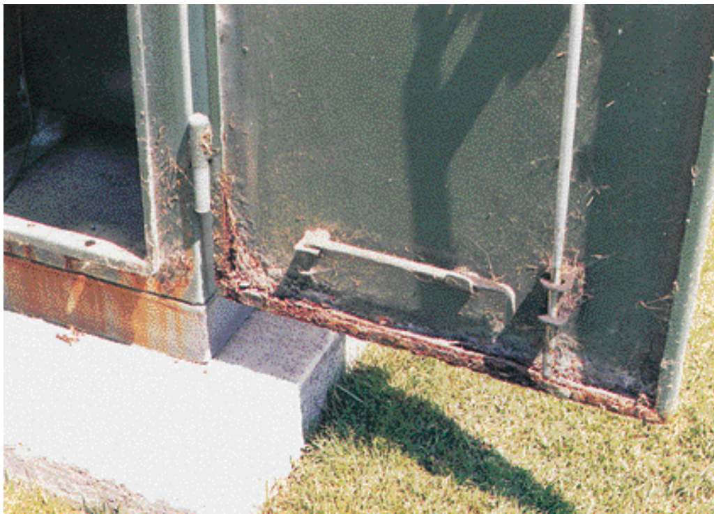
Figure 6–19: Interior Blistering, Flaking, Corrosion, and Discoloration
