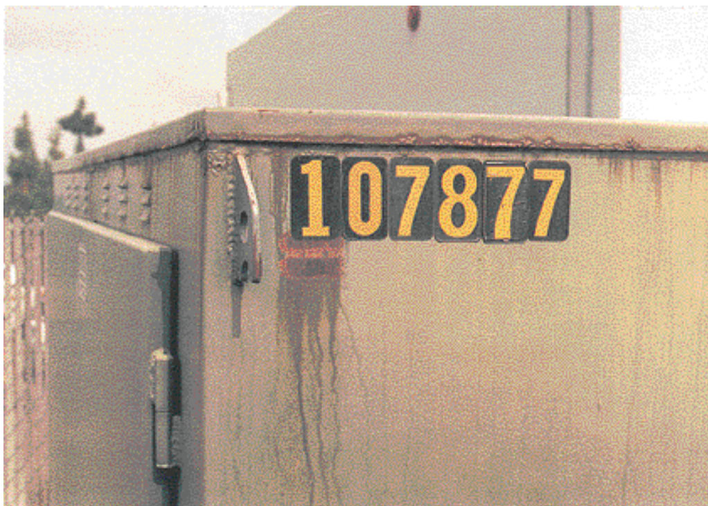
Figure 6–28: Light Corrosion at Lower Edge of Top Cover and Brackets (No Serious Pitting)
