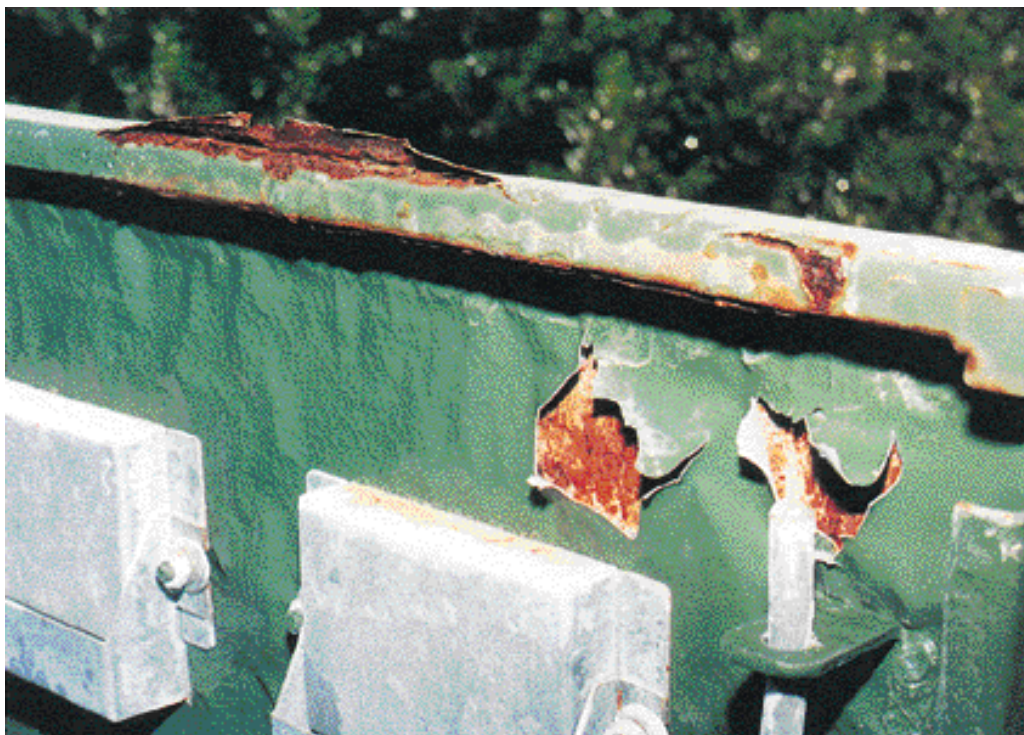
Figure 6–20: Peeling of Paint with Moderate Pitting
