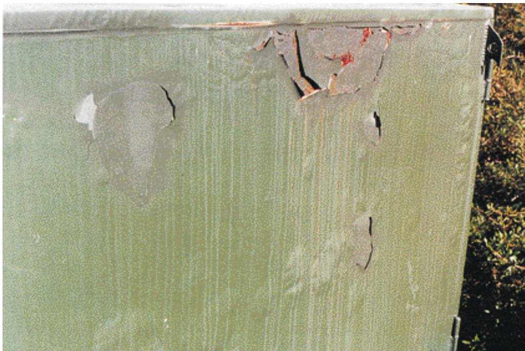
Figure 6–12: Ineffective Prior Repairs
