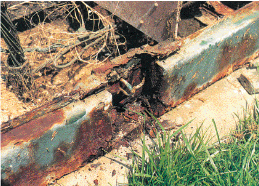
Figure 6–2: Very Heavy Corrosion of Locking Assembly
