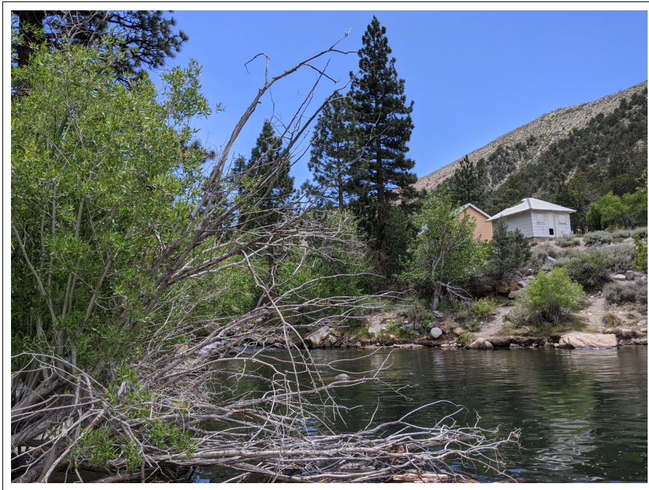
Location of the second recording device at Powerhouse 2.
