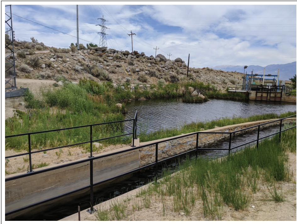
Location of the first recording device at Powerhouse 5.
