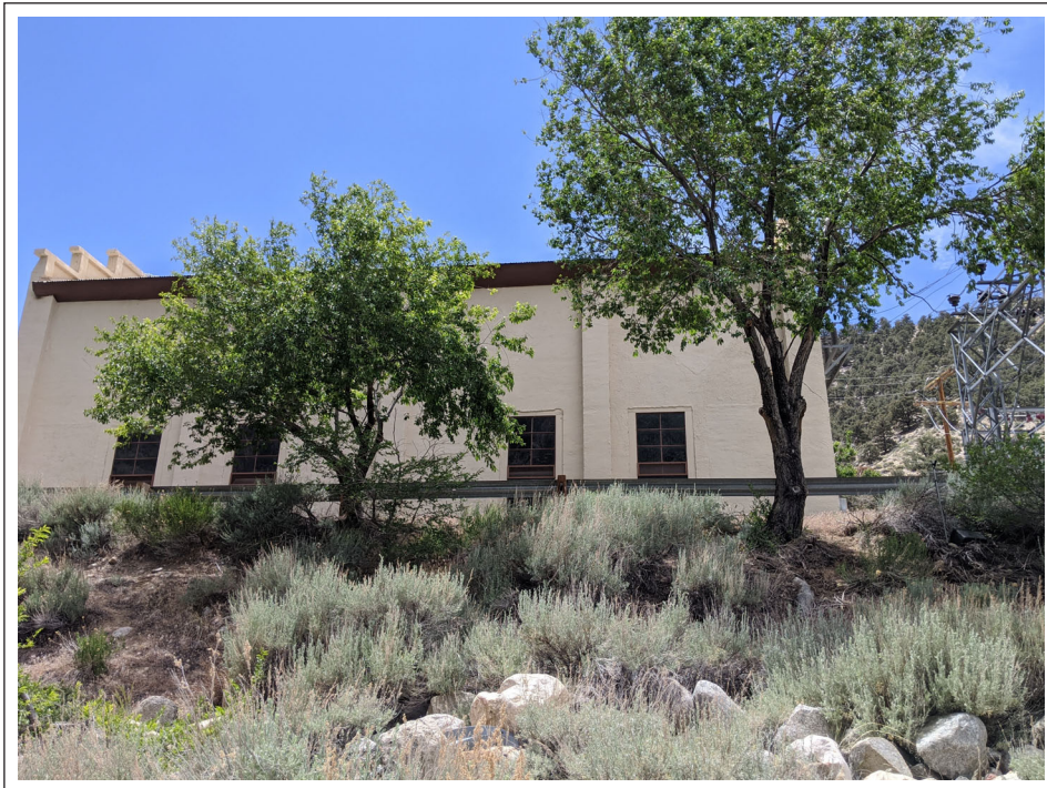
Location of the first recording device at Powerhouse 2.
