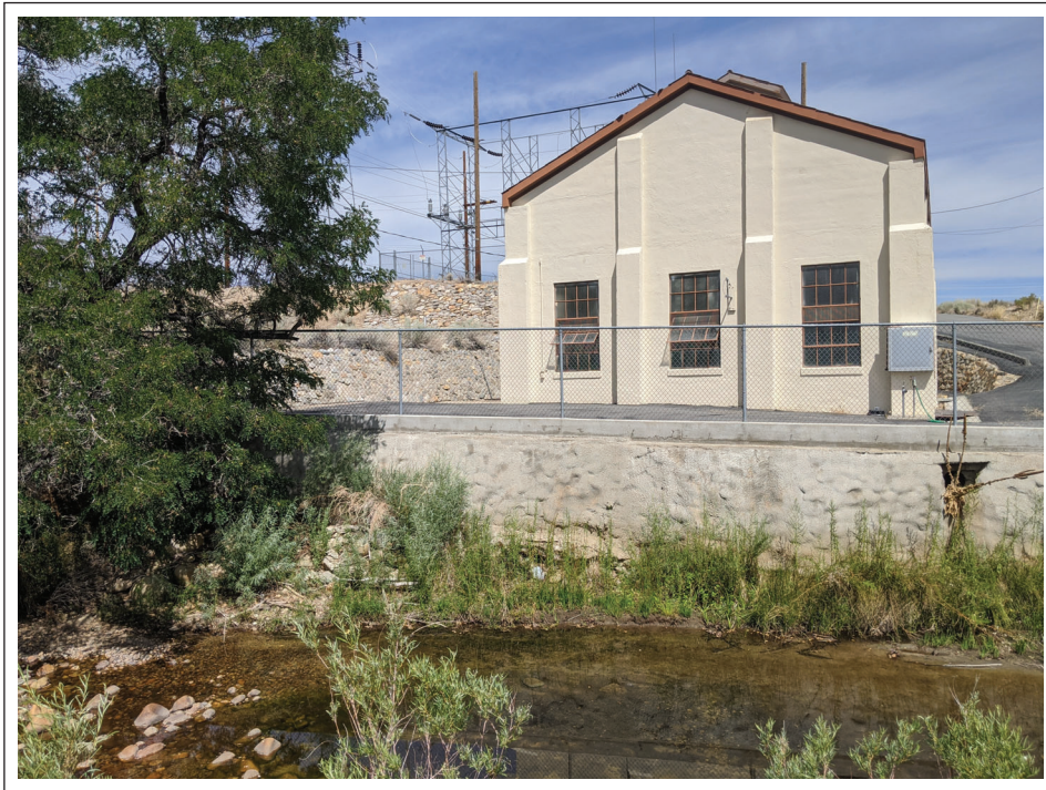
Location of the recording device at Powerhouse 6.
